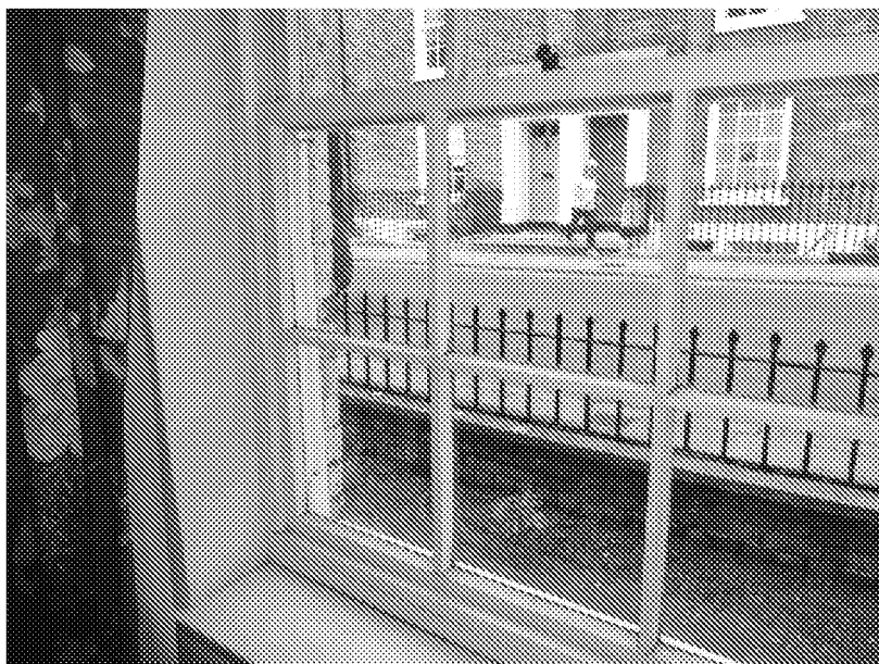
Existing timber sash windows to the front, with thick glazing bars.
