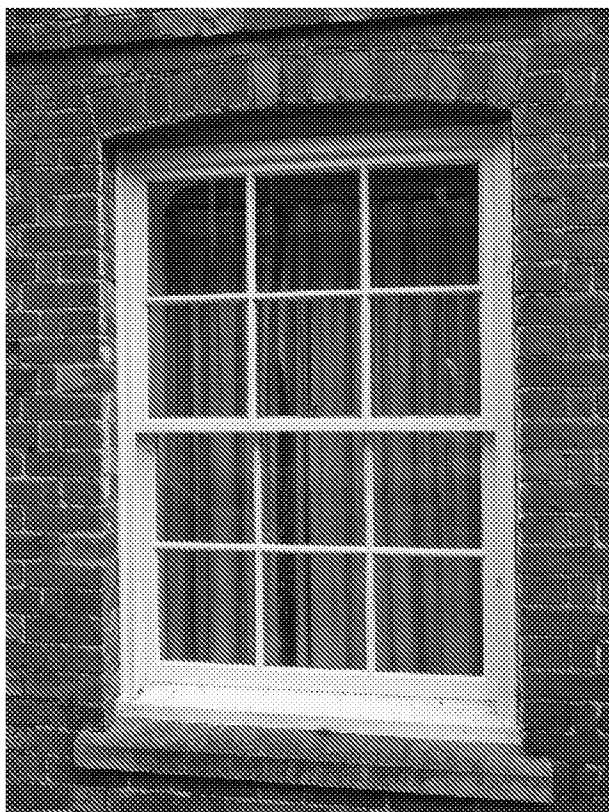
Existing timber sash windows to the front.
