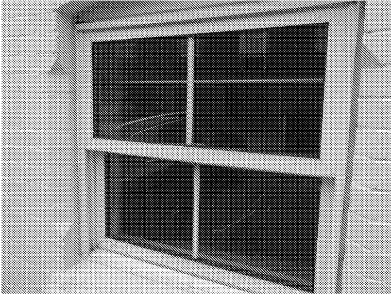
Existing aluminium framed windows to rear.
