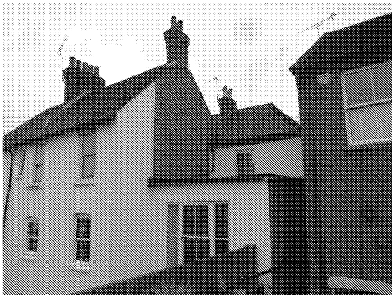
Photo 3 – Rear Elevation, showing flat roof area for potential roof terrace.
