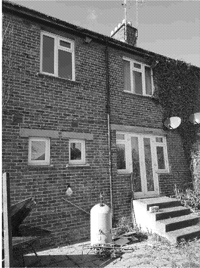
4. View of rear (North East) of property
