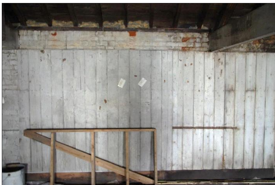
Plate 17: Typical vertical timber wide board panelling along west wall.
