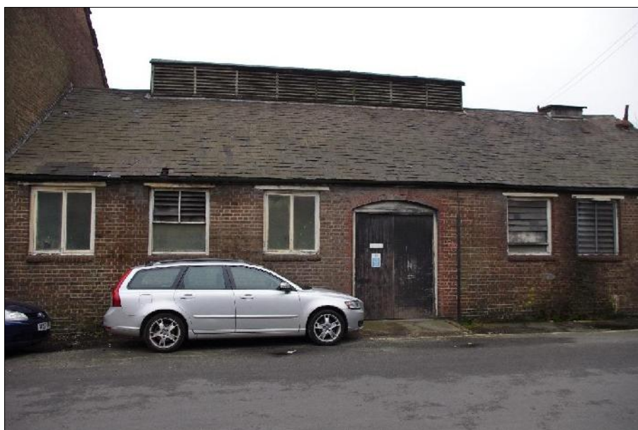
Plate 5: View looking west towards the single-storey range. Windows have either been replaced with modern casements or adapted to include louvers.
