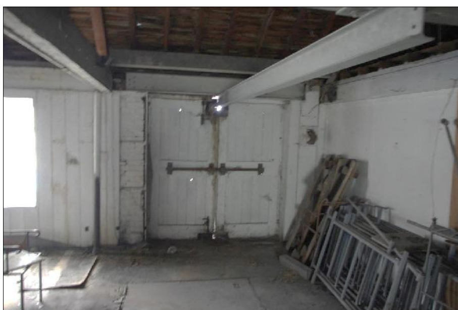
Plate 14: Timber double-leaf loading bay doors on east wall with metal I-beams and a trap door to ground floor.
