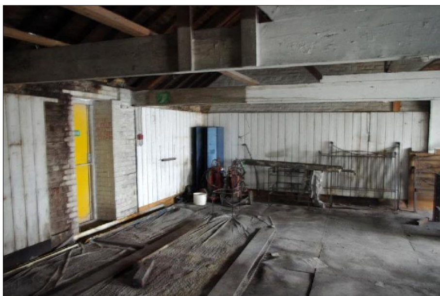
Plate 16: The walls are typically white-painted brickwork with vertical timber wide board panelling along west and north walls.
