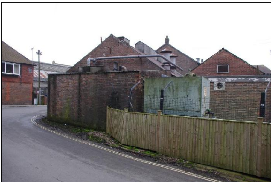
Plate 7: View looking south at the north wall of the single-storey range. Morden plant and pipework is evident on the gable end and west roof pitch.
