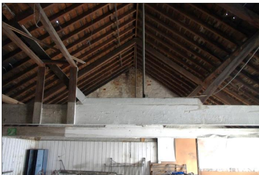
Plate 15: Original timber tie beams and metal king posts, albeit with additional timber framing applied for additional support and likely to house machinery. This is considered a typical roof structure from the late nineteenth century.
