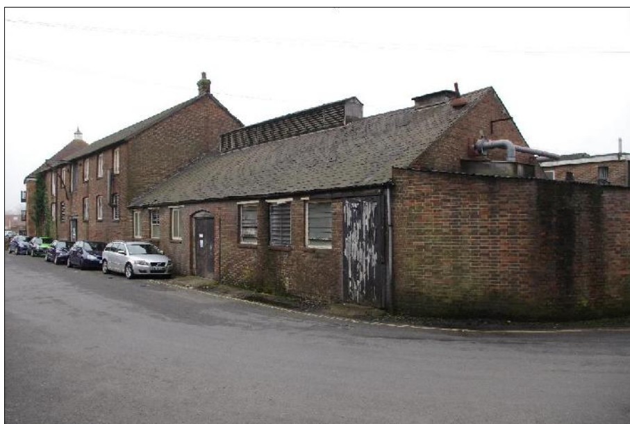
Plate 6: View looking south-west towards the single-storey range with two-storey range beyond.
