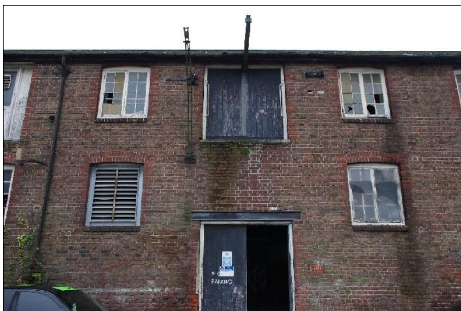
Plate 3: View looking west towards central bay of two-storey range where the main double-leaf door at ground floor and double-leaf loading bay at first floor exist.
