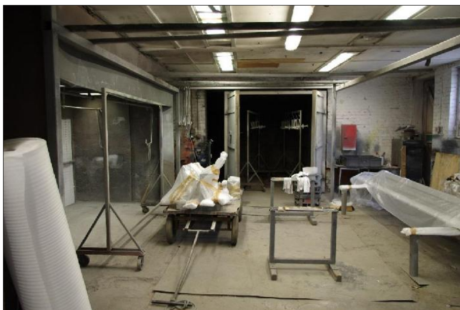
Plate 9: North room in single-storey range with modern false ceiling, partitions, and concrete floor.
