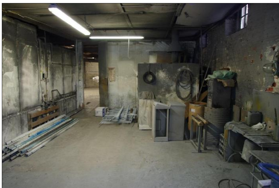
Plate 11: Main ground floor room in two-storey range. Modern false ceiling and partitions have been inserted, breaking up the original plan layout.
