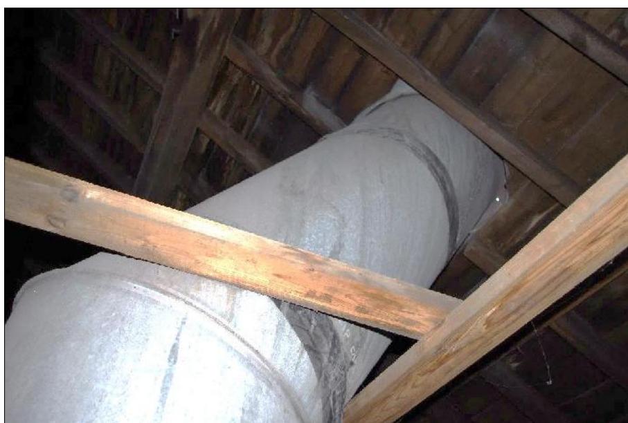
Plate 18: Modern metal flue which has been inserted from ground floor plant room below and out through planked underside of roof.
