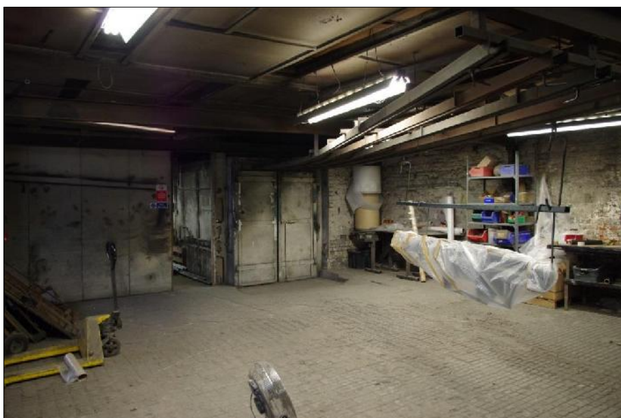
Plate 8: South room in single-storey range with engineering brick floor and false ceiling, and provides access to ground floor of two-storey range through modern sliding door.
