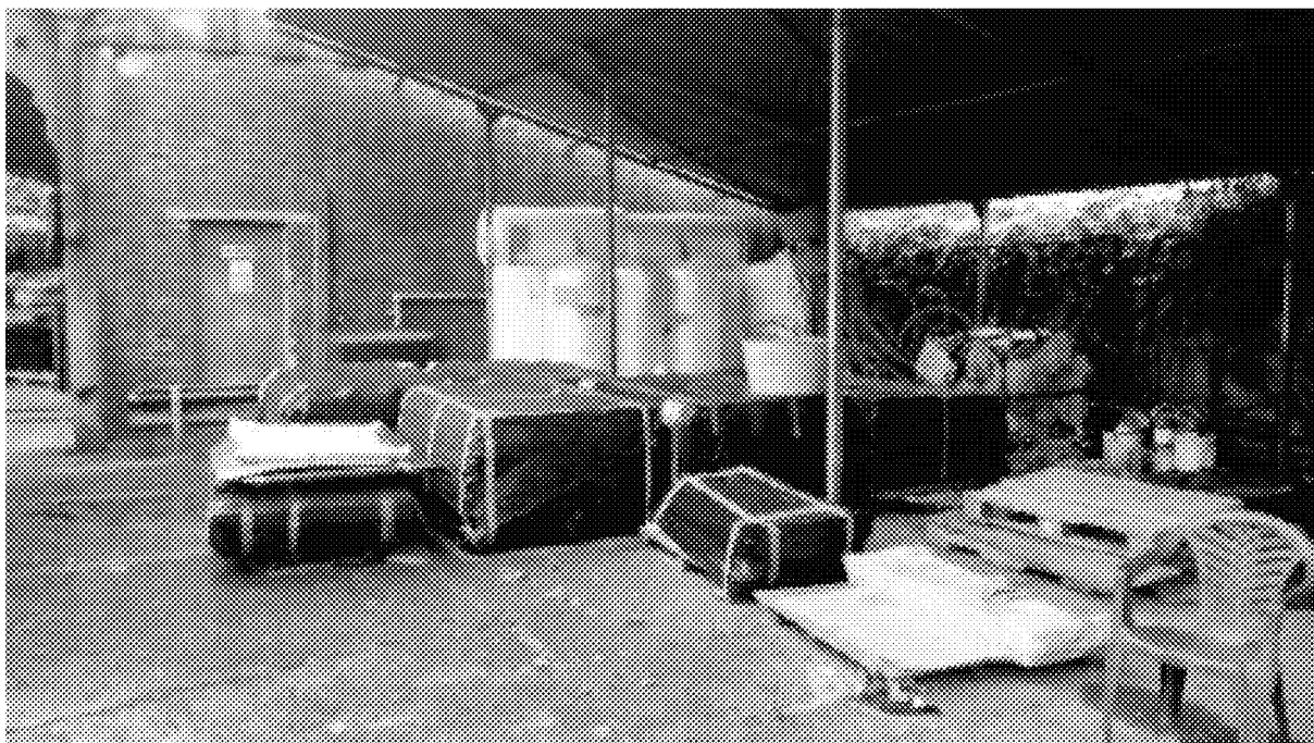
Photograph 2: Storage of products on site.
