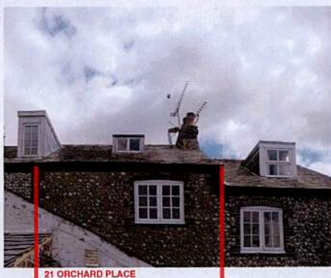
Existing rear condition, showing the current dormer window in relation to the larger neighbouring windows
