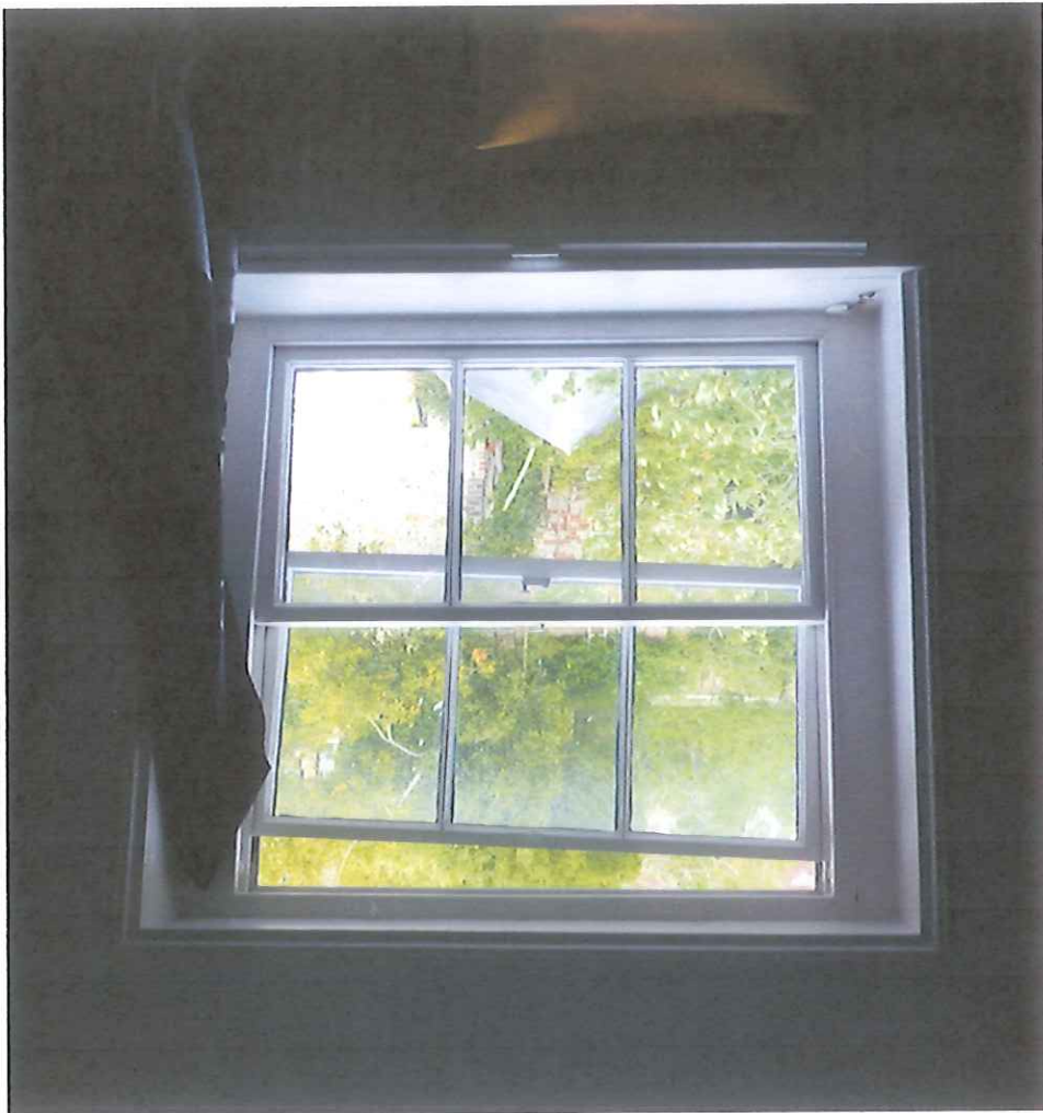
WINDOW W6/REPLACE + DOUBLE GLAZE
