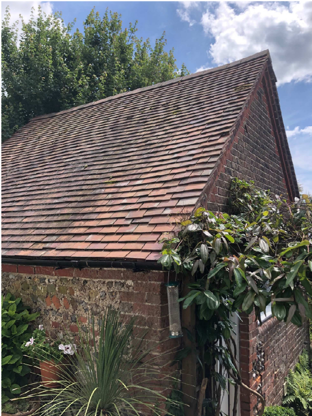
Front north elevation of rear outbuilding
