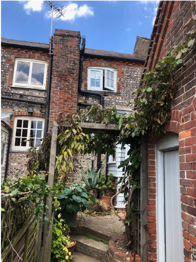
Rear south elevation – 11 Bond Street
