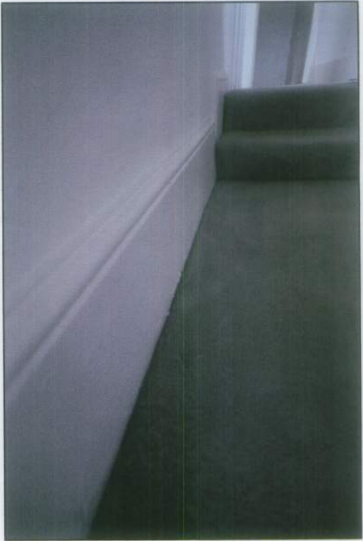
Photo of existing skirting (S2)
