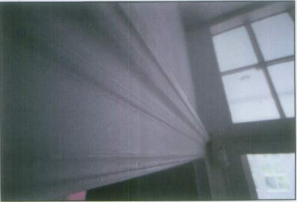
Photo of existing architrave (A2)
