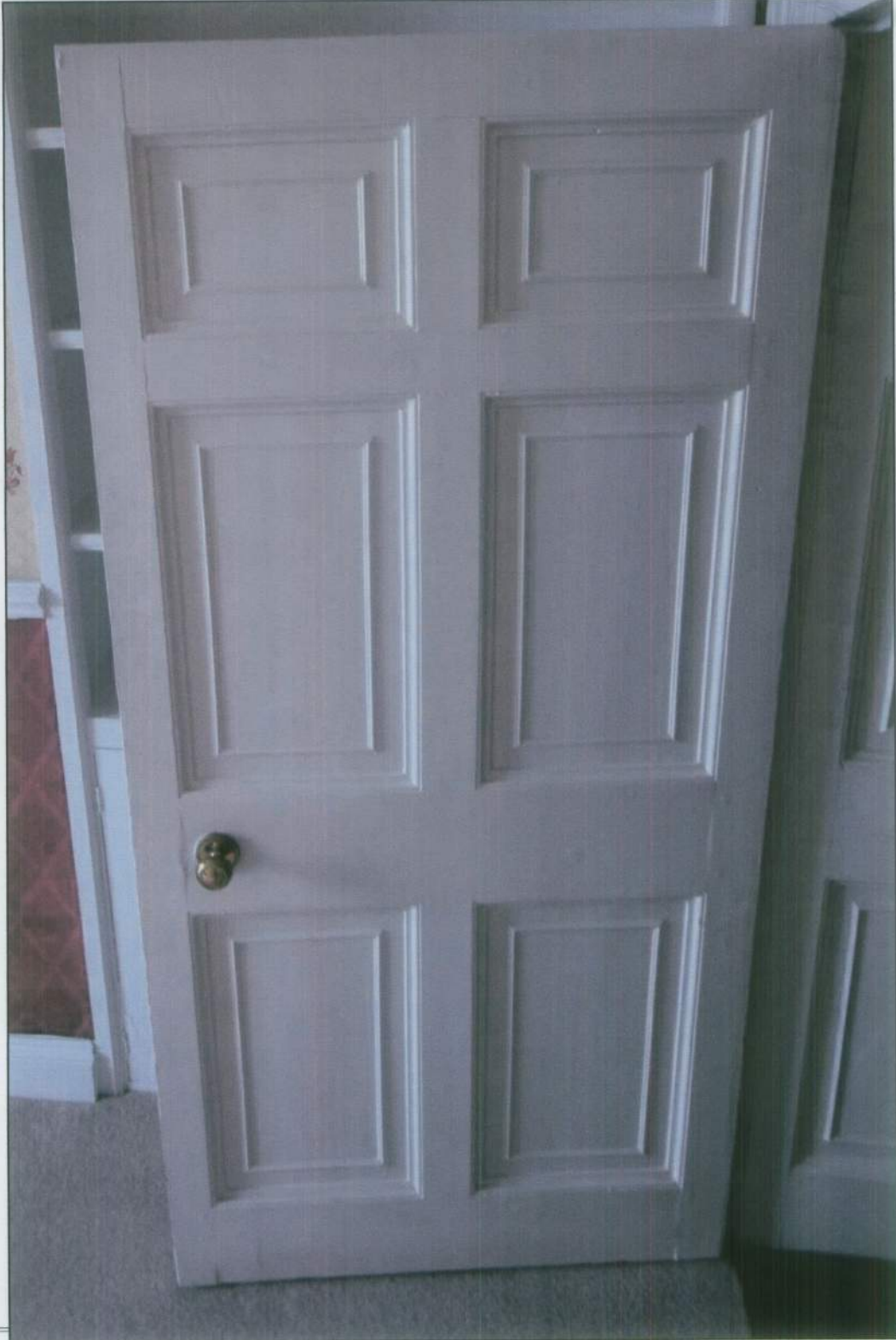
Photo of existing door, Type 2
