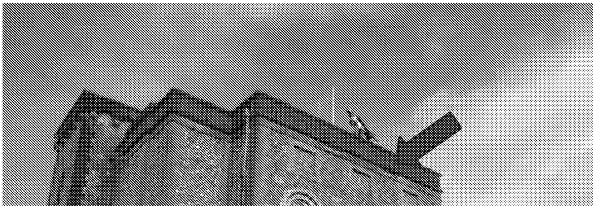
Image – Photo - Arundel Town Hall – Vents at high level through parapets & black anchor plates.
