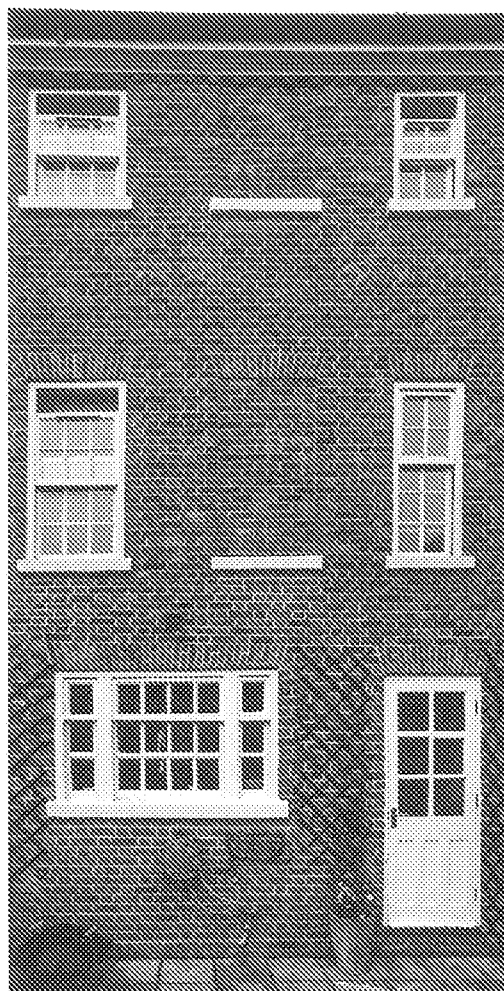
10 Nineveh Shipyard – Current rear
