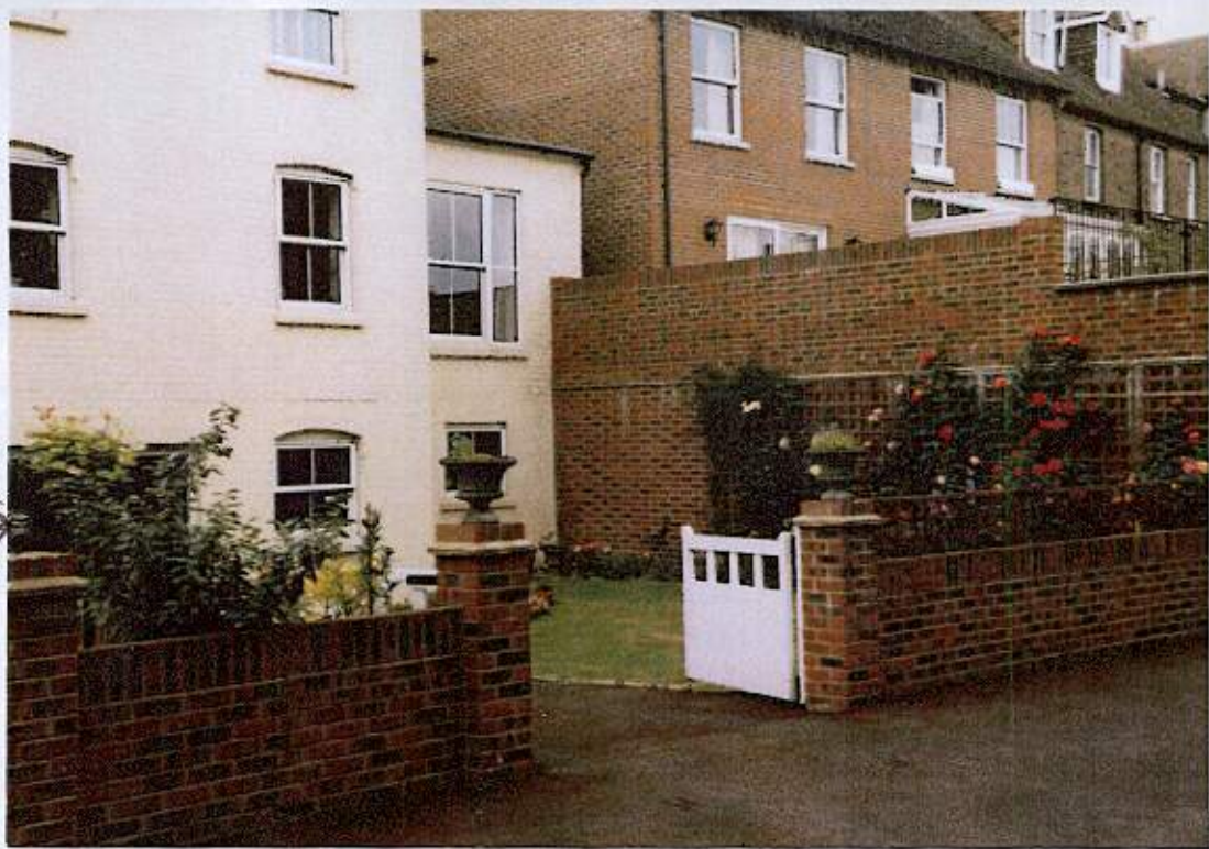
Rear view of No. 83 TARRANT ST. FROM GARAGE MEWS OF TARRANT WHARF
