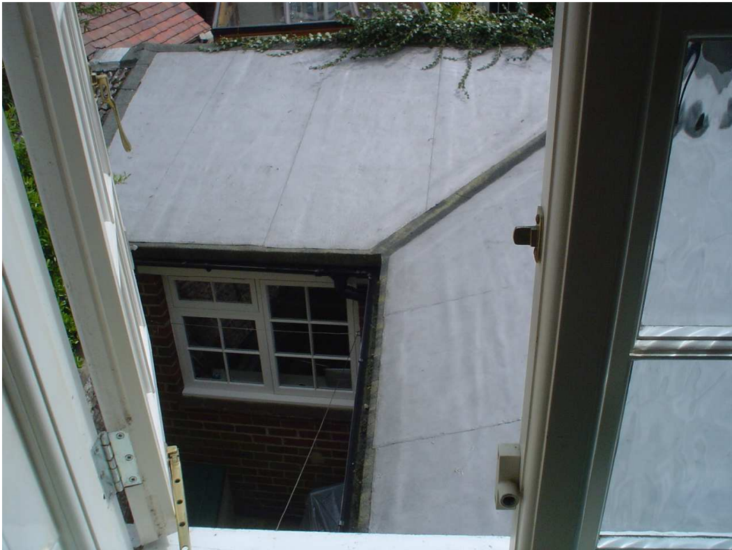
VIEW OF EXISTING SINGLE STOREY BUILDING LOOKING EAST
