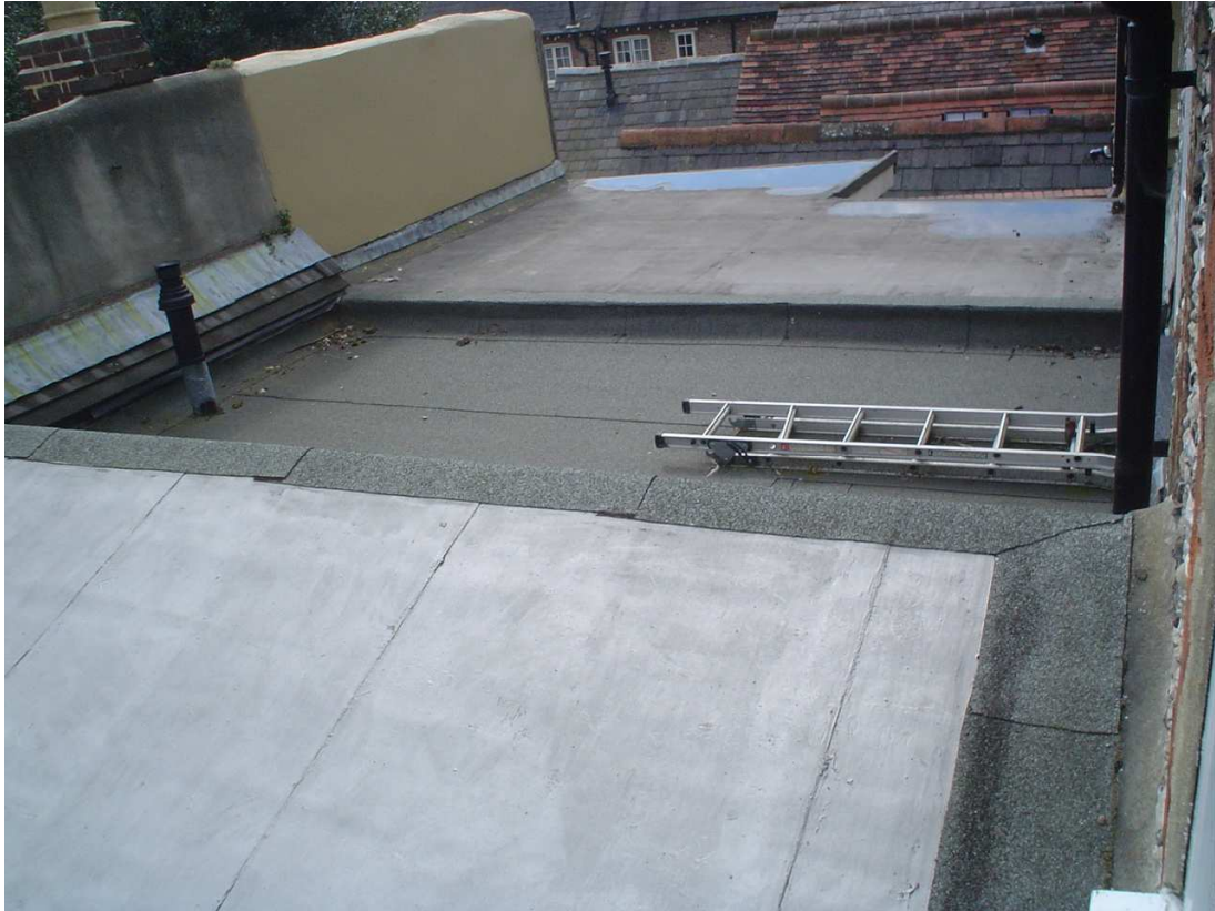
ADJOINING FLAT ROOFED BUILDINGS TO THE SOUTH
