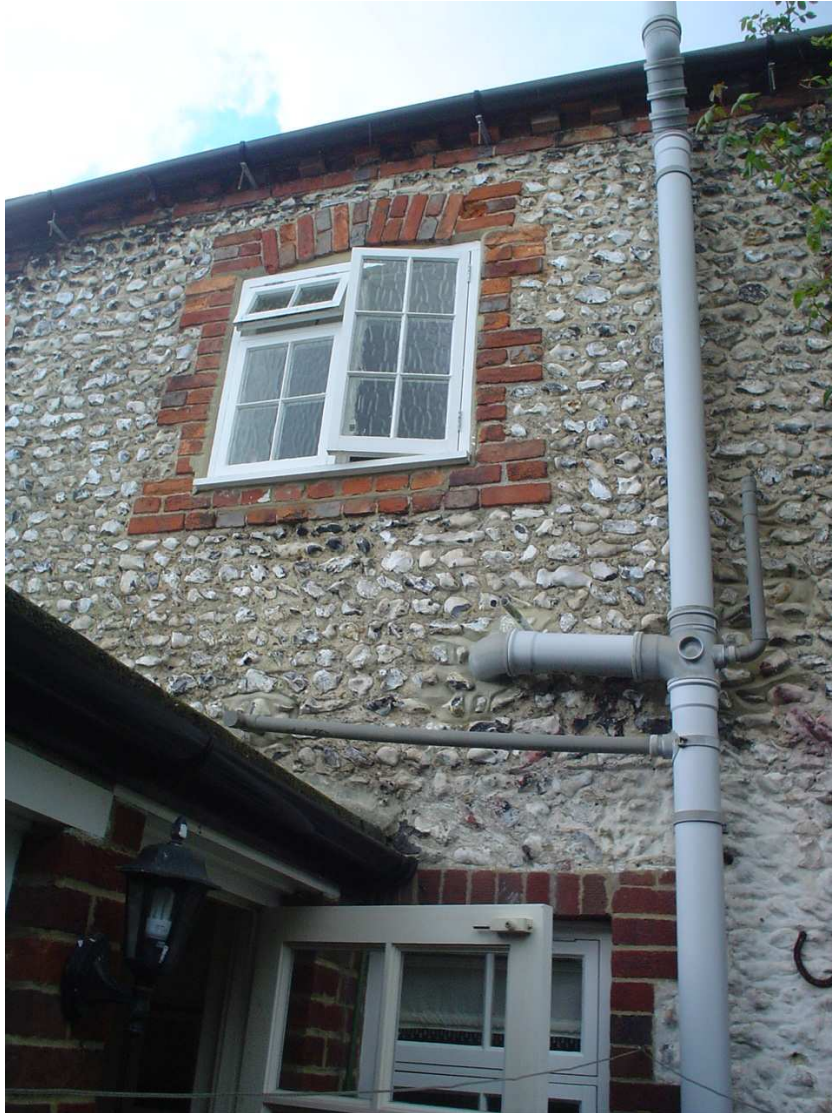
REAR ELEVATION OF MAIN HOUSE
