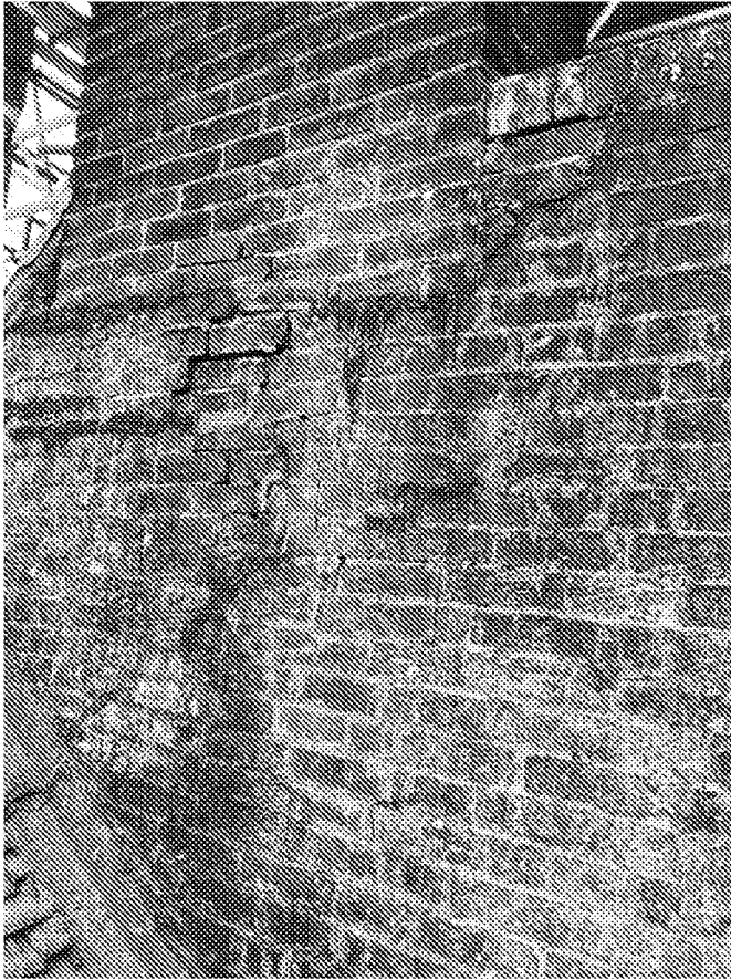
Fig. 1, Base of existing chimney.
