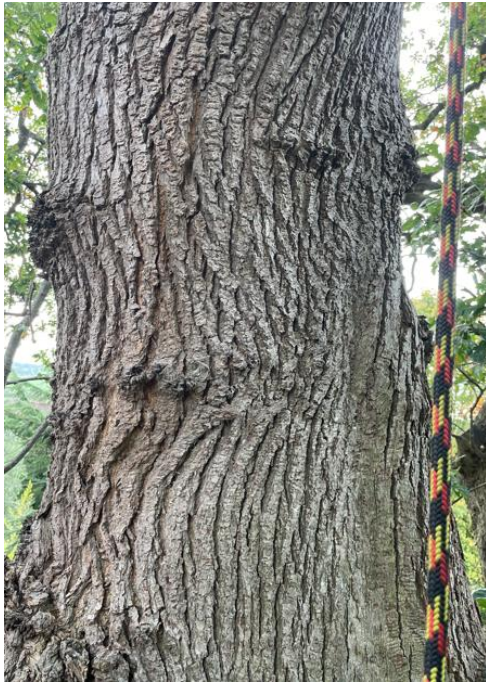
Photo 3. The opposite side of the stem, relative to the branch wound and decay. Shown from the north and exhibits no signs of decay.
