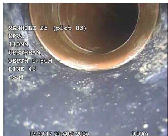
SVPX_2a61e4e4-b748-43a6-859b-07c19e03c5cd_20260917_184618_523.jpg, 00:00:30, 0.02 m Line deviates right
