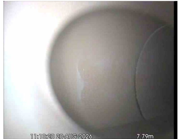
MH19X_87352554-c3a2-4c3d-886e-ea60928cbe1a_20260917_173707_311.jpg, 00:01:21, 7.79 m Finish node, major connection without manhole, reference: BLIND JUNCTION - JOINS THE MAIN SEWER, **IN THE ROAD**
