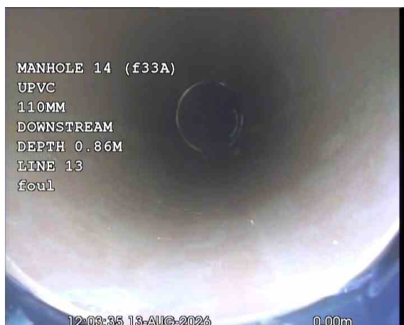
MH14 (F33AX_c128a3d8-e5f8-48ef-931e-8feba2648af1_20260917_165344_759.jpg, 00:00:34, 0.00 m Start node, manhole, reference: MANHOLE 14 (MH14), (F33A)
