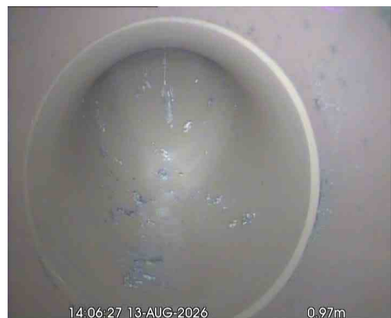
SVPX_e743adae-db1d-4e84-8163-44e73515b26a_20260917_170529_959.jpg, 00:00:38, 0.97 m Line deviates up, REST BEND
