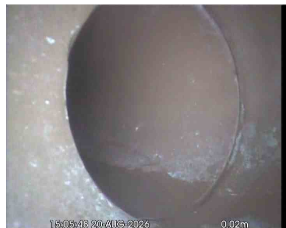
SVPX_ddfad58a-0b6c-4283-a492-8677f958758b_20260918_092316_775.jpg, 00:00:21, 0.02 m Line deviates left
