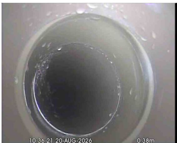
SVPX_fdd0e0d6-8e91-4ef3-b778-3b0a6ac22db0_20260917_172300_699.jpg, 00:00:29, 0.38 m Line deviates left
