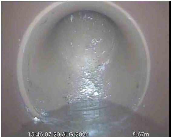
UTIL. SINKX_1084a421-f083-4ae1-b810-c7a12b0fe103_20260918_093430_630.jpg, 00:01:37, 8.67 m Water level, 5% of the vertical dimension
