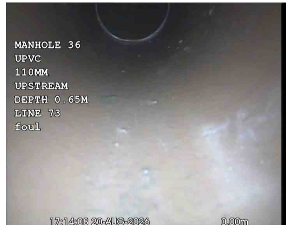
CAPPED OFFX_e6c949f3-364b-4e0d-9c79-17786187e698_20260918_101643_361.jpg, 00:00:11, 0.00 m Water level, 0% of the vertical dimension
