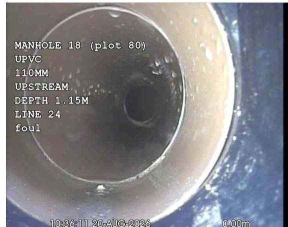
SVPX_c651a3df-8f10-4d18-9e79-4cfe3e3c62d9_20260917_172240_669.jpg, 00:00:19, 0.00 m Water level, 0% of the vertical dimension
