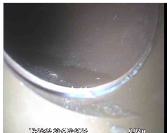
SVPX_b7ab71b3-2d14-44ea-9f15-2c95f3af226f_20260918_102254_485.jpg, 00:00:27, 0.02 m Line deviates left
