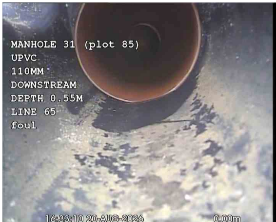
MH31X_7acb1600-036b-4443-83cc-c4d7daa298e3_20260918_094652_704.jpg, 00:00:13, 0.00 m Start node, manhole, reference: MANHOLE 31 (MH31)
