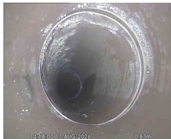
BASINX_4352884e-0c3c-48e3-b304-1235cdef5f5c_20260917_170904_555.jpg, 00:00:40, 0.83 m Line deviates left
