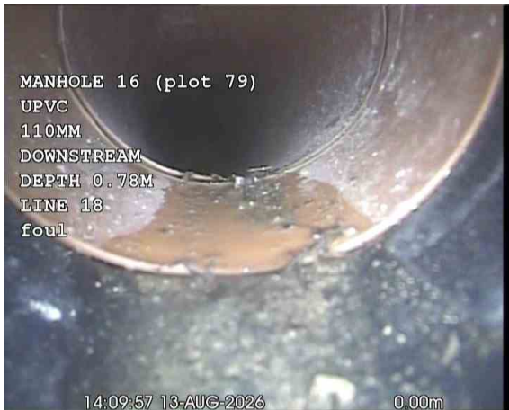
MH16X_7ed15a63-7253-4d54-bc25-7c3c44105ce0_20260917_170643_154.jpg, 00:00:22, 0.00 m Start node, manhole, reference: MANHOLE 16 (MH16)
