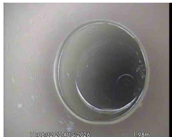
W_CX_bf7f41d6-6092-4f26-b0fa-a86bc298efb0_20260917_173307_462.jpg, 00:00:28, 1.98 m Line deviates right
