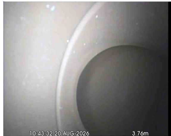
MH18X_a928e2e4-2da2-4094-816f-51954ca8c04c_20260917_172749_269.jpg, 00:00:59, 3.76 m Finish node, major connection without manhole, reference: BLIND JUNCTION - JOINS SECTION 29 (S29)
