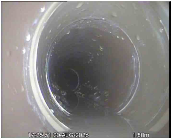
SVPX_3a130f28-d381-44ea-9998-2b1494308618_20260918_102334_975.jpg, 00:00:45, 1.80 m Water level, 5% of the vertical dimension
