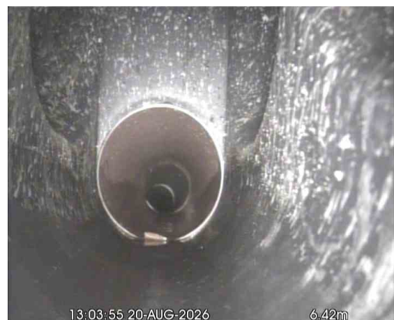
MH24X_9b2ca61f-d6e0-4dee-b5b2-998733174fa9_20260917_184230_765.jpg, 00:01:28, 6.42 m Finish node, manhole, reference: MANHOLE 9 (MH9), (F32)
