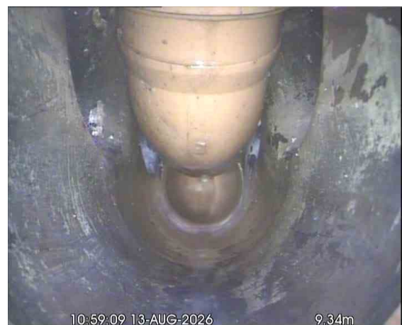
MH11 (F34)X_2c3b0f7a-188f-4f48-b23e-ffca18901513_20260917_163929_591.jpg, 00:03:12, 9.34 m Finish node, manhole, reference: MANHOLE 12 (MH12), (F35)
