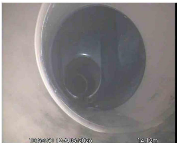
MH1 (S23)X_76bf3cf8-8282-4de9-a750-7fe0fe7e797e_20260917_155155_107.jpg, 00:03:30, 4.12 m Line deviates left
