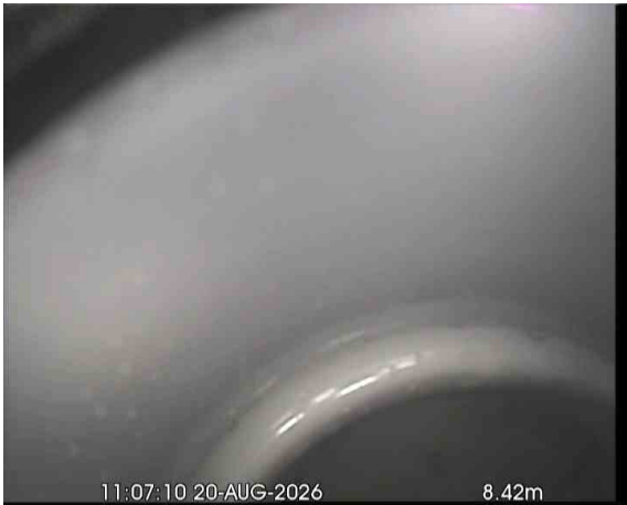
W_CX_409388aa-d100-4396-b8a9-0fc85fbb24d7_20260917_173350_054.jpg, 00:01:05, 8.42 m Finish node, major connection without manhole, reference: W/C
