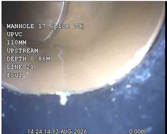
SVPX_5a0120fe-2875-4ba6-92e4-71d64a493fda_20260917_171218_915.jpg, 00:00:29, 0.00 m Start node, manhole, reference: MANHOLE 17 (MH17)
