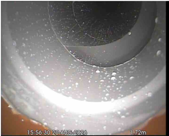
SVPX_6dcee700-b0e5-4bd0-b866-ffd0f022fe8e_20260918_093952_502.jpg, 00:00:48, 1.72 m Finish node, major connection without manhole, reference: SOIL VENT PIPE (SVP) & DOWNSTAIRS W/C
