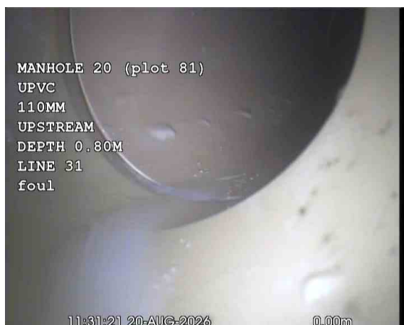
UTIL. SINKX_578b374c-c4ed-4317-960c-69d16578a319_20260917_175029_804.jpg, 00:00:17, 0.00 m Start node, manhole, reference: MANHOLE 20 (MH20)
