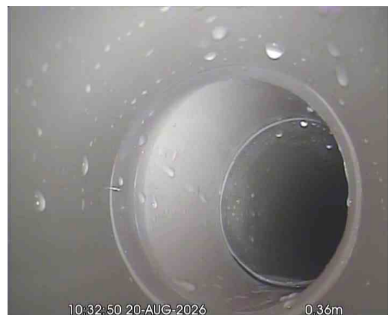
KIT. SINKX_7f6a78dd-bf72-4feb-9690-3e8ee3f130d6_20260917_172051_549.jpg, 00:00:44, 0.36 m Line deviates right
