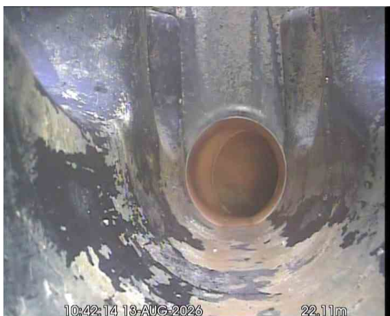
MH10 (F33)X_09784df2-4f93-46ba-9049-4ed3d1541d28_20260917_163151_061.jpg, 00:04:16, 22.11 m Finish node, manhole, reference: MANHOLE 11 (MH11), (F34)
