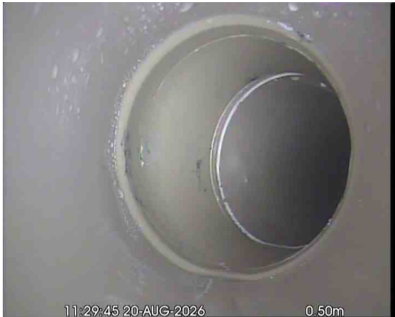
KIT. SINKX_c2e0c532-d8b6-4860-86cf-757afc9b706e_20260917_174902_799.jpg, 00:00:43, 0.50 m Line deviates right
