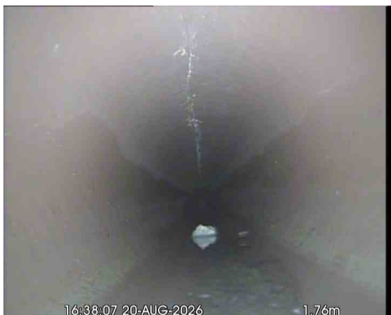
MH32X_8387c9db-cf90-4561-a64e-93d17577154f_20260918_095158_589.jpg, 00:00:34, 1.76 m Water level, 10% of the vertical dimension
