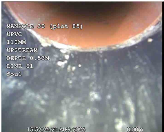
BASINX_b32eb044-732f-424e-85ef-fc1e748c28bb_20260918_093544_204.jpg, 00:00:17, 0.00 m Start node, manhole, reference: MANHOLE 30 (MH30)
