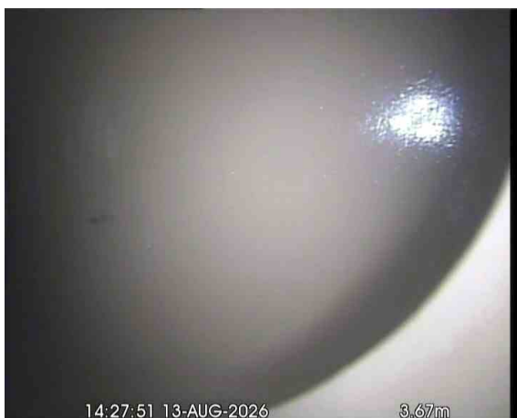
MH17X_63e6a9da-b00e-4df3-bf8a-768f73311e2a_20260917_171604_159.jpg, 00:01:39, 3.67 m Finish node, major connection without manhole, reference: BLIND JUNCTION - JOINS SECTION 16 (S16)
