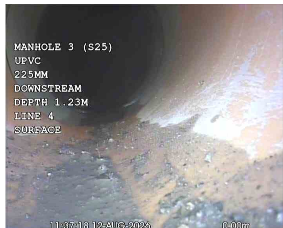
MH3 (S25)X_bbd337cd-102c-4321-9ed5-c37510282807_20260917_160249_304.jpg, 00:01:09, 0.00 m Water level, 0% of the vertical dimension
