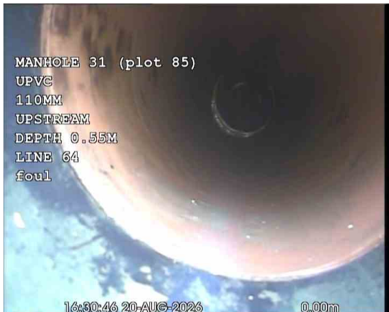
SVPX_d8ca7d10-eb8b-4d85-a6c4-8f013f9c7bcd_20260918_094423_397.jpg, 00:00:49, 0.00 m Start node, manhole, reference: MANHOLE 31 (MH31)
