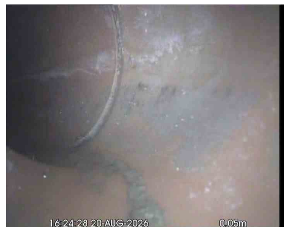
MH30X_e592d5ce-48ca-48f3-b79f-d5a45f793627_20260918_094122_115.jpg, 00:00:20, 0.05 m Line deviates left
