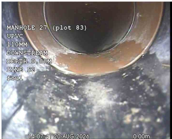
MH27X_b8072987-1f9e-42d7-9b53-a5a8ae555f10_20260917_190322_868.jpg, 00:00:25, 0.00 m Start node, manhole, reference: MANHOLE 27 (MH27)
