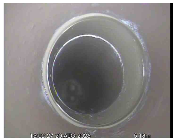
SVPX_7899bd78-7d08-4328-aeec-14e2c43b2580_20260918_091802_470.jpg, 00:00:39, 5.18 m Line deviates left
