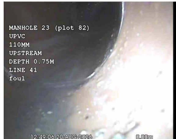
UTIL. SINKX_483d4967-86d1-467b-ac14-0623c15e0530_20260917_183535_295.jpg, 00:00:24, 0.00 m Water level, 0% of the vertical dimension
