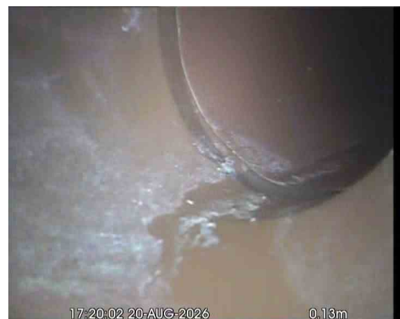
MH36X_e09b0b01-f82c-40f3-8aca-19f216624f20_20260918_102100_633.jpg, 00:00:46, 0.13 m Line deviates right
