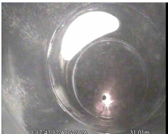
MH2 (S24)X_d71bb206-4d3c-4feb-865c-4210ee6c4161_20260917_155959_075.jpg, 00:04:36, 31.01 m Junction at 11 o'clock, diameter: 150mm
