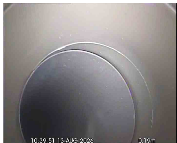
MH10 (F33)X_cf6c9501-8720-47d1-8897-0ad26da18fac_20260917_162801_379.jpg, 00:01:53, 0.19 m Line deviates left
