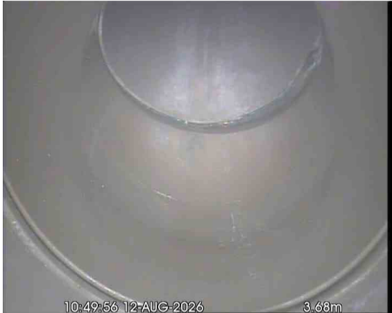
S. GULLYX_c841ab05-4e20-45ef-94d7-4ac12e3120df_20260917_155120_453.jpg, 00:01:35, 3.68 m Line deviates up
