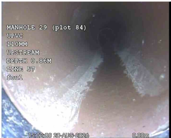
SVPX_37573cdb-8ec3-4616-a0a4-d3f7198a9f2c_20260918_091555_516.jpg, 00:00:20, 0.00 m Start node, manhole, reference: MANHOLE 29 (MH29)
