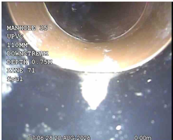
MH35X_4c7770df-1197-4553-b7e1-d152173171aa_20260918_101257_039.jpg, 00:00:16, 0.00 m Start node, manhole, reference: MANHOLE 35 (MH35)
