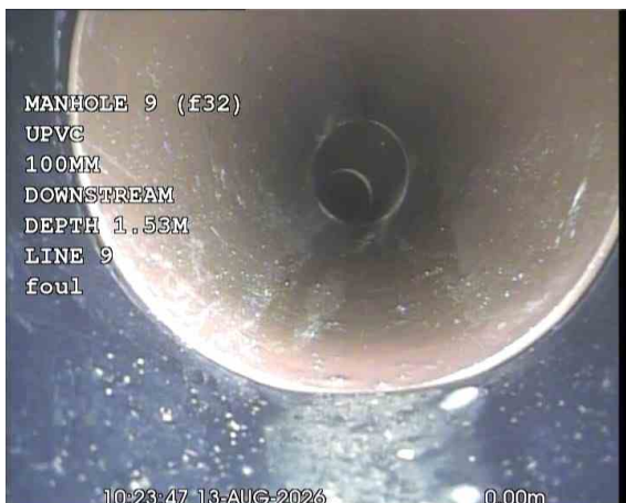
MH9 (F32)X_489cd220-7614-4143-8eff-ce8eab942a81_20260917_162353_874.jpg, 00:00:41, 0.00 m Start node, manhole, reference: MANHOLE 9 (MH9), (F32)
