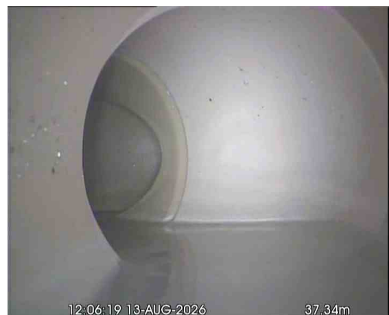
MH14 (F33AX_c8caa492-caf9-4867-bdec-ade6c186e3d0_20260917_165438_125.jpg, 00:03:18, 37.34 m Water level, 10% of the vertical dimension
