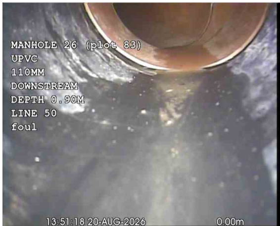
MH26X_df3942ec-aca3-4573-a697-11e0494948f6_20260917_185658_828.jpg, 00:00:24, 0.00 m Start node, manhole, reference: MANHOLE 26 (MH26)
