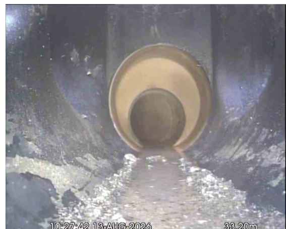
MH9 (F32)X_4e9ac8c6-0901-45d4-917d-3c1168824f94_20260917_162519_220.jpg, 00:04:36, 33.20 m Finish node, manhole, reference: MANHOLE 10 (MH10), (F33)
