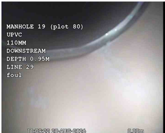
MH19X_39b1171e-fc43-48b7-acbd-f285a79238fb_20260917_173450_637.jpg, 00:00:23, 0.00 m Start node, manhole, reference: MANHOLE 19 (MH19)
