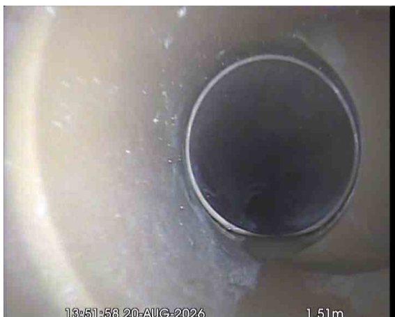
MH26X_e0202715-f291-445b-b406-8e3a656578b7_20260917_185750_378.jpg, 00:01:04, 1.51 m Junction at 3 o'clock, diameter: 110mm, SECTION 47 (S47)
