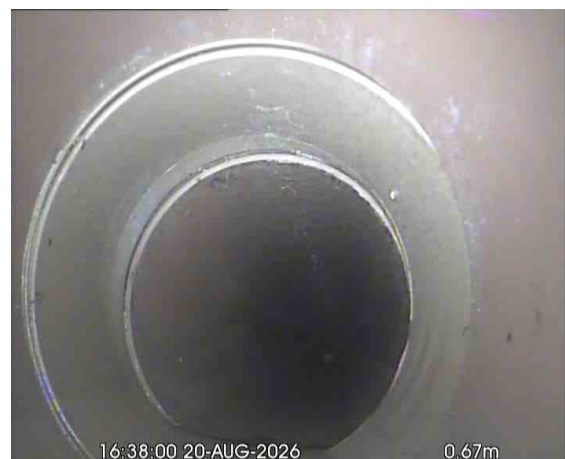
MH32X_5e0910aa-3f6e-4157-b4b1-465c047b25e9_20260918_095139_344.jpg, 00:00:28, 0.67 m Line deviates right
