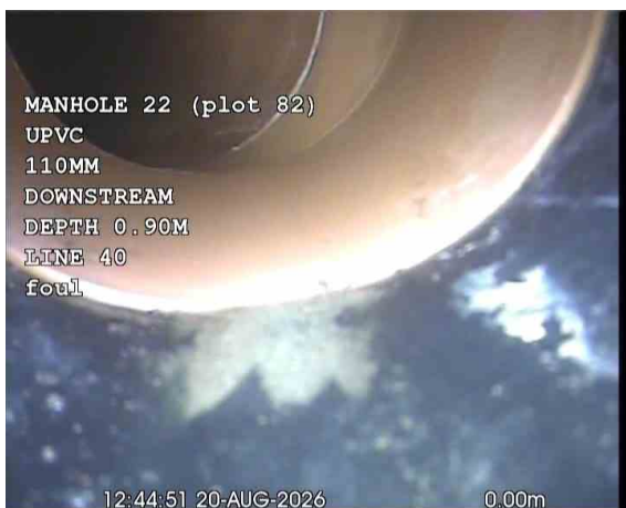
MH22X_6304265d-8e2a-4b6a-b1f2-5c4f5fd468ba_20260917_183354_669.jpg, 00:00:21, 0.00 m General remark, **PLOT 82**
