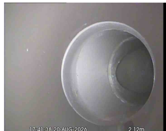
MH38X_b16c1fe1-a967-40eb-a772-f7dbd54acb74_20260918_103238_514.jpg, 00:00:33, 2.12 m Line deviates right
