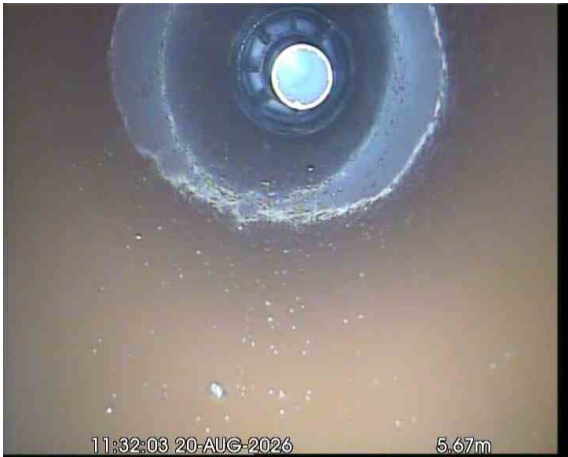
UTIL. SINKX_909ac16d-6327-4b52-9e95-248ba5637d24_20260917_175133_486.jpg, 00:00:59, 5.67 m Finish node, major connection without manhole, reference: UTILITY SINK
