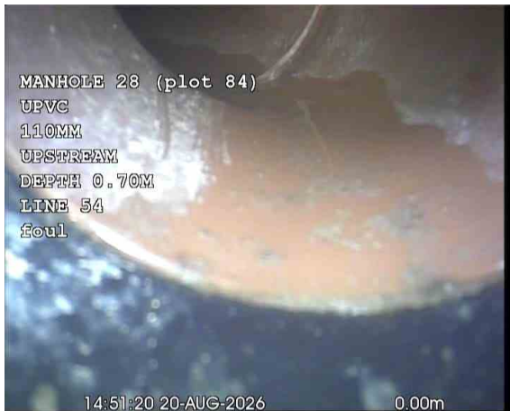
SVPX_02082cc5-32a1-4dc0-b2f7-d6bec0ddbcb2_20260918_090826_115.jpg, 00:00:27, 0.00 m Start node, manhole, reference: MANHOLE 28 (MH28)
