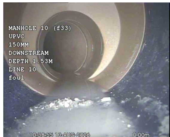
MH10 (F33)X_d878b1ba-4f3d-4473-877b-22a78de67df5_20260917_162705_885.jpg, 00:00:57, 0.00 m Water level, 5% of the vertical dimension
