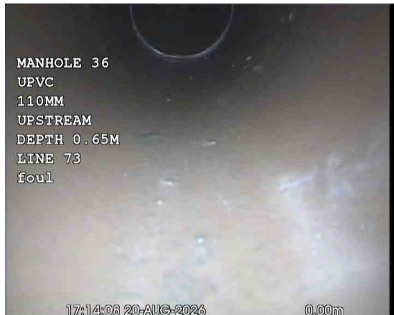
CAPPED OFFX_c9cd19b9-49db-441b-9723-6cf9d343a64c_20260918_101637_110.jpg, 00:00:11, 0.00 m Start node, manhole, reference: MANHOLE 36 (MH36)
