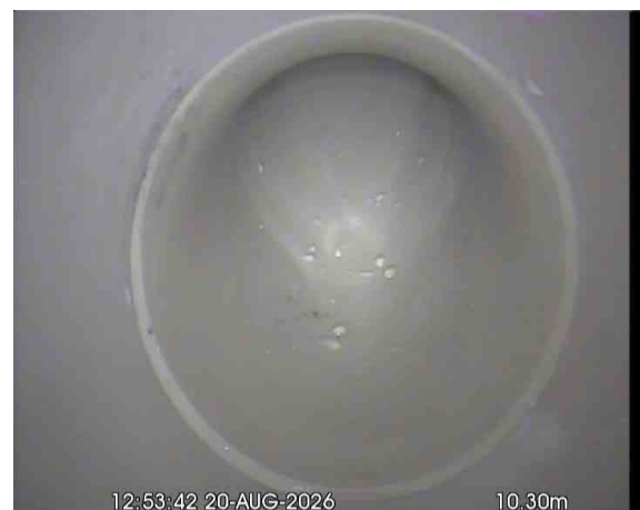
SVPX_c6a3b36b-720f-453a-9592-58dc0503e30a_20260917_183749_790.jpg, 00:01:13, 10.30 m Line deviates up, REST BEND
