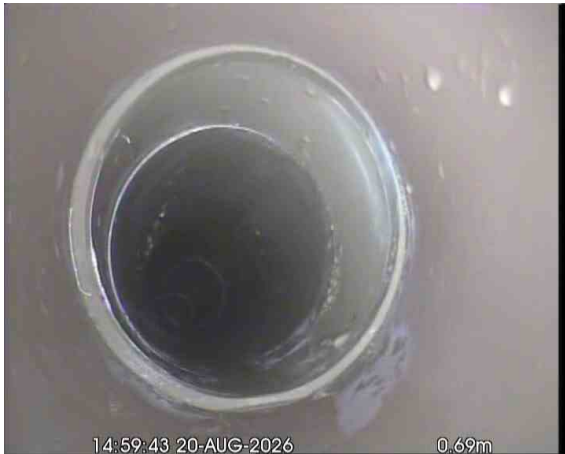
KIT. SINKX_cacbad40-2203-4c44-901a-1d7539de821b_20260918_091411_860.jpg, 00:00:28, 0.69 m Line deviates left
