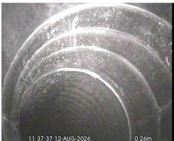
MH3 (S25)X_4ba9618a-5a5f-41f0-ae3c-0a1d373c7321_20260917_160302_250.jpg, 00:01:28, 0.26 m Line deviates left
