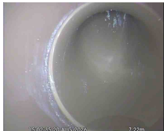
SVPX_28b784ac-d56d-4867-80d0-49573f454542_20260918_092115_855.jpg, 00:00:47, 7.22 m Line deviates up, REST BEND
