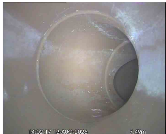
MH15X_c3dfec66-6f70-4ed8-9596-f3f5208a5763_20260917_170323_835.jpg, 00:01:26, 7.49 m Line deviates right
