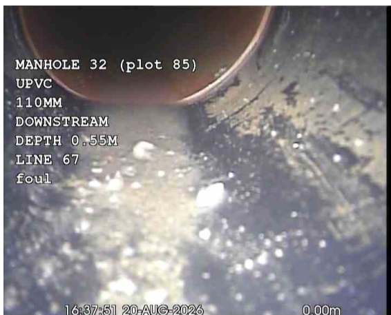
MH32X_a749461f-2d39-4856-aaf8-75adc7fa6e60_20260918_095112_484.jpg, 00:00:18, 0.00 m Start node, manhole, reference: MANHOLE 32 (MH32)
