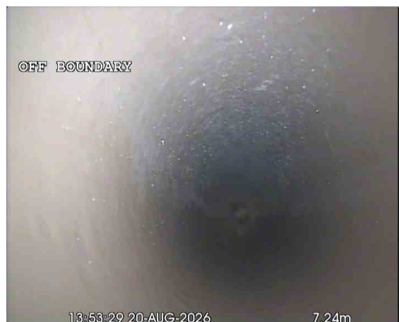
MH26X_f241e131-e784-466b-9d94-6af77b7cf11d_20260917_185848_786.jpg, 00:01:46, 7.24 m General remark, **BOUNDARY POINT**
