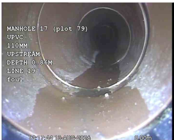
BASINX_af5ce351-2921-4ba2-bdaf-ebc53474b9f7_20260917_170828_084.jpg, 00:00:25, 0.00 m Start node, manhole, reference: MANHOLE 17 (MH17)
