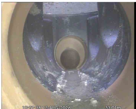
MH9 (F32)X_fd623ebe-d1d6-449f-a4a3-b1a95742cd59_20260917_162458_154.jpg, 00:04:32, 33.01 m Size changes, new size(s), 150mm high
