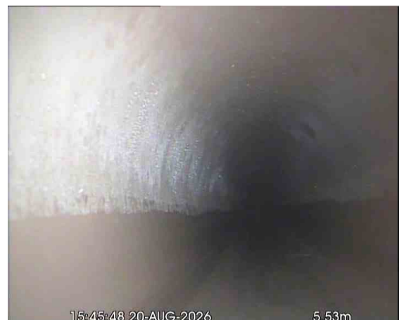
UTIL. SINKX_7a5c597b-7542-4429-bbf0-6048260c1ef1_20260918_093340_678.jpg, 00:01:18, 5.53 m Water level, 5% of the vertical dimension
