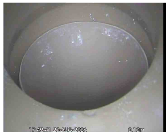
MH39X_7944ec74-93d7-4598-ac61-282eadb9ab4d_20260918_103511_794.jpg, 00:00:29, 0.10 m Line deviates down, **VERTICALLY DOWN**
