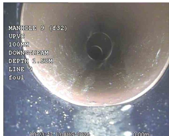
MH9 (F32)X_e3973f59-9613-42f8-9210-aab46720dede_20260917_162400_532.jpg, 00:00:41, 0.00 m Water level, 0% of the vertical dimension
