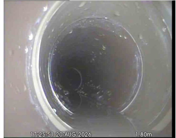
SVPX_c4796f40-e1a7-4241-85fc-d148100cf665_20260918_102327_175.jpg, 00:00:45, 1.80 m Line deviates left
