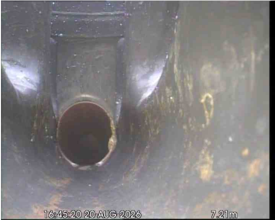
MH33X_05ca6e2c-e1cb-44b5-a9f9-6d6e8b4bc_20260918_095725_479.jpg, 00:00:57, 7.21 m Finish node, manhole, reference: MANHOLE 34 (MH34)
