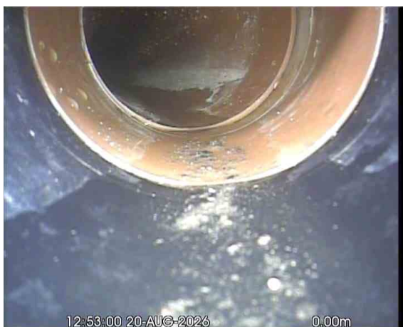
SVPX_17640d32-d379-4e05-baac-137395ff5db9_20260917_183733_366.jpg, 00:00:30, 0.02 m Line deviates left
