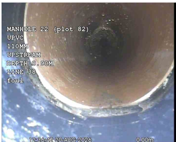
SVPX_dcb35af0-f88e-4edc-8a4a-27670d7f09f6_20260917_182951_340.jpg, 00:00:15, 0.00 m Start node, manhole, reference: MANHOLE 22 (MH22)
