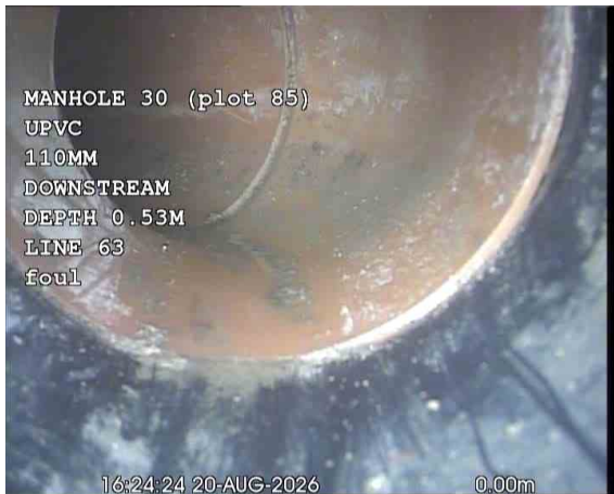
MH30X_2d32c39e-2488-4136-8f1e-d84b379d3cdd_20260918_094053_039.jpg, 00:00:17, 0.00 m Start node, manhole, reference: MANHOLE 30 (MH30)
