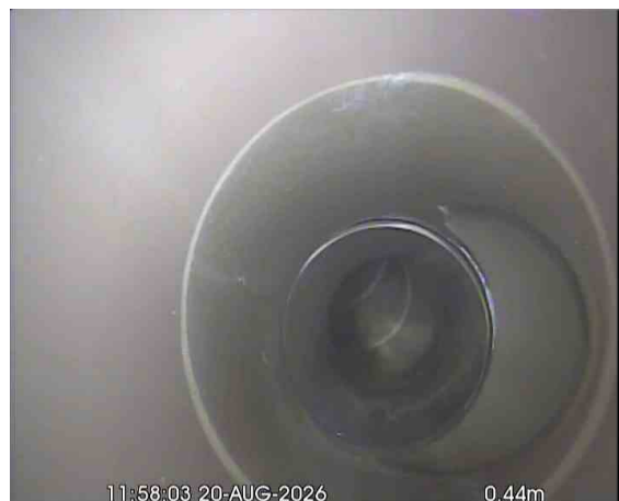
MH21X_cebf1ea1-56be-48ab-b0b2-7dd4ed90976c_20260917_182138_613.jpg, 00:00:38, 0.44 m Junction at 3 o'clock, diameter: 110mm, SECTION 32 (S32)
