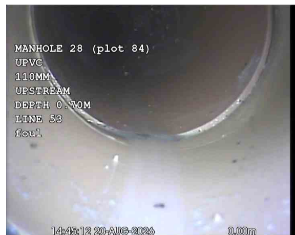
CAPPED OFFX_6a3eb29f-20be-462c-9acd-e750ac4ced1a_20260918_ 090640_574.jpg, 00:00:30, 0.02 m Line deviates left
