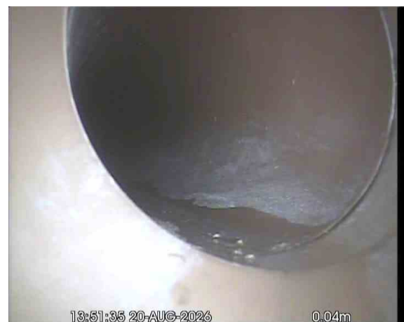
MH26X_e532ab15-eb3a-42da-84df-3b3f30bbe6c7_20260917_185727_439.jpg, 00:00:41, 0.04 m Line deviates left
