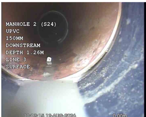
MH2 (S24)X_32ea514b-be78-46ea-86b7-50292b24514a_20260917_155635_895.jpg, 00:00:07, 0.00 m Start node, manhole, reference: MANHOLE 2 (MH2), (S24)
