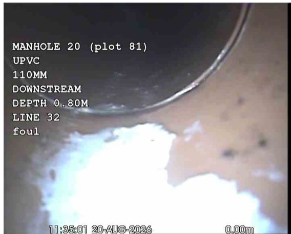
MH20X_482556e8-18fb-44d2-851f-46a30a011ab4_20260917_175228_858.jpg, 00:00:30, 0.00 m Start node, manhole, reference: MANHOLE 20 (MH20)
