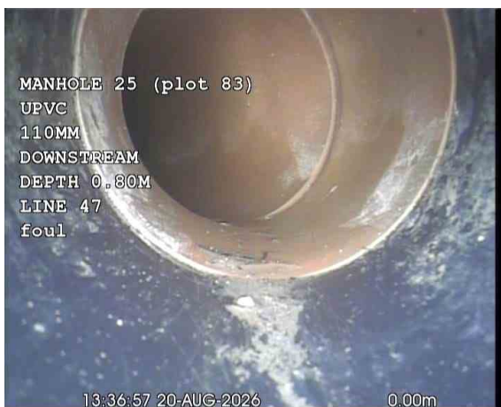
MH25X_515502b2-b2dd-488e-83c9-661ac8e3c260_20260917_185018_354.jpg, 00:00:19, 0.00 m General remark, **PLOT 83**
