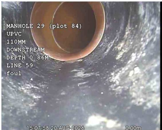
MH29X_915e2cf9-5035-452c-b7bc-f39c08b0d4a7_20260918_092704_584.jpg, 00:00:18, 0.00 m Start node, manhole, reference: MANHOLE 29 (MH29)
