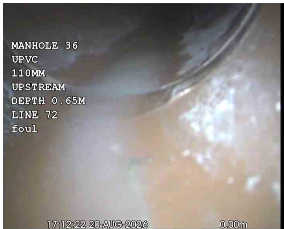
SVPX_e944b52e-348b-4bb0-bb42-e3366dd31f44_20260918_101443_234.jpg, 00:00:19, 0.00 m Start node, manhole, reference: MANHOLE 36 (MH36)
