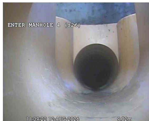
MH3 (S25)X_a07b1e89-ad44-4d33-956a-2a54c47cce03_20260917_160326_826.jpg, 00:02:57, 9.02 m Finish node, manhole, reference: MANHOLE 4 (MH4), (S26)
