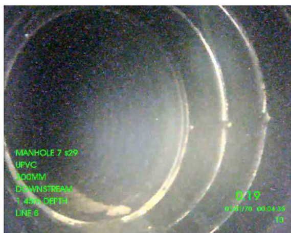
MH7 (S29)X_d7dcf0f8-609e-4756-ba6c-0d55cc8bb014_20260917_161846.png, 0.19 m Line deviates right
