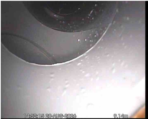
SVPX_9ea43e84-82a3-437b-893d-5aa136d075fe_20260918_090939_640.jpg, 00:01:21, 9.14 m Finish node, major connection without manhole, reference: SOIL VENT PIPE (SVP) & DOWNSTAIRS W/C
