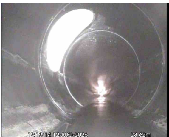
MH5 (S26)X_65b27f55-c831-4031-afb9-47e4ef07d4c3_20260917_160551_209.jpg, 00:04:51, 28.62 m Junction at 10 o'clock, diameter: 150mm
