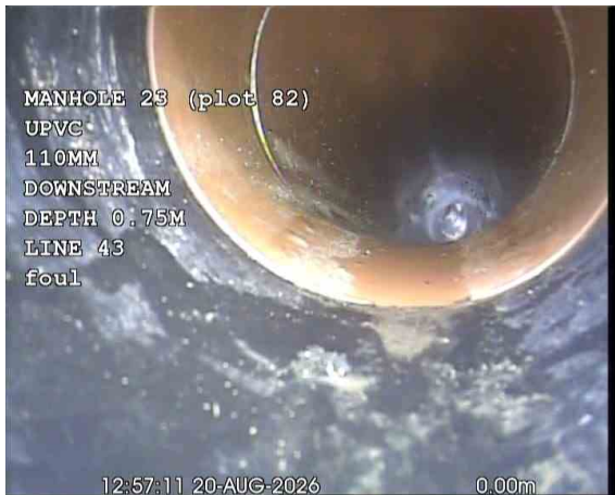
MH23X_2e07efe7-02fa-4850-b759-3bf05391faf_20260917_183910_280.jpg, 00:00:18, 0.00 m Start node, manhole, reference: MANHOLE 23 (MH23)
