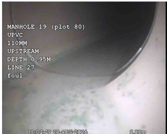
BASINX_7d255818-8980-4b5b-9301-0e50d3741451_20260917_172918_690.jpg, 00:00:54, 0.00 m Start node, manhole, reference: MANHOLE 19 (MH19)
