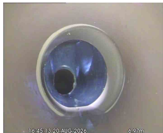
MH33X_7969662a-4f60-406a-8183-673844b0759d_20260918_095704_584.jpg, 00:00:50, 6.97 m Line deviates left
