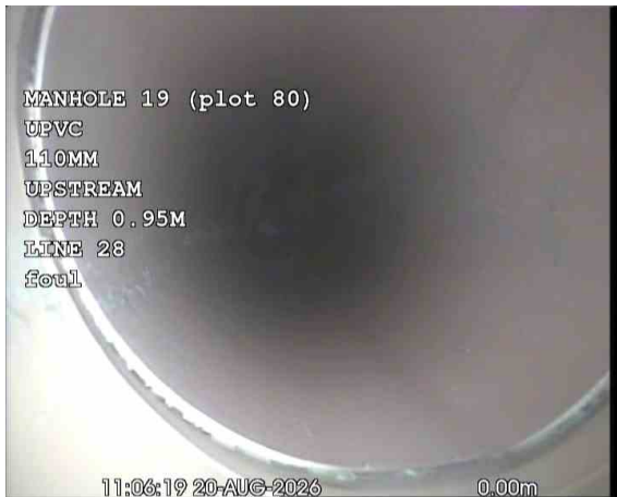
W_CX_114763e0-15fc-4e1f-885e-ab74307a7e63_20260917_173236_658.jpg, 00:00:14, 0.00 m Start node, manhole, reference: MANHOLE 19 (MH19)
