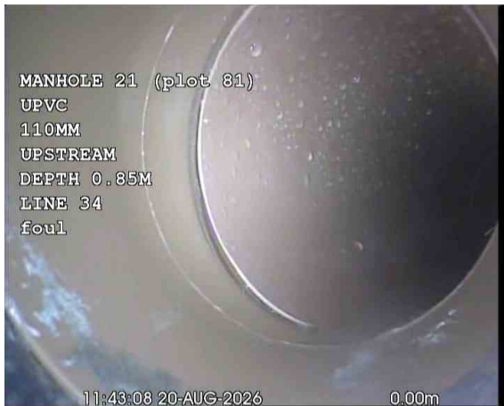
BASINX_3ce3f895-d02d-466c-8391-f9e368b19190_20260917_175733_165.jpg, 00:00:22, 0.00 m Start node, manhole, reference: MANHOLE 21 (MH21)
