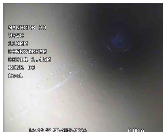
MH33X_7e40d295-b96c-4b4d-aae4-fdb9dc3b0372_20260918_095456_010.jpg, 00:00:25, 0.00 m Water level, 0% of the vertical dimension
