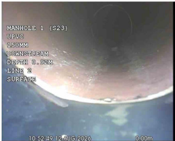
MH1 (S23)X_4d4814a7-cf8b-4114-976f-03e03bb0a39d_20260917_155148_736.jpg, 00:00:30, 0.00 m Start node, manhole, reference: MANHOLE 1 (MH1), (S23)
