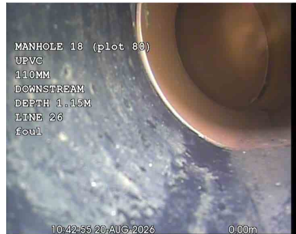
MH18X_d190bcd2-5cb7-42a8-a38a-37c5f93c884b_20260917_172630_110.jpg, 00:00:21, 0.00 m Water level, 0% of the vertical dimension
