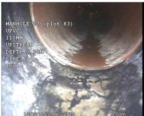
SVPX_e3fe6dbd-809f-442a-9bbd-239b3fc9dbe0_20260917_190034_222.jpg, 00:00:21, 0.00 m Start node, manhole, reference: MANHOLE 27 (MH27)
