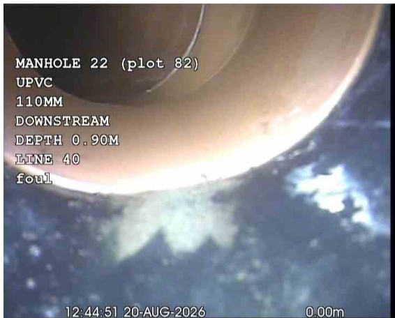
MH22X_06481b2a-6201-4c44-bc15-0ddffc2c6d1e_20260917_183341_955.jpg, 00:00:21, 0.00 m Start node, manhole, reference: MANHOLE 22 (MH22)
