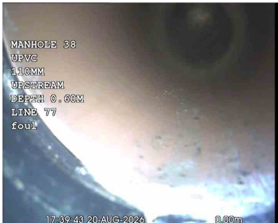
SVPX_b22644d8-a6d2-40e5-8027-5581d46c021f_20260918_103014_530.jpg, 00:00:40, 0.00 m Start node, manhole, reference: MANHOLE 38 (MH38)
