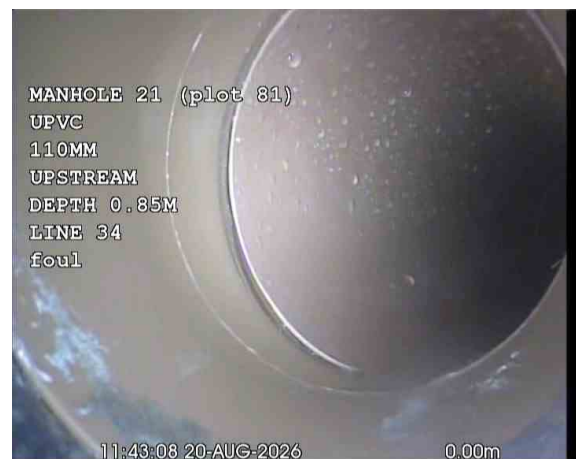
BASINX_174c6773-1f98-49d0-8a46-bf51393b0f07_20260917_175755_367.jpg, 00:00:22, 0.02 m Line deviates right
