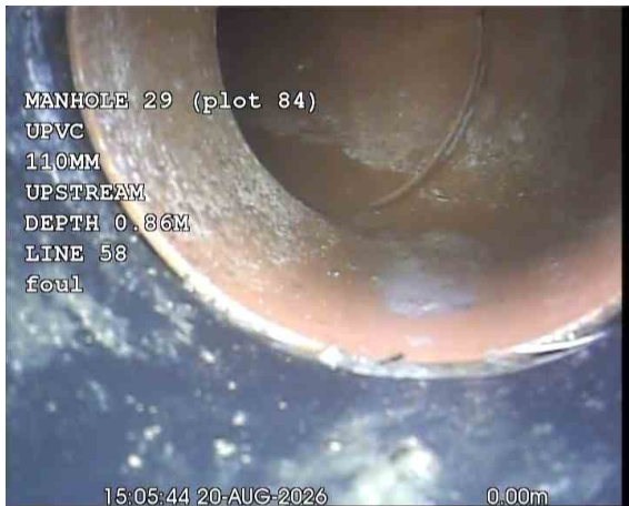
SVPX_6bddfa59-6e48-495d-ad33-15f4c2e595df_20260918_092242_050.jpg, 00:00:17, 0.00 m Start node, manhole, reference: MANHOLE 29 (MH29)
