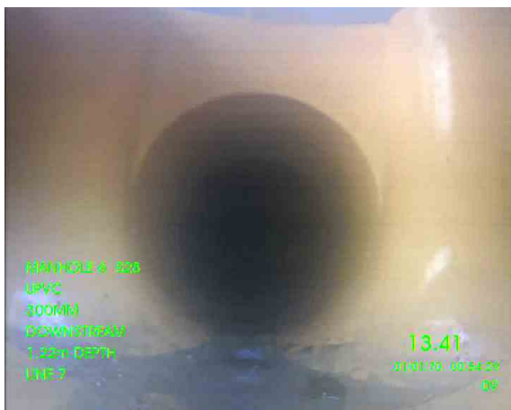
MH6 (S28)X_7e920f37-da11-4577-bff2-d13314ea7b33_20260917_ 161500.png, 13.41 m Finish node, manhole, reference: MANHOLE 7 (MH7), (S29)
