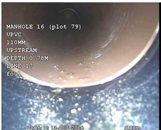
SVPX_f04ced03-d09c-4ac6-97e2-8e53969a3199_20260917_170448_268.jpg, 00:00:23, 0.00 m Start node, manhole, reference: MANHOLE 16 (MH16)
