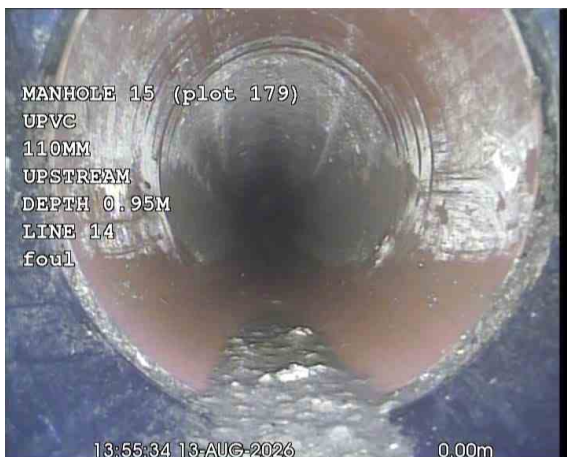
SVPX_b177d65f-3e32-4885-93b1-34f03347b9b5_20260917_165723_780.jpg, 00:00:31, 0.00 m Start node, manhole, reference: MANHOLE 15 (MH15)
