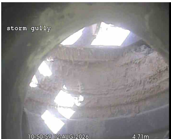
S. GULLYX_3b60e3f0-573d-481c-b75f-bc5ef4611ab7_20260917_155150_610.jpg, 00:01:57, 4.71 m Finish node, gully, reference: STORM GULLY
