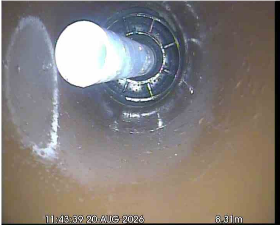
BASINX_d5c22b29-dda7-4334-9cbb-2a31b3a5bf66_20260917_175832_110.jpg, 00:00:54, 8.31 m Finish node, major connection without manhole, reference: BASIN
