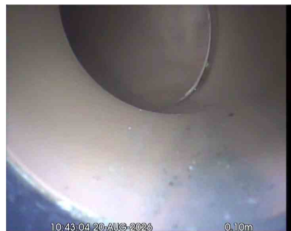
MH18X_fc59def7-a7fe-4719-bfc2-ec6431eecb40_20260917_172649_229.jpg, 00:00:30, 0.10 m Line deviates left
