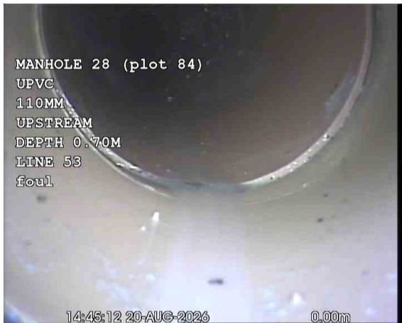
CAPPED OFFX_750fa9a6-73ff-401b-9c07-3590f6c37903_20260918_09 0618_818.jpg, 00:00:30, 0.00 m Start node, manhole, reference: MANHOLE 28 (MH28)
