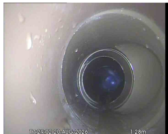
MH37X_dafdb3b2d-29d2-4ee2-bac9-e90bb8103ebb_20260918_102819_720.jpg, 00:00:34, 1.28 m Junction at 3 o'clock, diameter: 110mm, SECTION 78 (S78)
