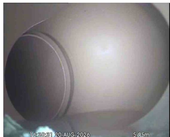
MH32X_3caed786-831d-4c98-978c-eb59492bdba9_20260918_095311_456.jpg, 00:00:58, 5.95 m Finish node, major connection without manhole, reference: BLIND JUNCTION - JOINS SECTION 63 (S63)
