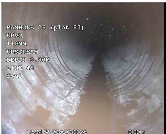
SVPX_cff1c84-fc60-40cd-a8a3-08646aed5a47_20260917_185501_819.jpg, 00:00:20, 0.00 m Start node, manhole, reference: MANHOLE 26 (MH26)
