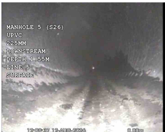
MH5 (S26)X_049c4293-9789-4496-bf72-6fb8cae8a49a_20260917_160501_585.jpg, 00:01:14, 0.00 m Start node, manhole, reference: MANHOLE 5 (MH5), (S26)
