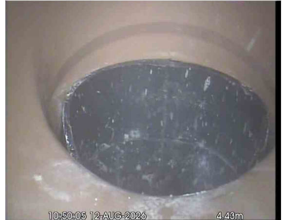
S. GULLYX_23b6788d-ddfa-4c0f-988e-e3344ba8fbbe_20260917_155137_696.jpg, 00:01:45, 4.43 m Line deviates down
