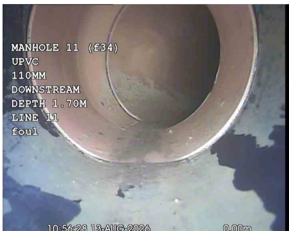
MH11 (F34)X_7c6f545c-8f02-44fd-9219-0492384b7187_20260917_163842_569.jpg, 00:00:31, 0.00 m Start node, manhole, reference: MANHOLE 11 (MH11), (F34)
