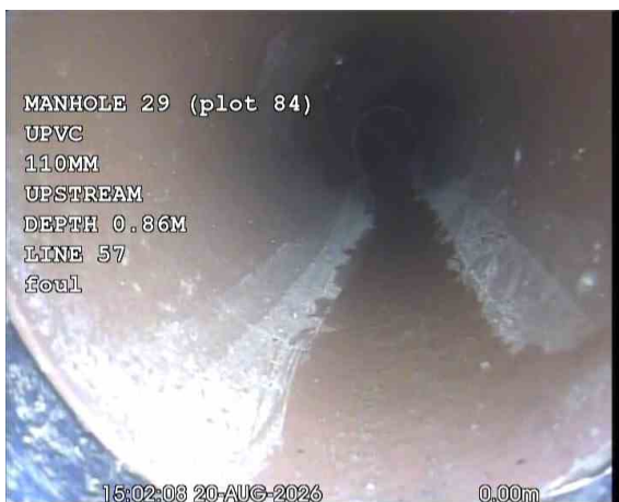
SVPX_f31f19a1-16f7-4b9c-944a-573df4eff671_20260918_091616_901.jpg, 00:00:20, 0.00 m General remark, **PLOT 84**
