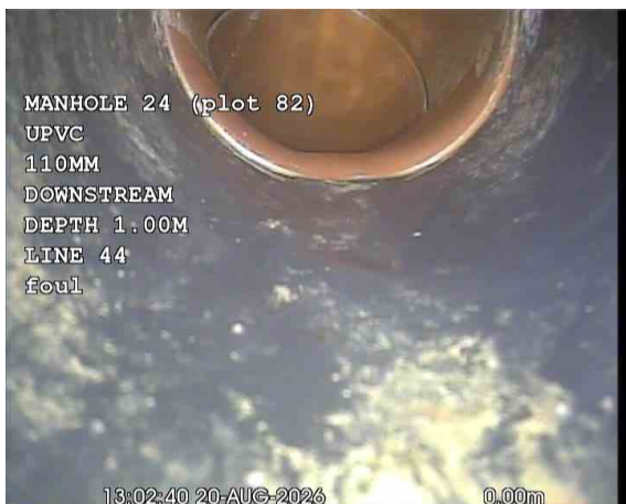
MH24X_74176b70-0352-48b6-8c17-b7cb16e8dd27_20260917_184100_499.jpg, 00:00:18, 0.00 m Start node, manhole, reference: MANHOLE 24 (MH24)
