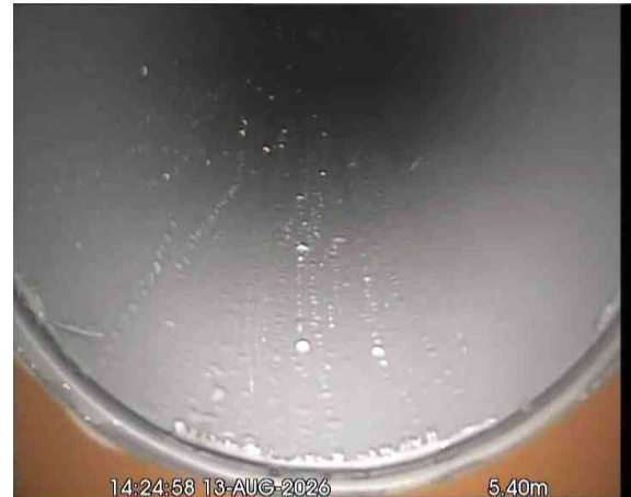
SVPX_f5641a2a-3f0d-4dfb-9118-07a890dbf729_20260917_171329_515.jpg, 00:01:13, 5.40 m Finish node, major connection without manhole, reference: SOIL VENT PIPE (SVP)
