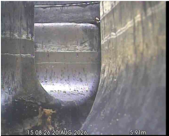
MH29X_90cc19f5-3069-4695-88a9-8e6927d34d75_20260918_092811_843.jpg, 00:00:46, 5.91 m Finish node, manhole, reference: MANHOLE 33 (MH33)
