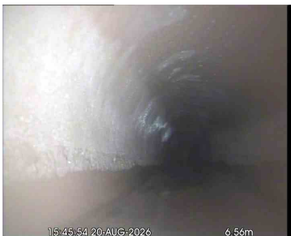
UTIL. SINKX_a729455a-41df-4ff1-8b30-236bad8511af_20260918_093357_871.jpg, 00:01:24, 6.56 m Water level, 10% of the vertical dimension
