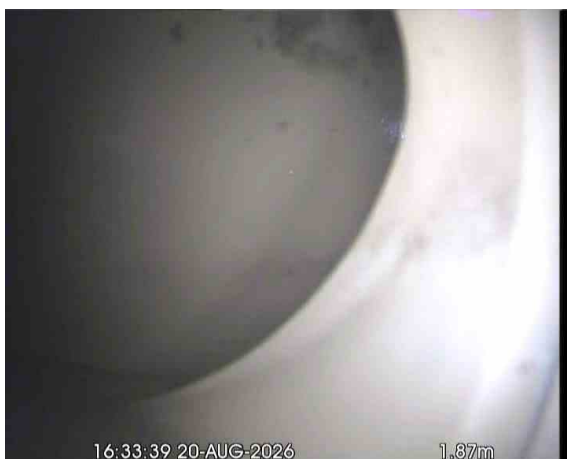
MH31X_572c7c30-c072-400f-bbda-de16bf5a7652_20260918_094817_536.jpg, 00:00:42, 1.87 m Finish node, major connection without manhole, reference: BLIND JUNCTION - JOINS SECTION 63 (S63)
