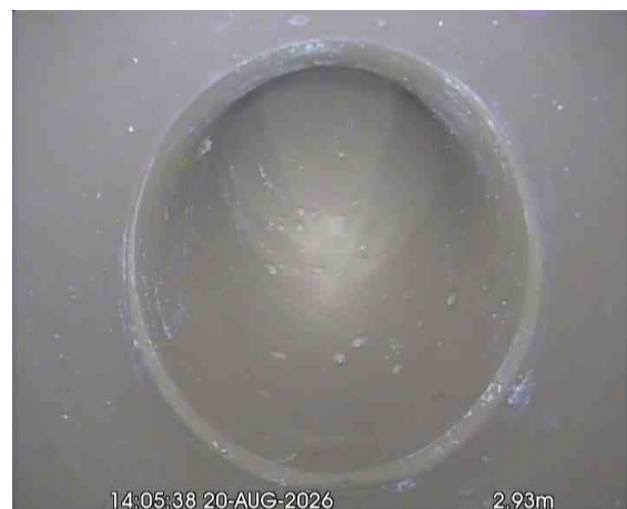
SVPX_4137f733-8701-4420-a8a6-eda23250ee5a_20260917_190105_466.jpg, 00:00:43, 2.93 m Line deviates up, REST BEND
