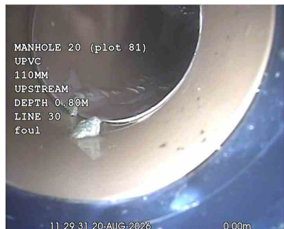
KIT. SINKX_a24192a0-7b26-4fed-8ce3-1a6fc3fda468_20260917_174849_550.jpg, 00:00:29, 0.04 m Line deviates right
