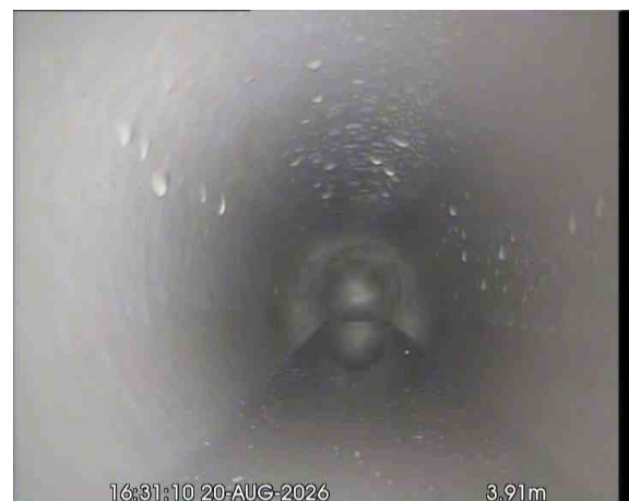
SVPX_bc697c7c-1b60-4529-9309-0248e86da1ea_20260918_094451_739.jpg, 00:01:14, 3.91 m Water level, 10% of the vertical dimension
