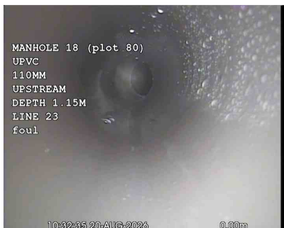
KIT. SINKX_127a114f-22b0-4eed-beac-47838286044a_20260917_172027_464.jpg, 00:00:29, 0.00 m Start node, manhole, reference: MANHOLE 18 (MH18)
