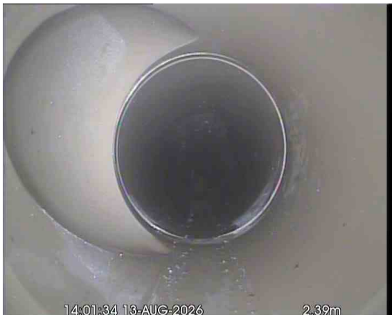
MH15X_5f45bb79-bc8c-4ba4-a2ae-7eff7c7fb217_20260917_170239_300.jpg, 00:00:46, 2.39 m Junction at 9 o'clock, diameter: 110mm, SECTION 22 (S22)
