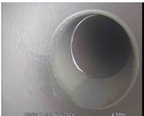
MH26X_8d16dd87-7703-4d23-96b7-7e473cd8e2cc_20260917_185826_415.jpg, 00:01:33, 4.99 m Line deviates right
