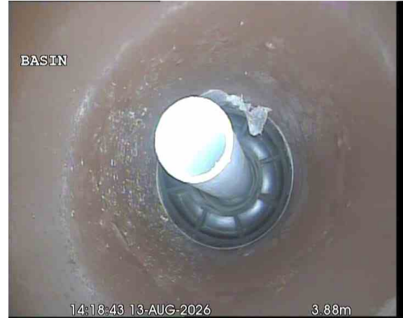
BASINX_bfb68a32-918e-4b3d-bd2d-c11b1287306e_20260917_170930_804.jpg, 00:01:14, 3.88 m Finish node, major connection without manhole, reference: BASIN
