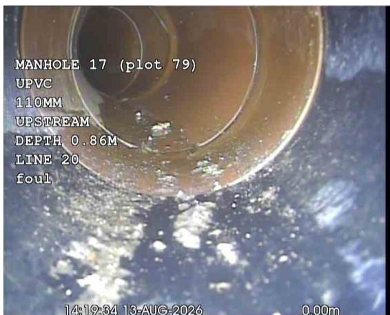
W_CX_1abf18ae-b3bd-411c-819f-99249c00b505_20260917_171020_769.jpg, 00:00:19, 0.00 m Start node, manhole, reference: MANHOLE 17 (MH17)
