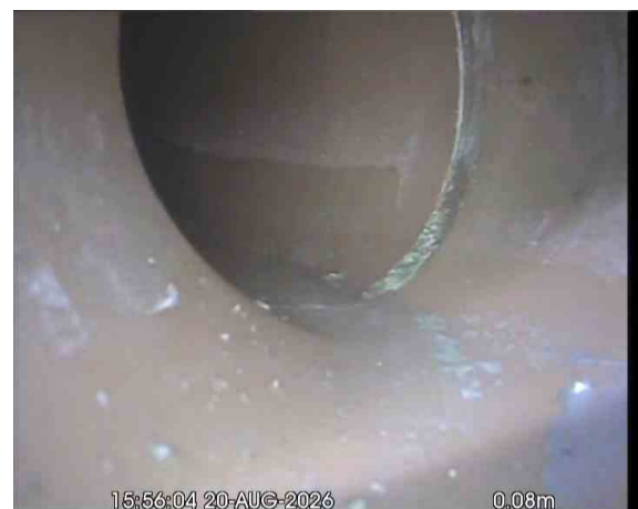
SVPX_3c8cd955-9b13-4dbc-8055-8037fb39841c_20260918_093910_496.jpg, 00:00:22, 0.08 m Line deviates left
