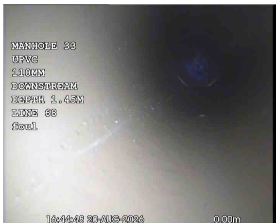
MH33X_77f784f2-afc8-470c-9a12-32775e750e11_20260918_095512_141.jpg, 00:00:25, 0.00 m General remark, **PLOT 85 & 84**
