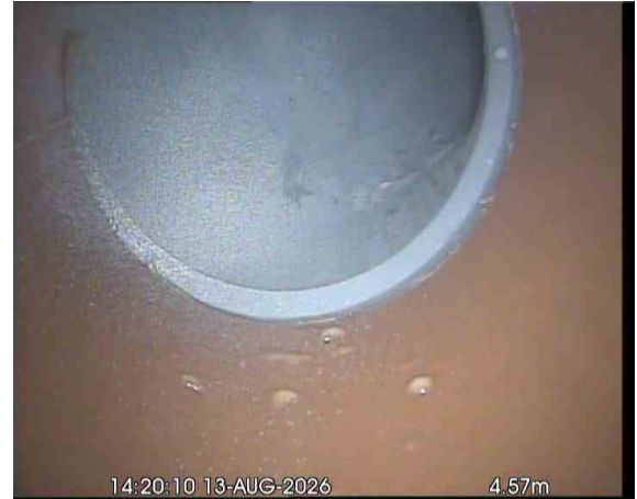
W_CX_6c84b869-0fbf-4491-b149-1df9dedb4af4_20260917_171124_774.jpg, 00:00:54, 4.57 m Finish node, major connection without manhole, reference: W/C
