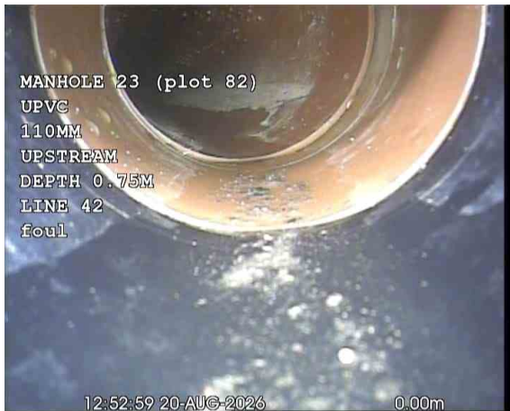
SVPX_158096e1-881e-4ce5-9f80-a11f19a6f17d_20260917_183711_515.jpg, 00:00:29, 0.00 m Start node, manhole, reference: MANHOLE 23 (MH23)
