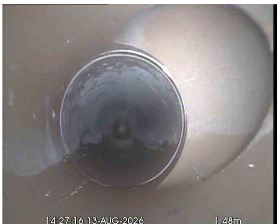
MH17X_29239583-7e43-4c4c-8f21-8b2c144d30ed_20260917_171521_414.jpg, 00:01:04, 1.48 m Junction at 3 o'clock, diameter: 110mm, SECTION 18 (S18)
