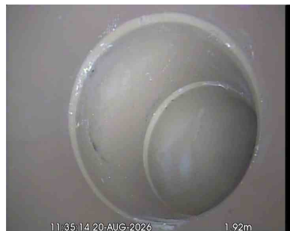
MH20X_6593b2f0-fa2f-4709-a780-fbc6a0b13676_20260917_175258_119.jpg, 00:00:42, 1.92 m Line deviates right
