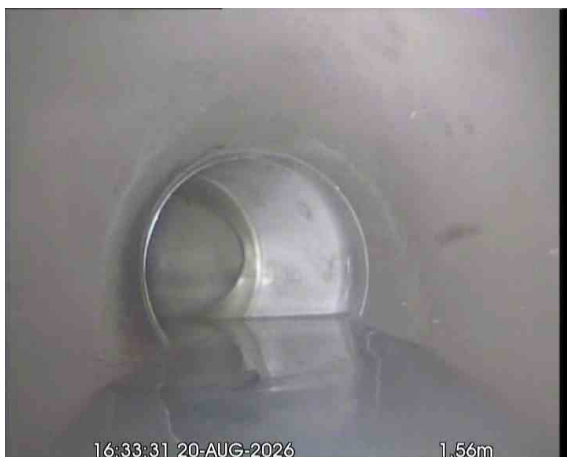
MH31X_886aa7a1-9acc-4338-9464-57e2dbb4c92f_20260918_094737_144.jpg, 00:00:34, 1.56 m Water level, 10% of the vertical dimension
