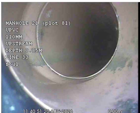
SVPX_f2157d9c-c9bd-431d-9665-e0a8a52972c7_20260917_175442_091.jpg, 00:00:40, 0.00 m Start node, manhole, reference: MANHOLE 21 (MH21)
