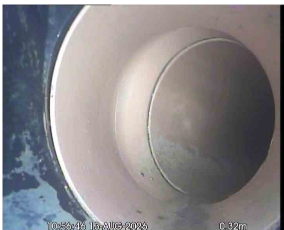
MH11 (F34)X_5ef1f7c6-ea67-4b36-998e-debf4a3d4f3e_20260917_163906_805.jpg, 00:00:49, 0.32 m Line deviates right
