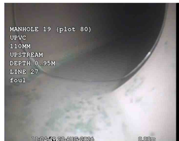
BASINX_68b4a55a-693d-4c87-8654-4240521c9e41_20260917_172940_995.jpg, 00:00:56, 0.02 m Line deviates right
