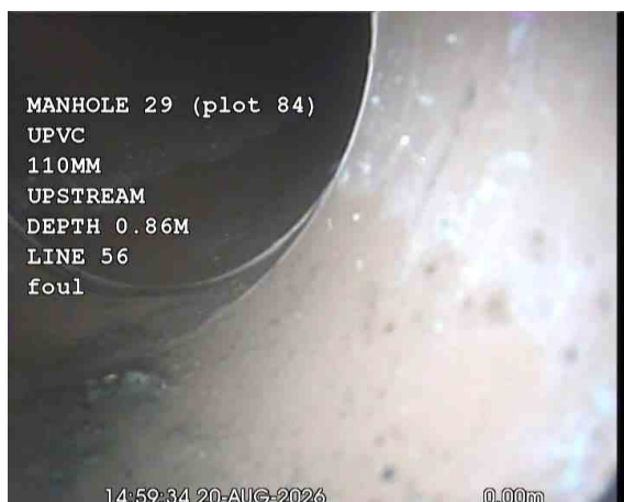
KIT. SINKX_38226131-854a-4229-8172-206b4c21a6a4_20260918_091323_039.jpg, 00:00:19, 0.00 m Start node, manhole, reference: MANHOLE 29 (MH29)
