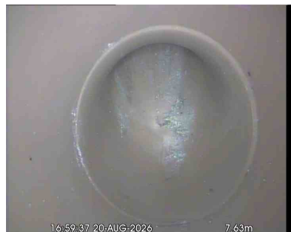
SVPX_897eb8ea-979f-4907-96d5-132e957b8e94_20260918_100927_359.jpg, 00:00:50, 7.63 m Line deviates up, REST BEND
