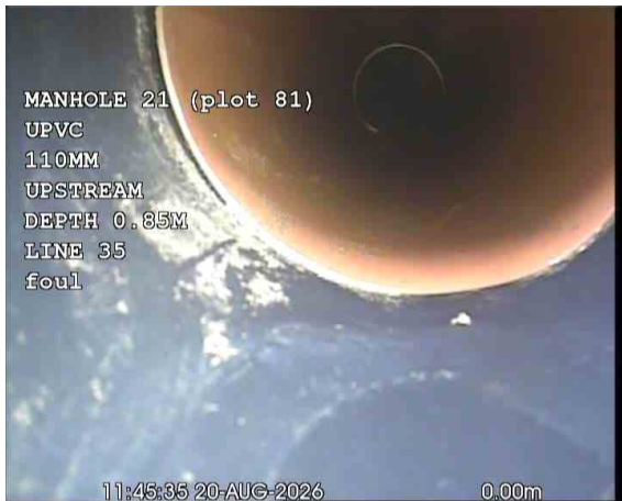
W_CX_be5123c8-25b0-4dcb-8499-8a13e69a35a2_20260917_181507_926.jpg, 00:00:20, 0.00 m Start node, manhole, reference: MANHOLE 21 (MH21)
