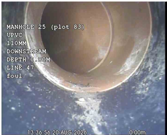
MH25X_ad981f67-90cc-45bc-a8a3-6a0eda50f06e_20260917_184954_605.jpg, 00:00:18, 0.00 m Start node, manhole, reference: MANHOLE 25 (MH25)
