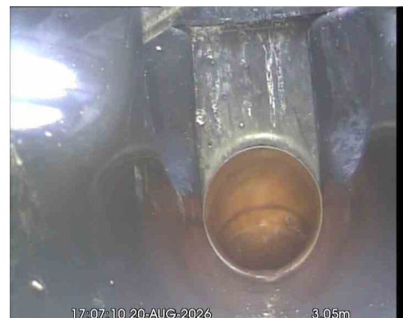
MH35X_ee4fe31a-49f5-4de4-b501-2b71efe3fd7b_20260918_101336_578.jpg, 00:00:36, 3.05 m Finish node, manhole, reference: MANHOLE 39 (MH39)
