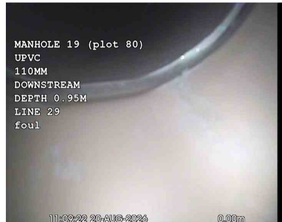
MH19X_4c81dade-bbaa-422a-a8e6-f72ab22431fd_20260917_173456_756.jpg, 00:00:23, 0.00 m Water level, 0% of the vertical dimension
