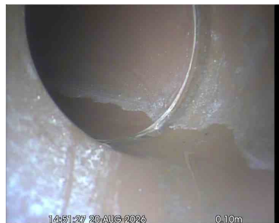
SVPX_ac7e61a2-c9ab-445d-b6f4-5a7d93b10f49_20260918_090851_753.jpg, 00:00:34, 0.10 m Line deviates left
