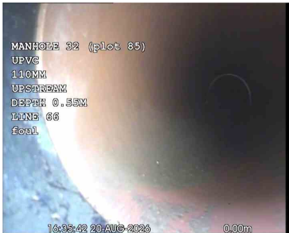
KIT. SINKX_6a6819dd-8a78-48b7-ae54-d48514df1eb1_20260918_094923_844.jpg, 00:00:17, 0.00 m Start node, manhole, reference: MANHOLE 32 (MH32)
