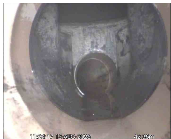
MH12 (F35)X_76902c83-d27e-4e16-98a6-616105d60454_20260917_165241_666.jpg, 00:04:47, 42.35 m Size changes, new size(s), 150mm high
