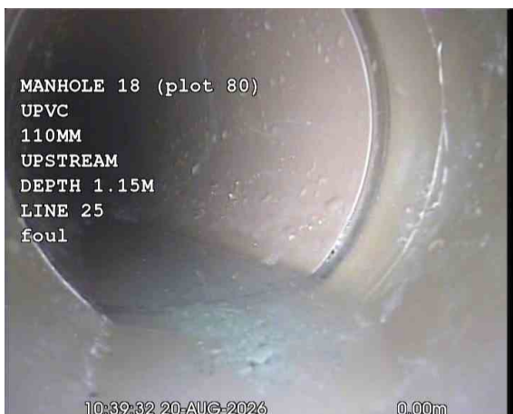
SVPX_0b274464-3330-45b2-9a17-49441895e9ff_20260917_172453_434.jpg, 00:00:33, 0.02 m Line deviates left
