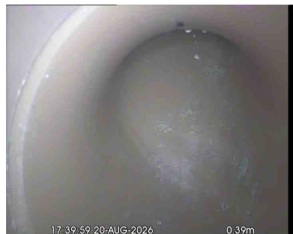
SVPX_3c8021a0-9ee2-4aa2-984c-97cee8fa075c_20260918_103043_648.jpg, 00:00:56, 0.39 m Line deviates up, REST BEND
