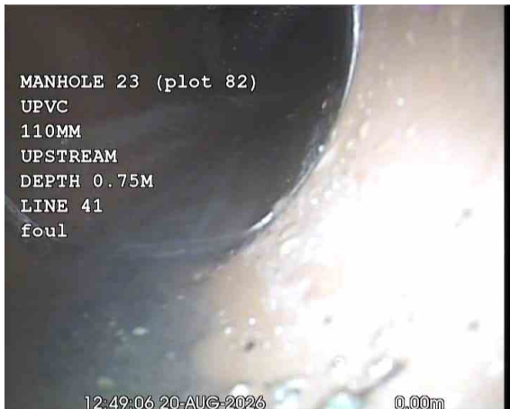
UTIL. SINKX_a1e3df06-70ba-4eaf-a188-2cd1ce9911b1_20260917_183529_173.jpg, 00:00:24, 0.00 m Start node, manhole, reference: MANHOLE 23 (MH23)
