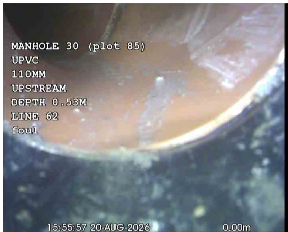
SVPX_0d1ca588-7d4d-4e9b-9296-3c992dfe303f_20260918_093842_294.jpg, 00:00:16, 0.00 m Start node, manhole, reference: MANHOLE 30 (MH30)
