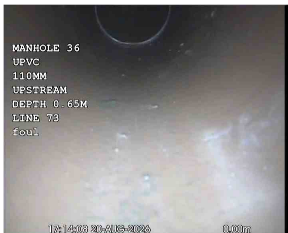
CAPPED OFFX_d28d7176-f54f-402d-9599-3ca24def1ea5_20260918_101711_413.jpg, 00:00:11, 0.00 m General remark, **PLOT 90**
