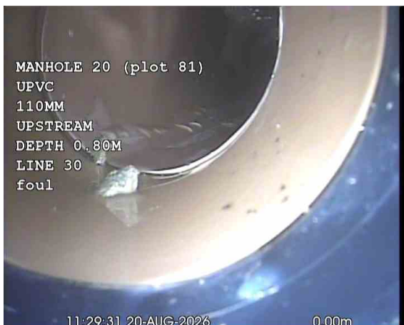
KIT. SINKX_528fc05f-cfd7-4f01-8447-395349a6ec3c_20260917_174823_422.jpg, 00:00:29, 0.00 m Start node, manhole, reference: MANHOLE 20 (MH20)
