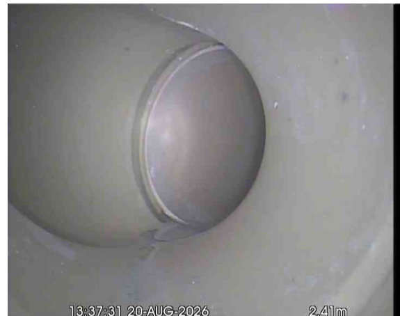
MH25X_5cc29811-30cf-4776-b1e2-48c33b9716a4_20260917_185118_701.jpg, 00:00:52, 2.41 m Finish node, major connection without manhole, reference: BLIND JUNCTION - JOINS SECTION 50 (S50)
