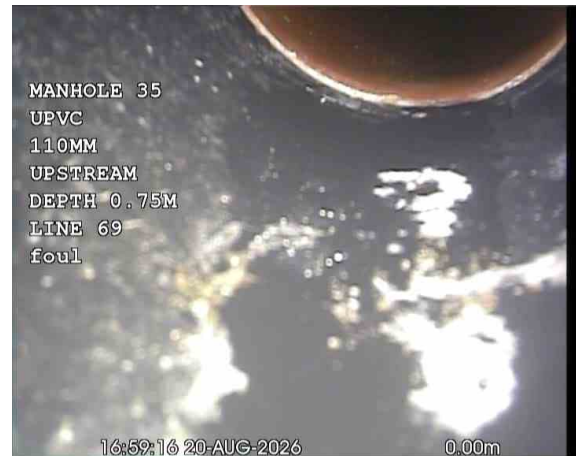
SVPX_736e7c03-119a-40f7-8979-e1b3106d80d4_20260918_100902_447.jpg, 00:00:29, 0.00 m Water level, 0% of the vertical dimension
