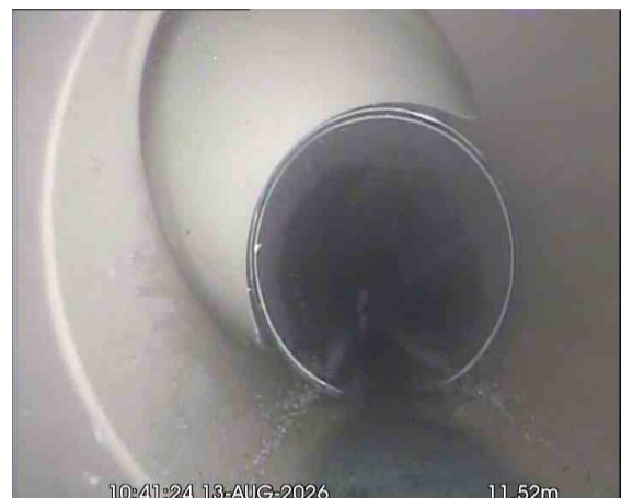
MH10 (F33)X_bf568a71-e48d-480d-80ff-eb7b6dc9d9f_20260917_163054_265.jpg, 00:03:26, 11.52 m Junction at 10 o'clock, diameter: 110mm
