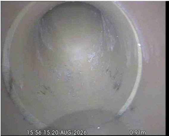
SVPX_dc1d9c19-7e35-43b5-9efa-c37a1a9c5eeb_20260918_093926_890.jpg, 00:00:33, 0.91 m Line deviates up, REST BEND
