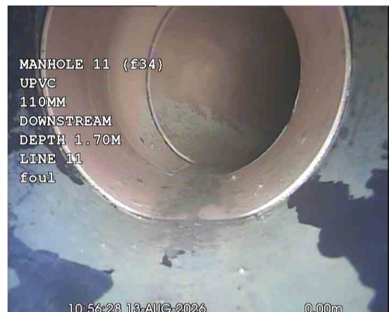
MH11 (F34)X_136808cb-5ccc-4bae-9277-86e9c56e0d3a_20260917_163848_292.jpg, 00:00:31, 0.00 m Water level, 0% of the vertical dimension
