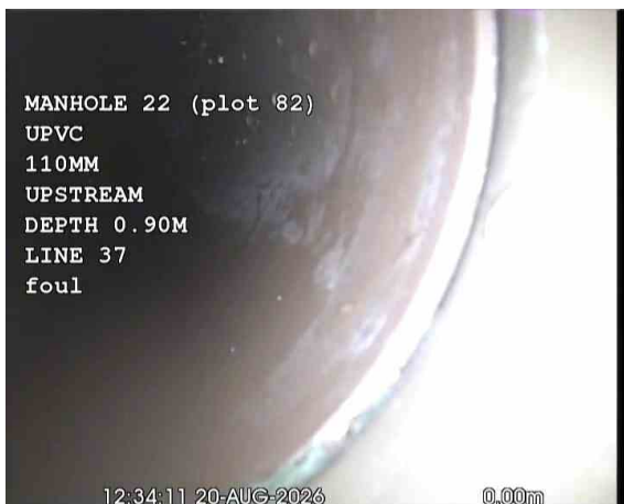
SVPX_329580d6-76e8-42e0-b84f-8c142b0f265b_20260917_182810_838.jpg, 00:00:37, 0.00 m Start node, manhole, reference: MANHOLE 22 (MH22)
