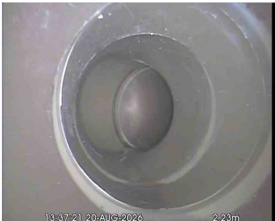
MH25X_0633491a-78ff-4ad8-9e9c-8e7e21fadc38_20260917_185042_809.jpg, 00:00:43, 2.23 m Line deviates left
