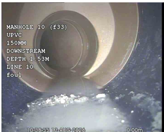
MH10 (F33)X_53dbb7e5-9dde-4b18-97cf-4fa8b41e333a_20260917_162659_649.jpg, 00:00:57, 0.00 m Start node, manhole, reference: MANHOLE 10 (MH10), (F33)
