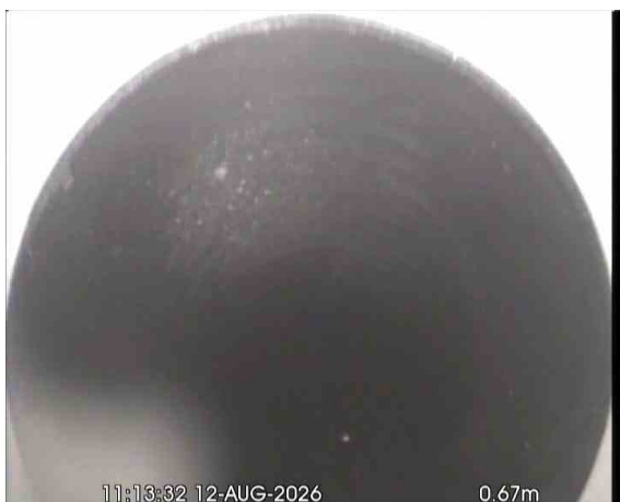
MH2 (S24)X_1640f63c-28bf-45fc-97de-4cd679e228b3_20260917_155700_752.jpg, 00:00:25, 0.67 m Size changes, new size(s), 225mm high
