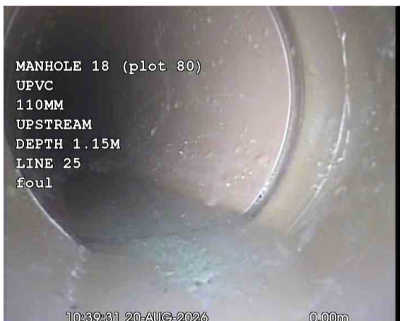
SVPX_db27abdd-764f-48a2-8db6-5257bb3fac5f_20260917_172439_531.jpg, 00:00:32, 0.00 m Start node, manhole, reference: MANHOLE 18 (MH18)
