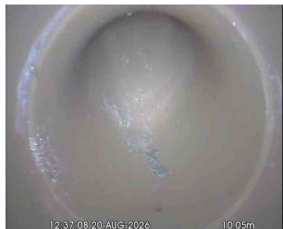
SVPX_ef59d4fd-517b-400d-a653-1d437e89bdcd_20260917_183028_478.jpg, 00:00:41, 10.05 m Line deviates up, REST BEND
