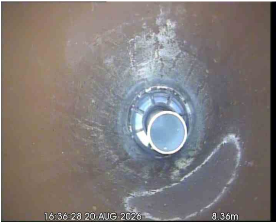
KIT. SINKX_3b50ca90-67ec-4a5c-b67b-d2a1fed15622_20260918_095015_783.jpg, 00:01:03, 8.36 m Finish node, major connection without manhole, reference: KITCHEN SINK
