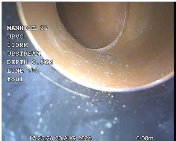
SVPX_f454dc11-7d36-4197-9d2a-7ded42e46329_20260918_102221_808.jpg, 00:00:21, 0.00 m Start node, manhole, reference: MANHOLE 37 (MH37)
