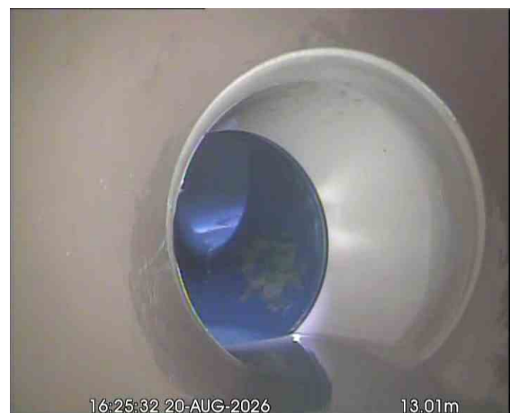
MH30X_e6dd477d-844e-49bb-8fa4-aae3ab251036_20260918_094245_330.jpg, 00:01:24, 13.01 m Line deviates left
