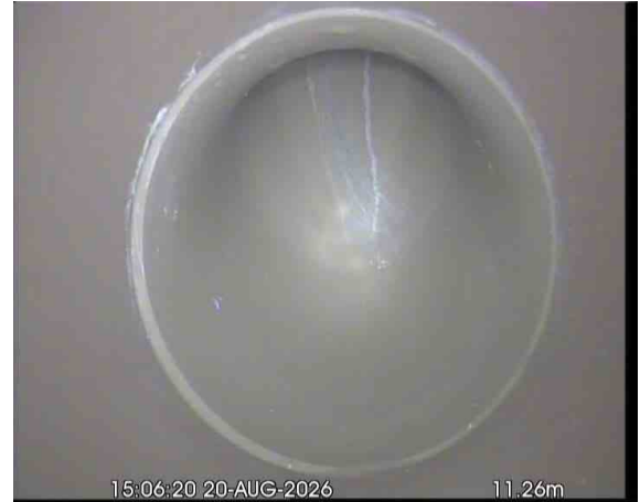
SVPX_823520d6-ebad-4206-bf54-7e7e307a5059_20260918_092357_476.jpg, 00:00:54, 11.26 m Line deviates up, REST BEND
