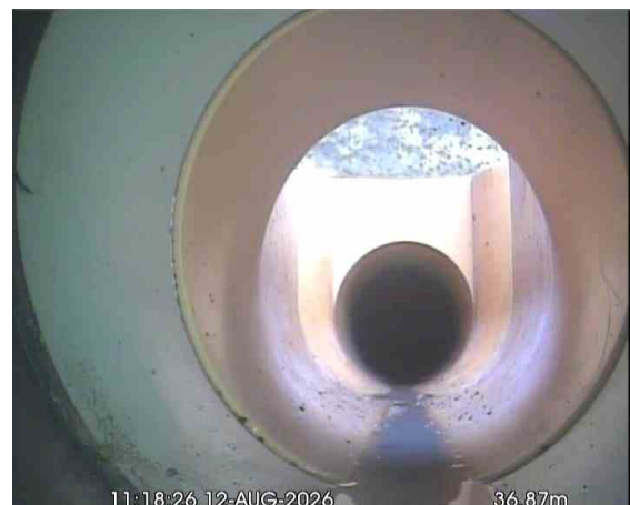
MH2 (S24)X_1f274a2c-b6c5-4dc5-a557-e1fbc41492d_20260917_160035_851.jpg, 00:05:19, 36.87 m Size changes, new size(s), 150mm high
