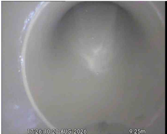
SVPX_8209400f-7154-4b0f-bf21-6b00a4c60ef7_20260918_102417_128.jpg, 00:01:04, 9.25 m Line deviates up, REST BEND
