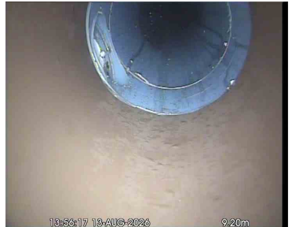
SVPX_dcc6d24c-69b0-44c0-9e6a-ca820a073452_20260917_165828_107.jpg, 00:01:14, 9.20 m Finish node, major connection without manhole, reference: SOIL VENT PIPE (SVP) & KITCHEN SINK
