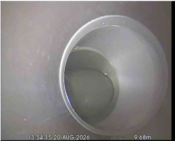
MH26X_8d97f965-42f0-4b65-abe9-5d5c172e9719_20260917_185907_550.jpg, 00:02:07, 9.68 m Line deviates left
