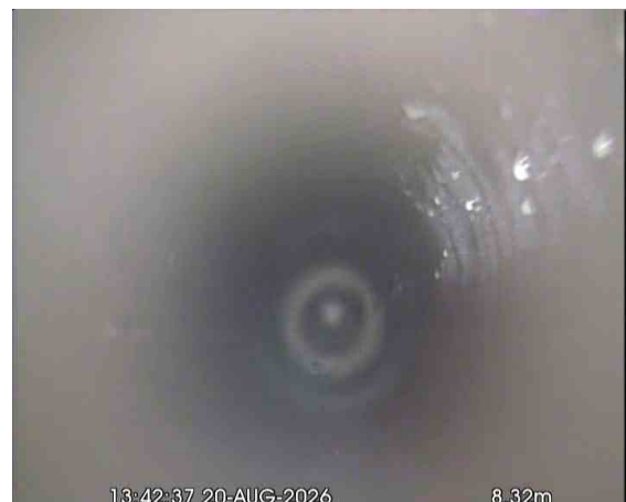
CAPPED OFFX_806f7018-b1ae-4e8c-bd13-b77898bdce52_20260917_185330_673.jpg, 00:01:28, 8.32 m Water level, 0% of the vertical dimension
