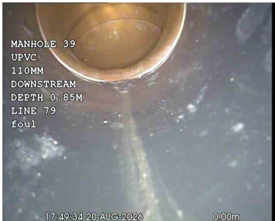
MH39X_c023d4a9-6269-49bd-b7b9-cf8accdccb14_20260918_103439_624.jpg, 00:00:23, 0.00 m Start node, manhole, reference: MANHOLE 39 (MH39)
