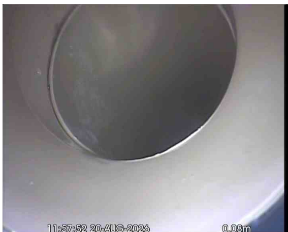
MH21X_bfb0d036-24df-40eb-af21-87cb0f3fa57b_20260917_182120_268.jpg, 00:00:27, 0.08 m Line deviates down
