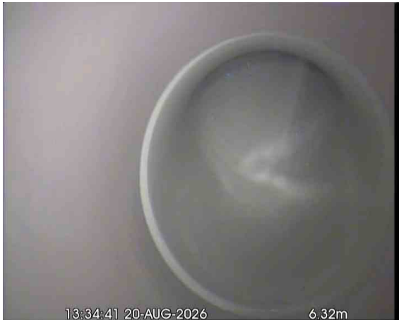
UTIL. SINKX_a5ffe22-e254-4a21-9083-55167c9d769c_20260917_184857_865.jpg, 00:00:42, 6.32 m Line deviates up, REST BEND
