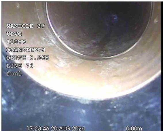
MH37X_38ed49cf-08e8-4ce0-8b34-251c6df5da31_20260918_102743_618.jpg, 00:00:18, 0.00 m Start node, manhole, reference: MANHOLE 37 (MH37)
