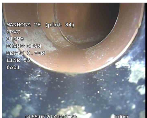
MH28X_b06b7e3b-e5d9-4086-85d1-04627a22dca0_20260918_091126_429.jpg, 00:00:20, 0.00 m Start node, manhole, reference: MANHOLE 28 (MH28)
