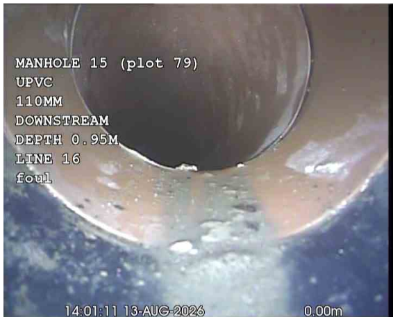
MH15X_63ecdd8e-6071-4a89-9ccf-77f62818ab1b_20260917_170120_156.jpg, 00:00:23, 0.00 m Start node, manhole, reference: MANHOLE 15 (MH15)
