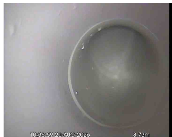
SVPX_b62ef229-8eab-40e3-aeda-763403b412c2_20260917_172320_991.jpg, 00:01:07, 8.73 m Line deviates up, REST BEND
