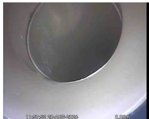
MH21X_2fe4941a-fc44-4b64-8983-a82f4c9ab2ab_20260917_182114_094.jpg, 00:00:27, 0.08 m Line deviates right
