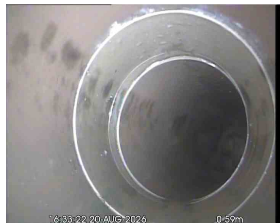
MH31X_d7c9df2d-077d-4a44-8e79-5a2920e7fa12_20260918_094722_462.jpg, 00:00:25, 0.59 m Line deviates right
