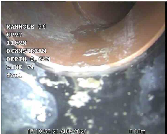
MH36X_7ff1463f-c8ca-476a-99e8-fccbf27363c_20260918_102031_515.jpg, 00:00:39, 0.00 m Start node, manhole, reference: MANHOLE 36 (MH36)
