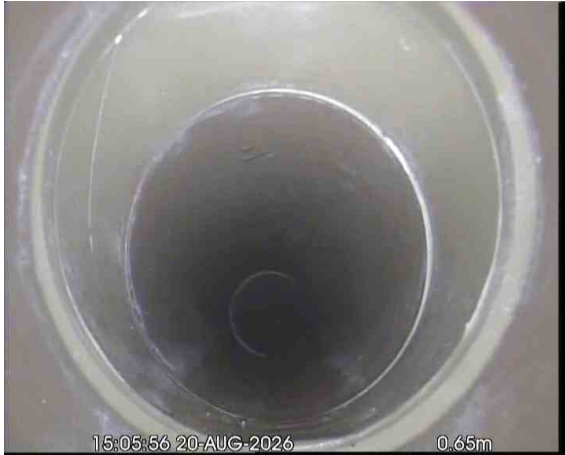
SVPX_6d52c3d2-25f5-451d-96f2-1c7d6744fab8_20260918_092336_423.jpg, 00:00:30, 0.65 m Line deviates down
