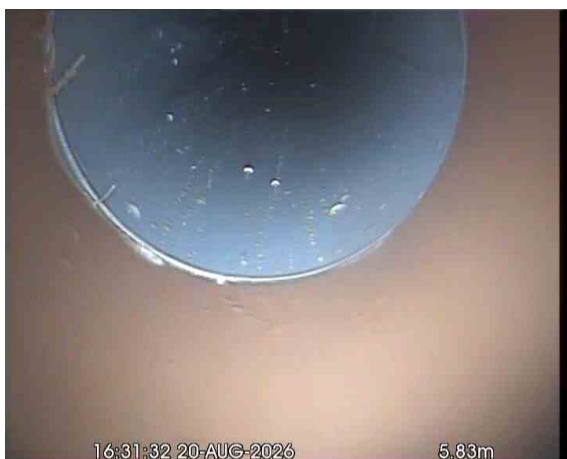
SVPX_338a2e6e-6e3d-45c7-8b63-0cd4e1440a49_20260918_094551_984.jpg, 00:01:36, 5.83 m Finish node, major connection without manhole, reference: SOIL VENT PIPE (SVP)
