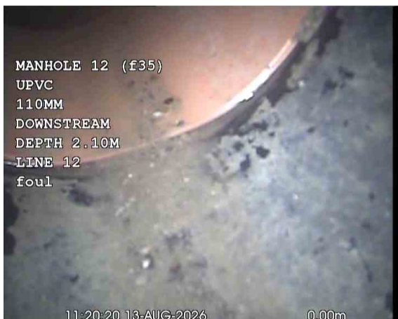
MH12 (F35)X_65c4e705-f367-41ad-a17c-f5910dea6bd0_20260917_165107_059.jpg, 00:00:50, 0.00 m Start node, manhole, reference: MANHOLE 12 (MH12), (F35)
