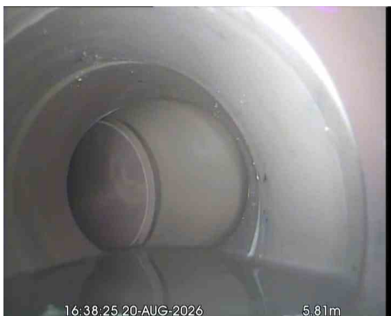
MH32X_dfc88d4f-44ce-4566-b4c4-49e10635f7a6_20260918_095245_591.jpg, 00:00:52, 5.81 m Water level, 10% of the vertical dimension
