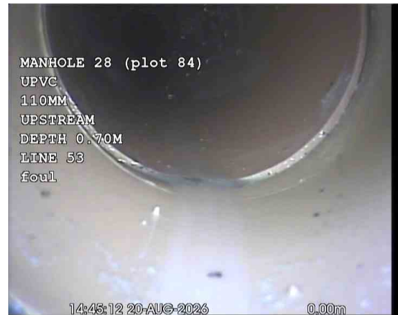
CAPPED OFFX_338b7339-8fc5-47ef-8607-58f75723d100_20260918_0 90625_104.jpg, 00:00:30, 0.00 m Water level, 0% of the vertical dimension
