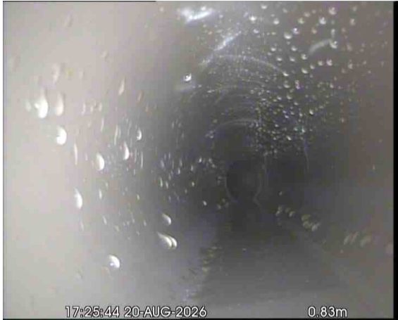
SVPX_c82a844d-0596-42db-a9f1-8bf3dbabeedd_20260918_102312_479.jpg, 00:00:38, 0.83 m Water level, 5% of the vertical dimension
