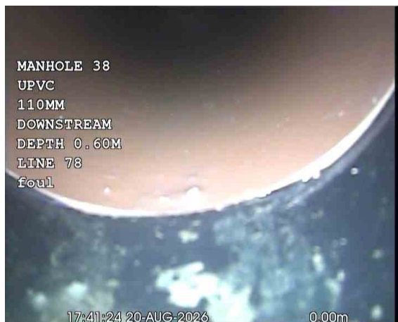
MH38X_36e04c52-039b-44b7-b53c-852b41b8c2c5_20260918_103210_214.jpg, 00:00:20, 0.00 m Start node, manhole, reference: MANHOLE 38 (MH38)
