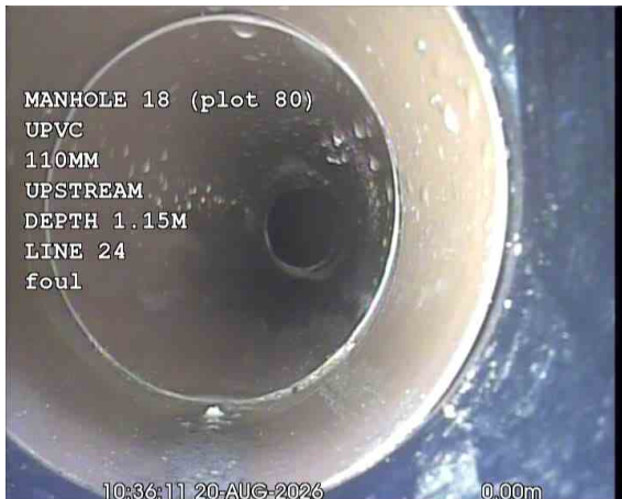
SVPX_e468887e-16f8-418e-80c7-2ed563686ce8_20260917_172235_349.jpg, 00:00:19, 0.00 m Start node, manhole, reference: MANHOLE 18 (MH18)
