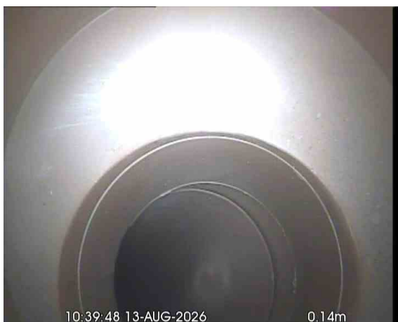
MH10 (F33)X_611c9cc4-c847-4f8c-be2e-970db7baba0f_20260917_162752_448.jpg, 00:01:50, 0.14 m Size changes, new size(s), 110mm high
