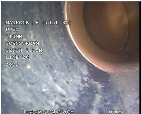
MH18X_99746b94-685d-4e1b-b362-86349ff1a78e_20260917_172625_060.jpg, 00:00:21, 0.00 m Start node, manhole, reference: MANHOLE 18 (MH18)
