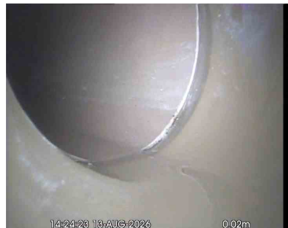
SVPX_65cf9813-f4ed-4a7c-a7f3-61bf8bdc7fbf_20260917_171245_884.jpg, 00:00:39, 0.02 m Line deviates left
