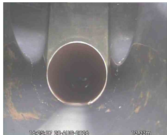
MH30X_de6d7b5e-1df0-4526-8621-0321ea6a95d2_20260918_094311_999.jpg, 00:01:29, 13.33 m Finish node, manhole, reference: MANHOLE 33 (MH33)
