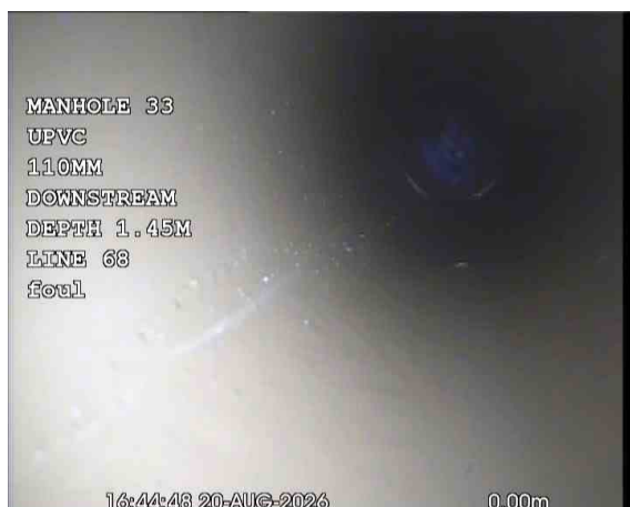
MH33X_42e53fca-b86e-4afe-b49b-3d8e4b965fed_20260918_095450_404.jpg, 00:00:25, 0.00 m Start node, manhole, reference: MANHOLE 33 (MH33)
