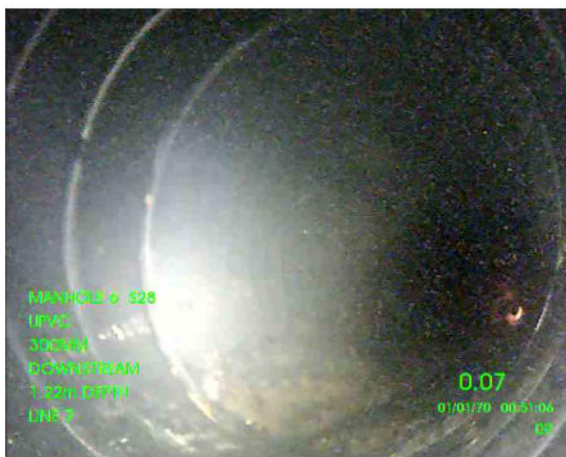
MH6 (S28)X_0572d9ae-b482-4f06-ad13-5a0d335b5bf1_20260917_161445.png, 0.07 m Line deviates right
