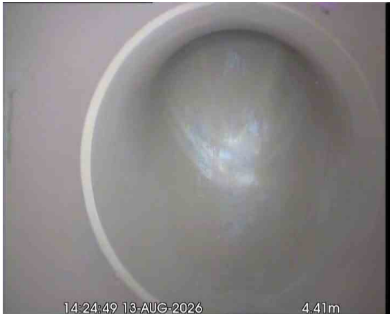
SVPX_20acf176-d350-4499-b5e7-33c17b2036cd_20260917_171310_629.jpg, 00:01:04, 4.41 m Line deviates up, REST BEND
