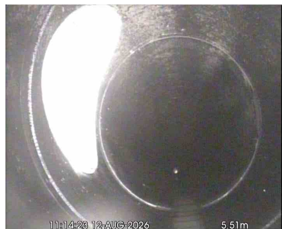
MH2 (S24)X_b5ecb4c4-0c32-4ed7-8a51-b194671de47a_20260917_155727_905.jpg, 00:01:16, 5.51 m Junction at 9 o'clock, diameter: 150mm
