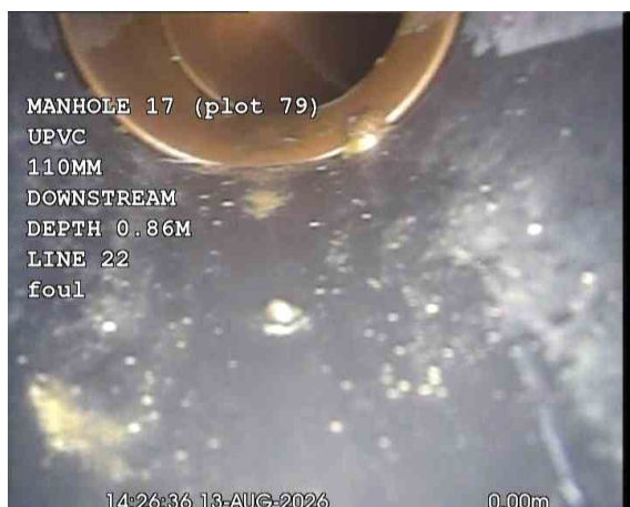
MH17X_44199b25-50d9-4700-891f-b23154a8e130_20260917_171426_034.jpg, 00:00:24, 0.00 m Start node, manhole, reference: MANHOLE 17 (MH17)
