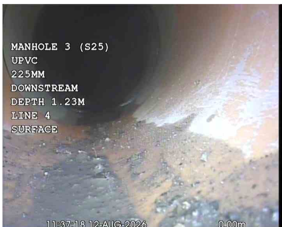
MH3 (S25)X_bc5ddc7d-f27a-4e64-b99e-2df88dd07134_20260917_160242_868.jpg, 00:01:09, 0.00 m Start node, manhole, reference: MANHOLE 3 (MH3), (S25)
