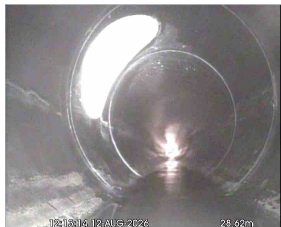
MH5 (S26)X_3a3654d2-9b1b-4e04-9694-8c7e2273311f_20260917_160559_119.jpg, 00:04:51, 28.62 m Water level, 5% of the vertical dimension
