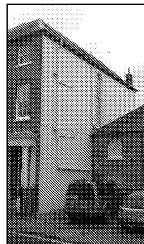
The west wall of Carleton House, from the north-west.
