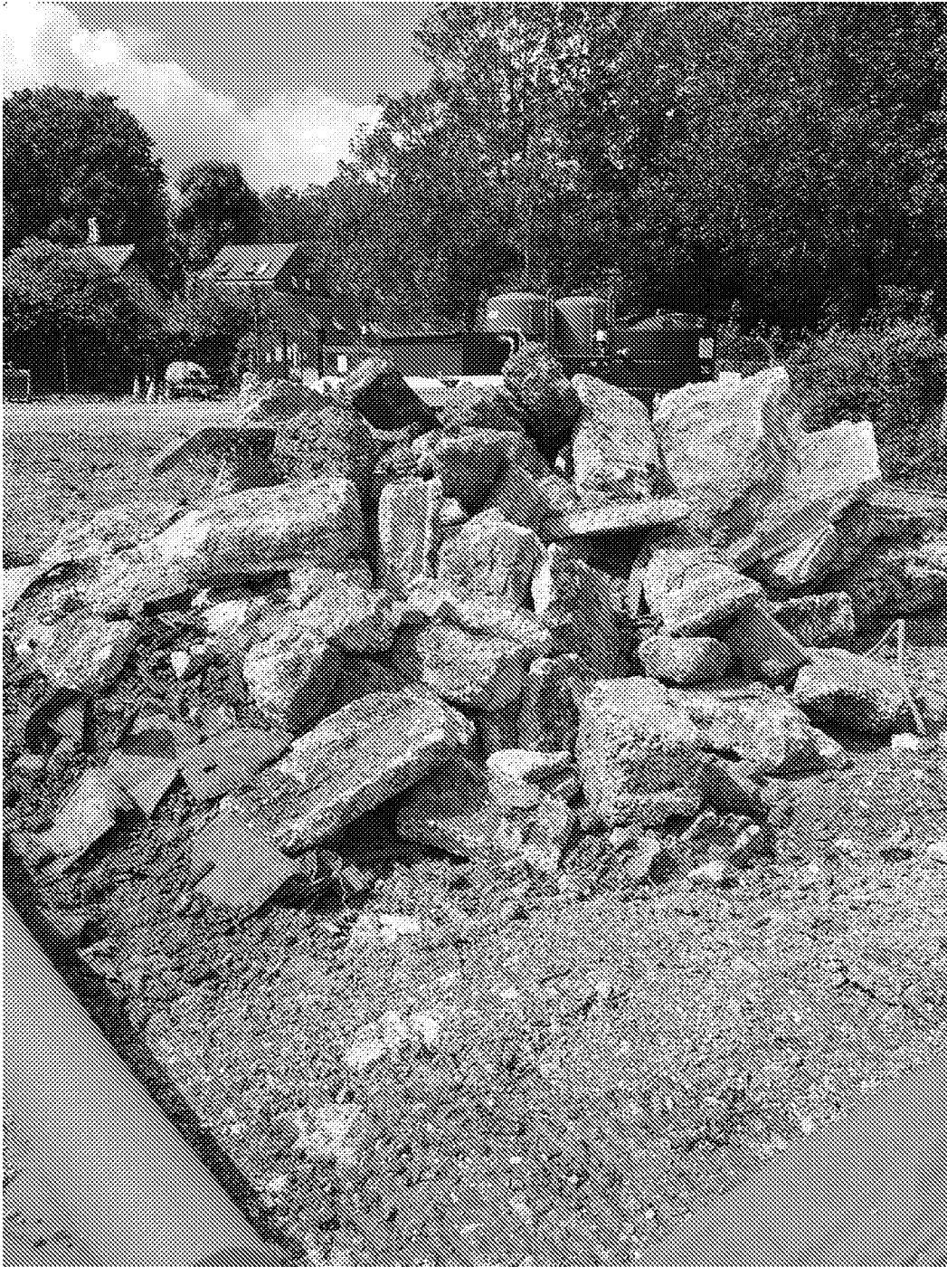
Plate 52 – Further concrete obstructions removed from Area 4
