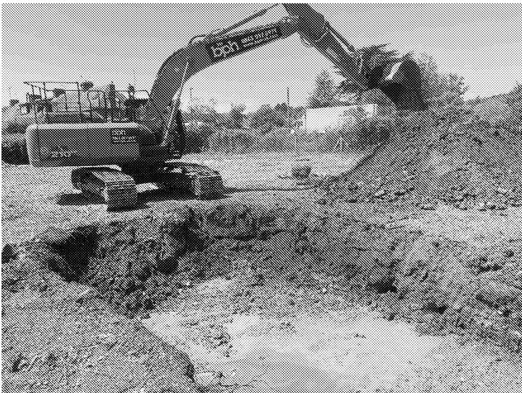
Plate 6 – Excavation of F4 in readiness for water treatment system area
