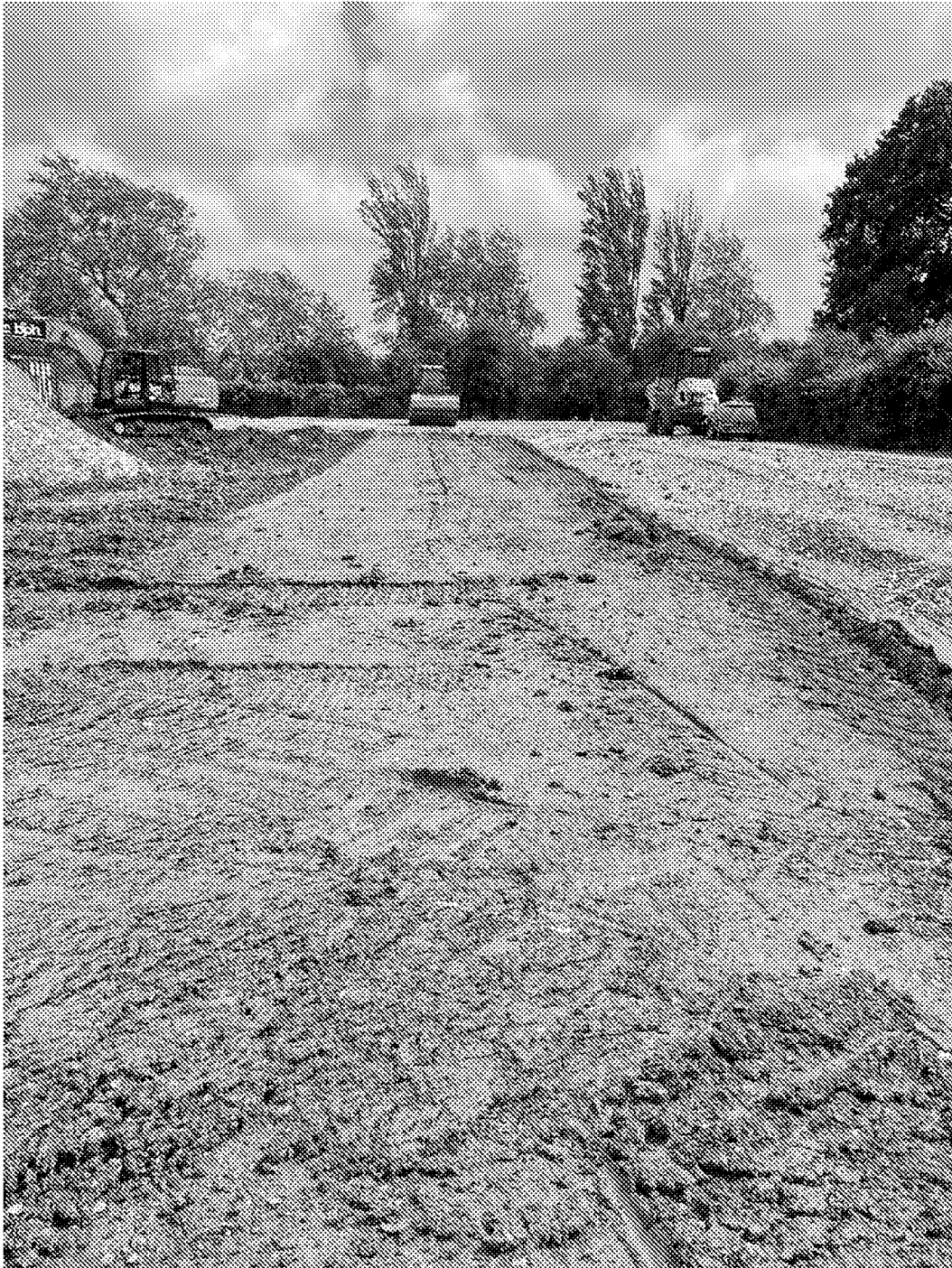
Plate 34 – Re-compacting made ground across Area 3
