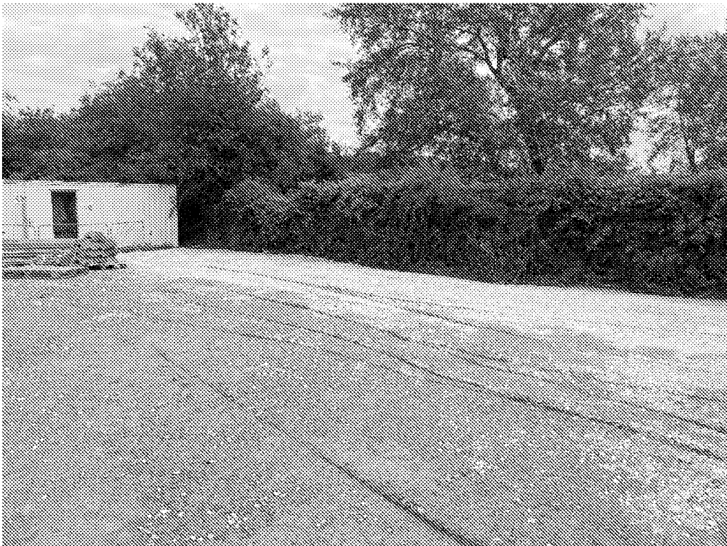
Plate 25 – Capping layer placed across Area 1
