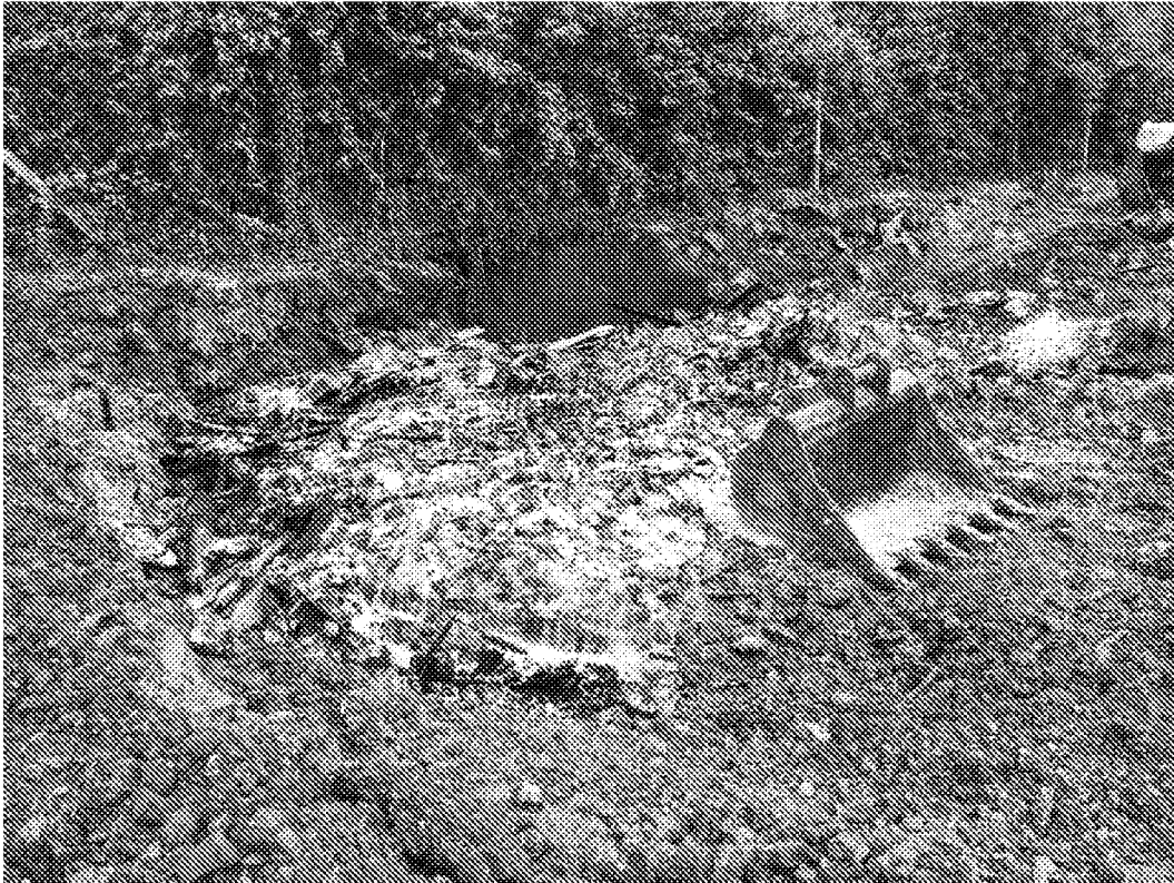
Plate 37 – Contaminated materials within former gasholder (feature no. 4)
