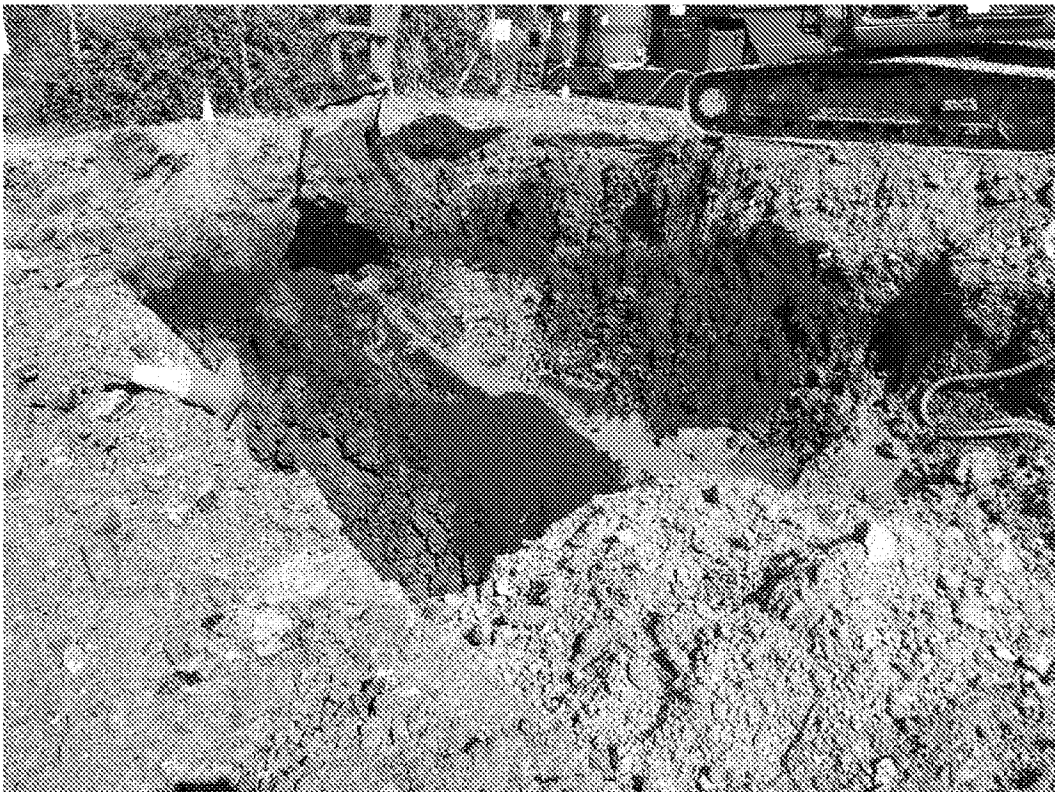
Plate 43 – Addition of PFA and cement grout to contaminated materials in grid E2
