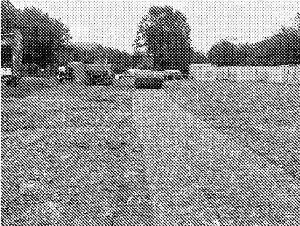
Plate 25 – Capping layer placed across Area 1
