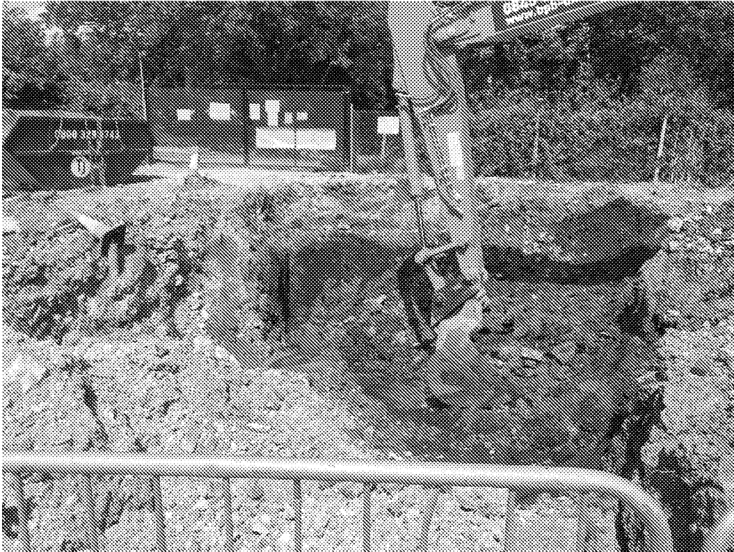
Plate 43 – Addition of PFA and cement grout to contaminated materials in grid E2
