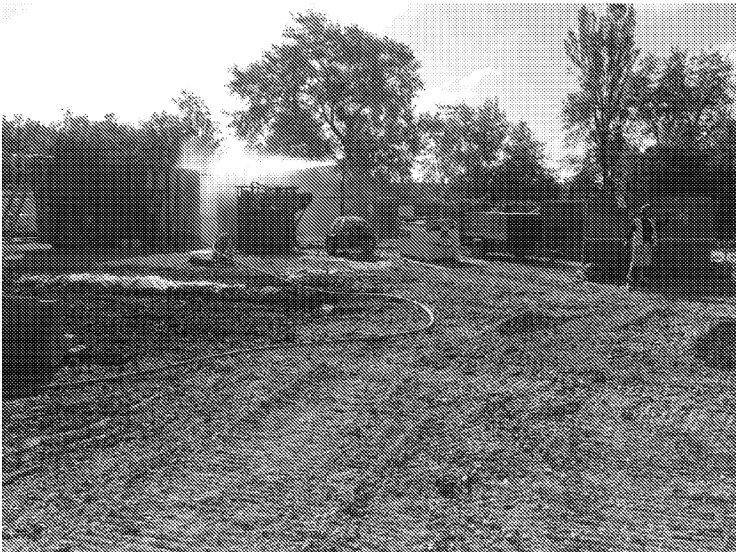
Plate 49 – Grout mixing area with water mist sprayer to dampen potential dust emissions
