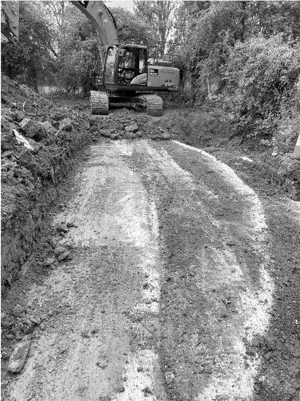
Plate 21 – Exposing the gas holder base across grid A7
