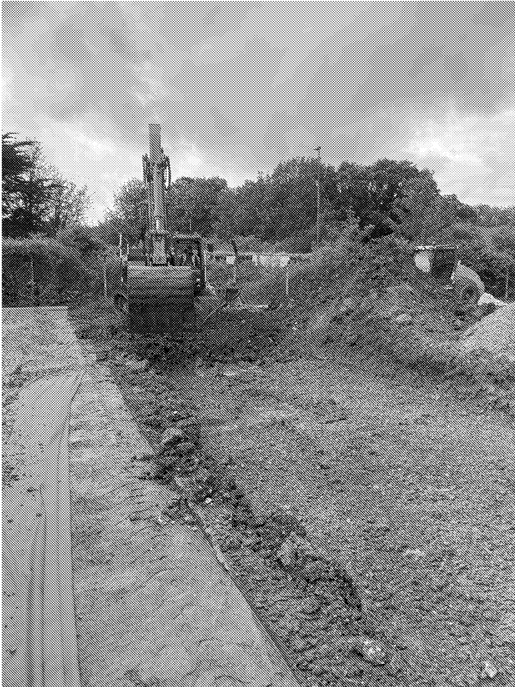
Plate 33 – Excavation to natural ground in grid C1 / C2
