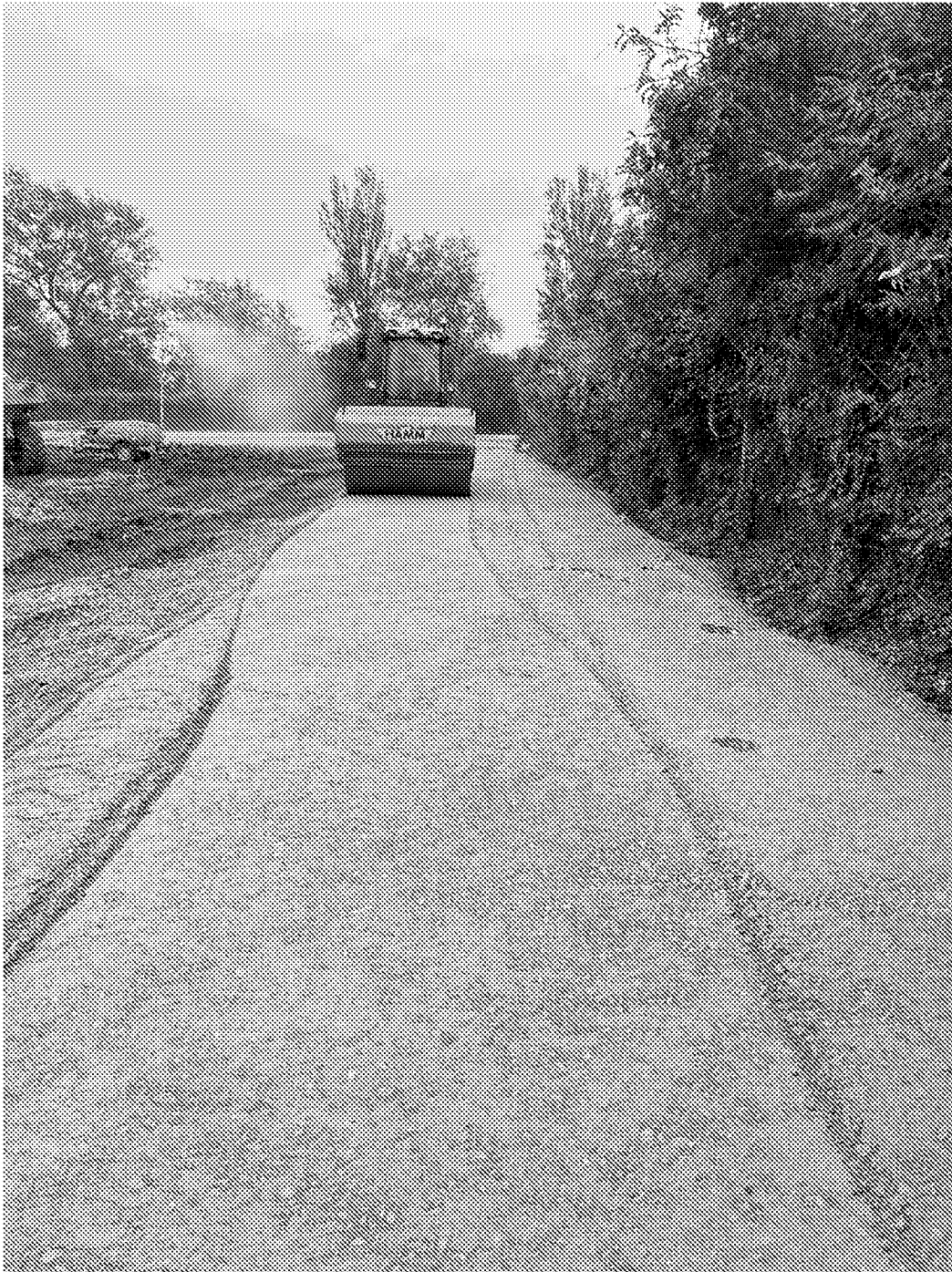
Plate 28 – Capping layer placed across Area 2
