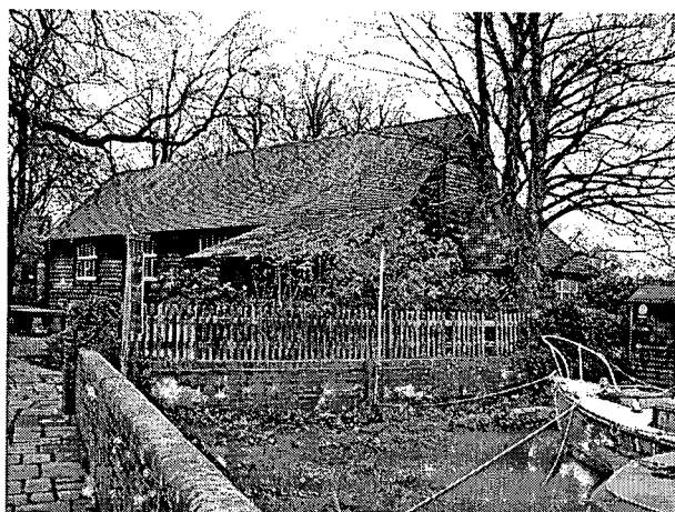
Existing Hall – View from the River
