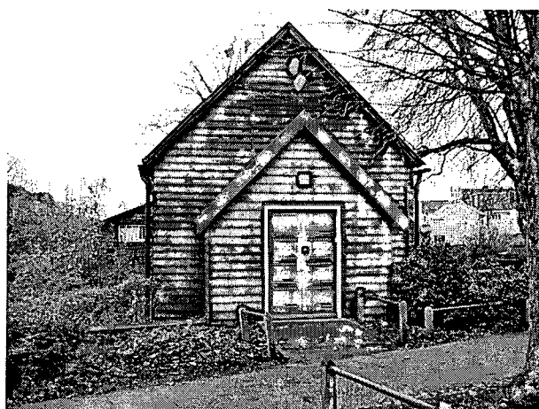
Existing Hall – Main Entrance
