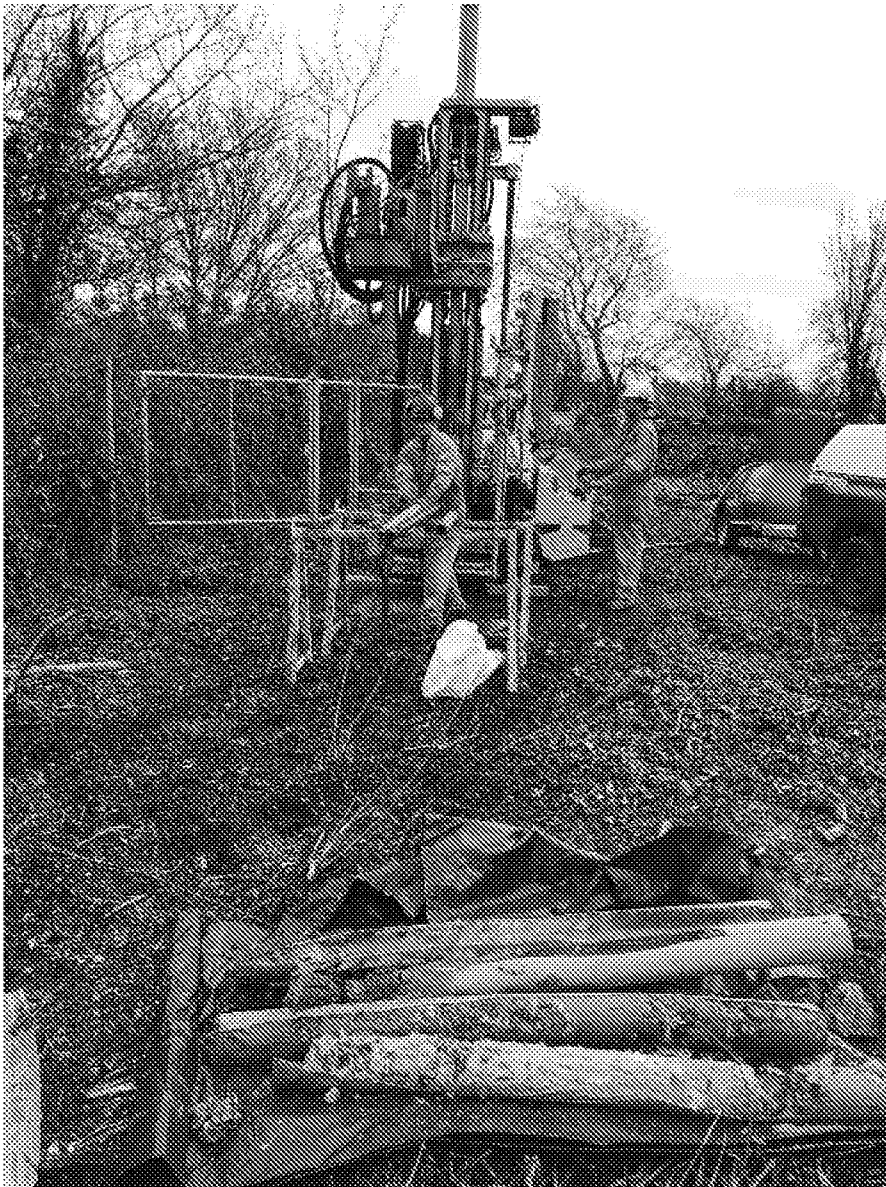
Plate 44 Borehole BH201 during drilling
