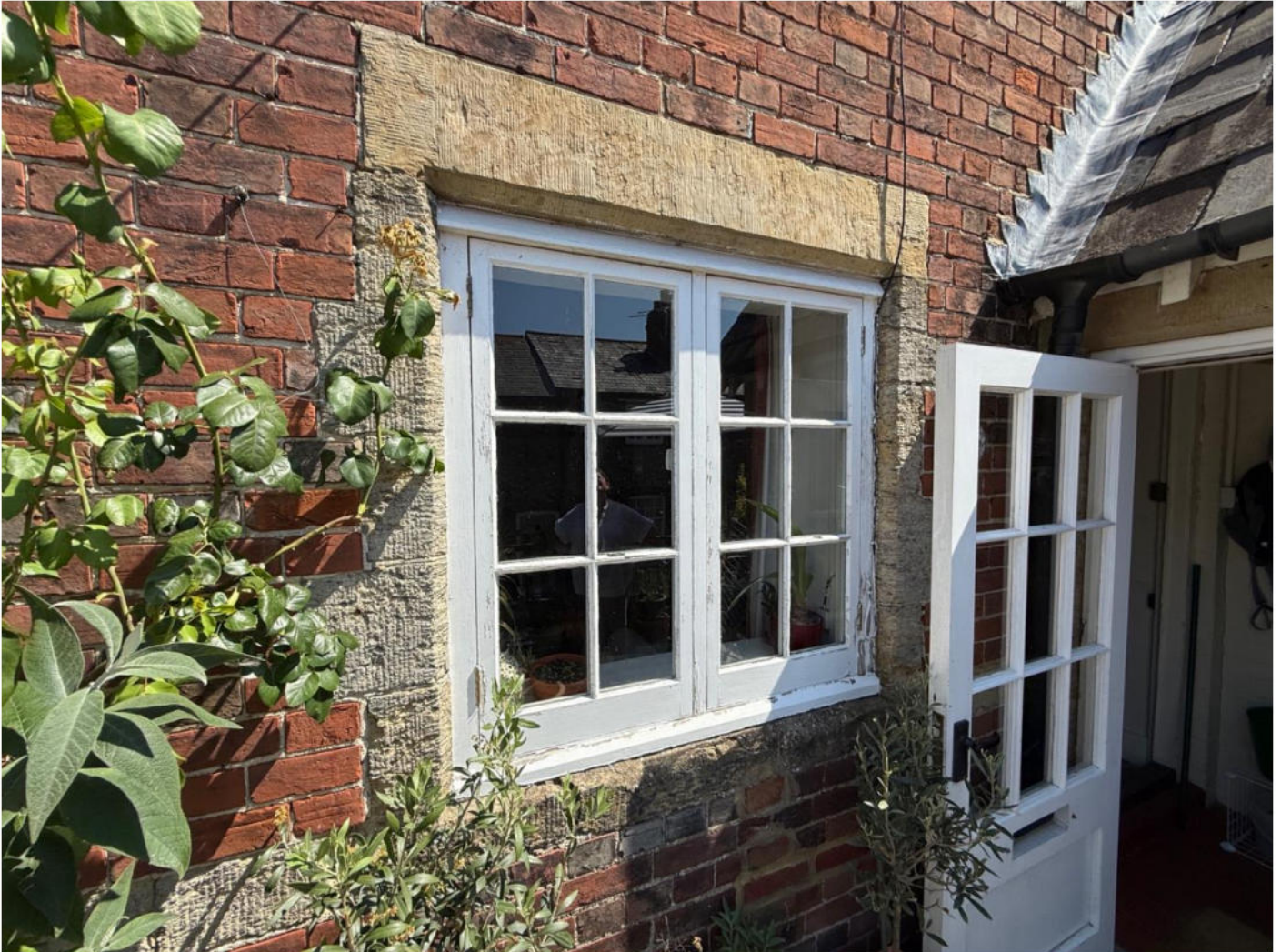
Ground floor front window and entrance door
