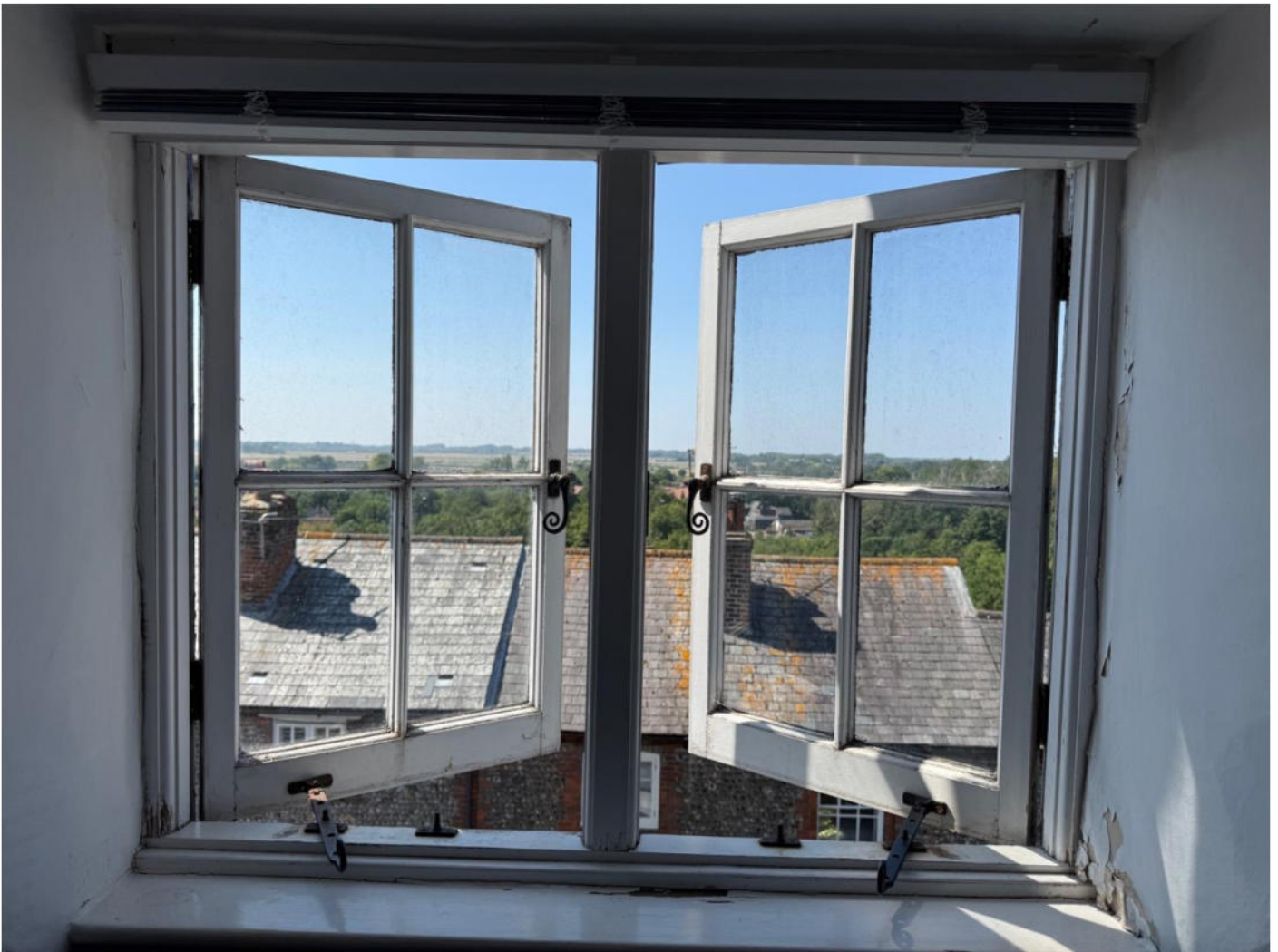
Existing front dormer window (internal)
