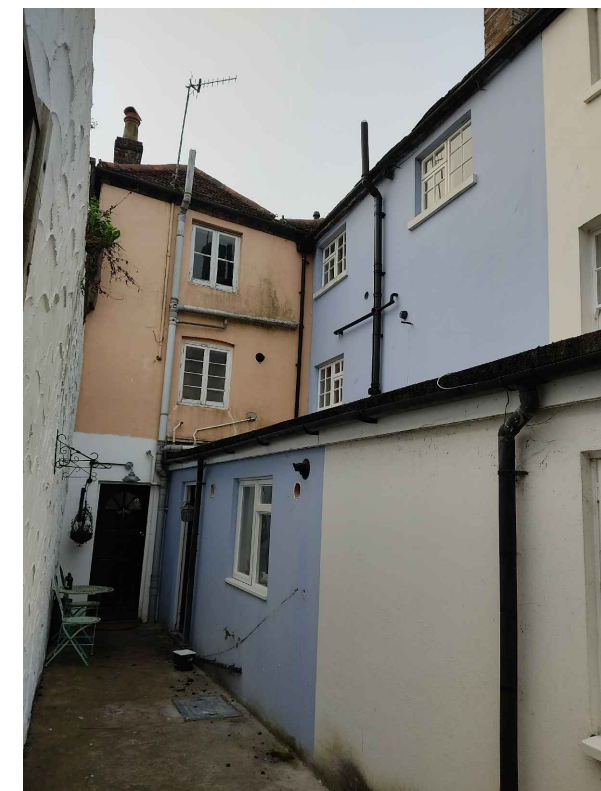
PHOTOGRAPH: REAR ELEVATION
