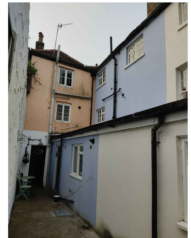
PHOTOGRAPH: REAR ELEVATION
