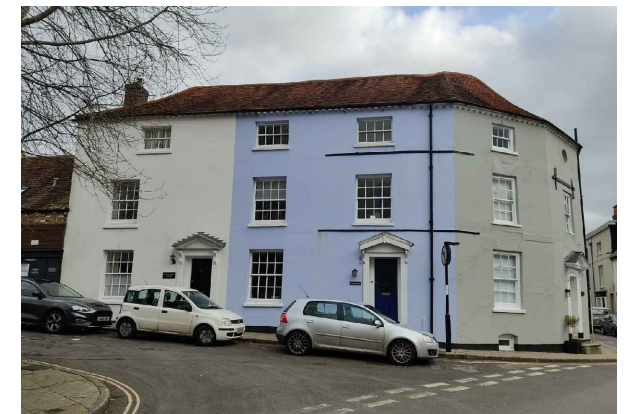
PHOTOGRAPH: FRONT ELEVATION
