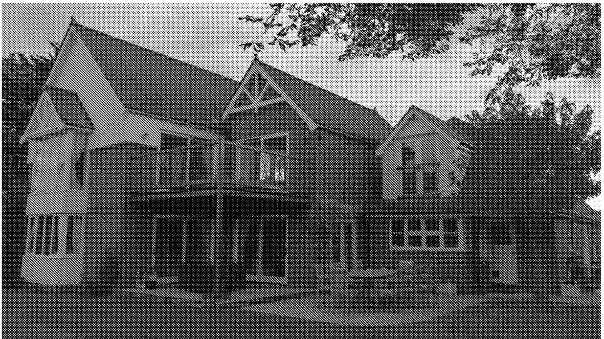
Photograph 3. Rear (North-West) elevation.
