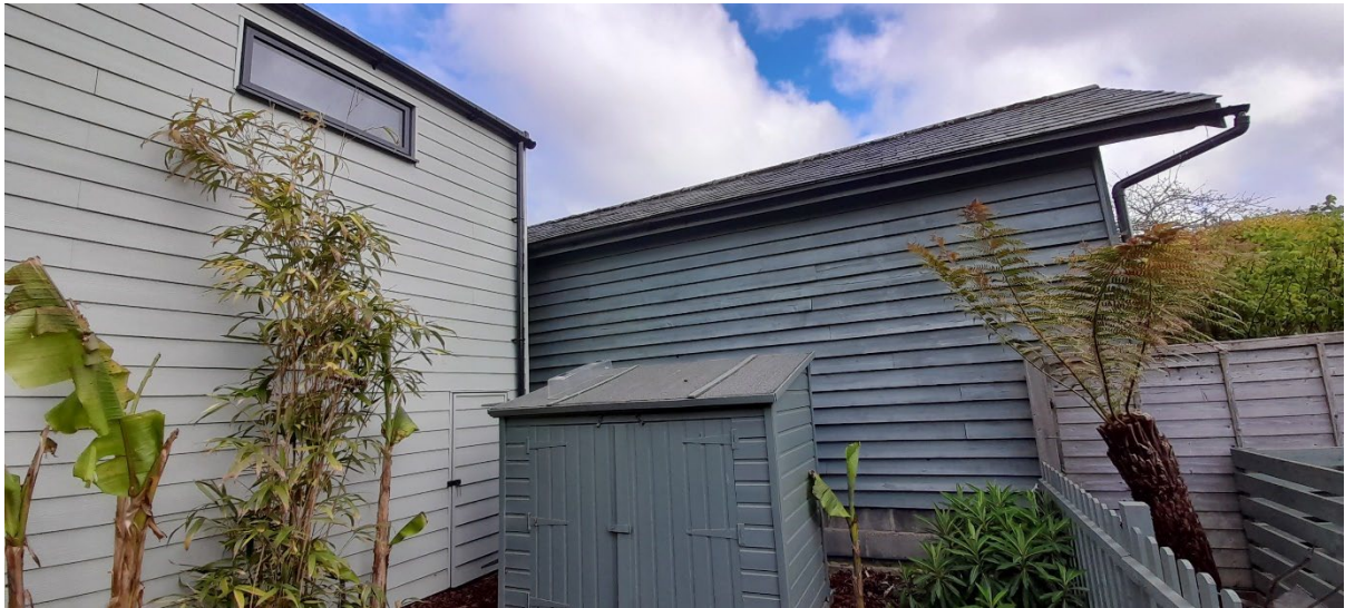
Further photo detailing the depth of the neighbouring structure in comparison to the summerhouse (shown on the left of the photo).
