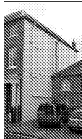
The west wall of Carleton House, from the north-west.
