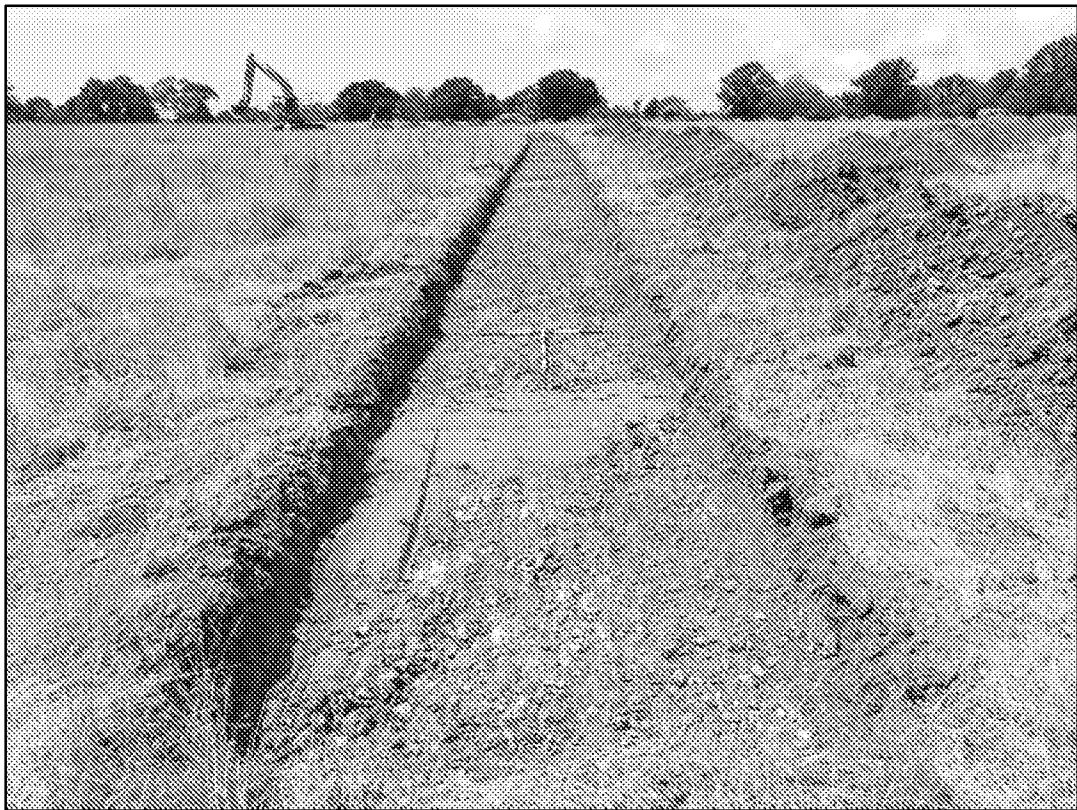
Plate 44: Area 2, Trench 24. View to southwest, 2x 1m Scale.
