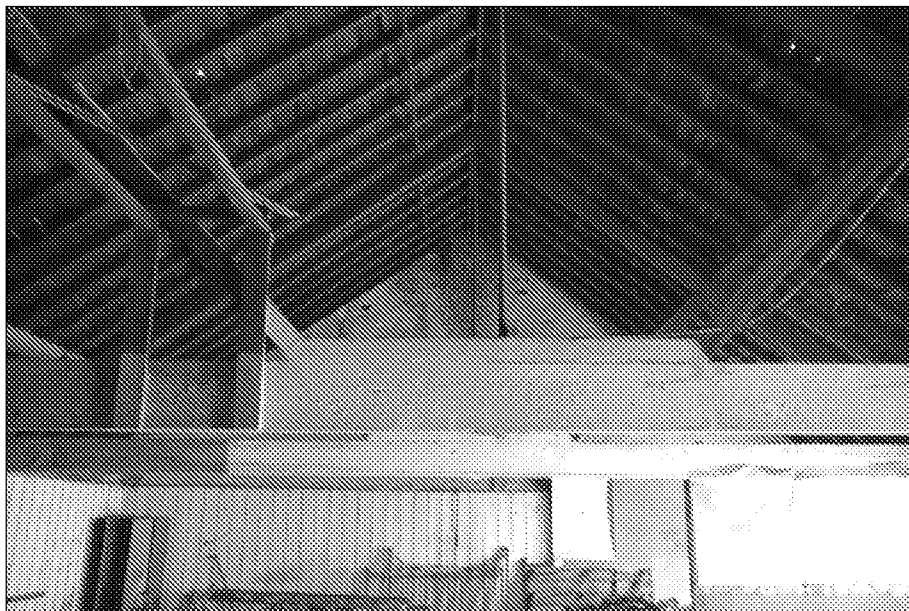
Figure 26: Original timber tie beams and metal king posts, albeit with additional timber framing applied for additional support and likely to house machinery. This is considered a typical roof structure from the late nineteenth century.
