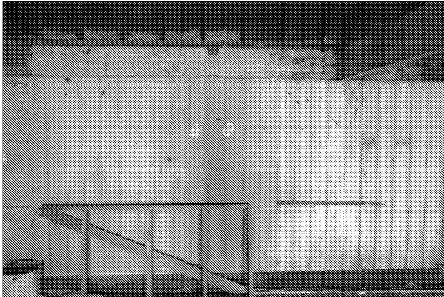
Figure 28: Typical vertical timber wide board panelling along west wall.
