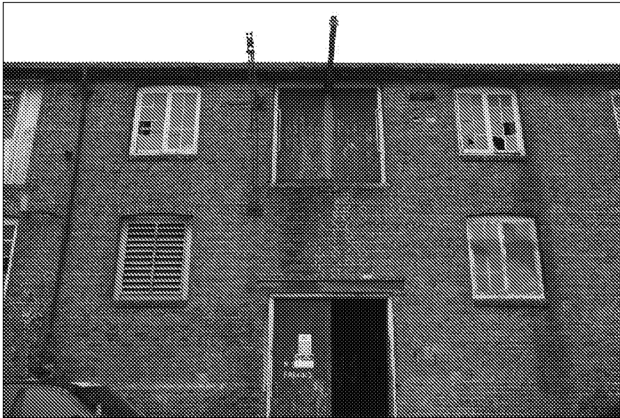
Figure 14: View looking west towards central bay of two-storey range where the main double-leaf door at ground floor and double-leaf loading bay at first floor exist.
