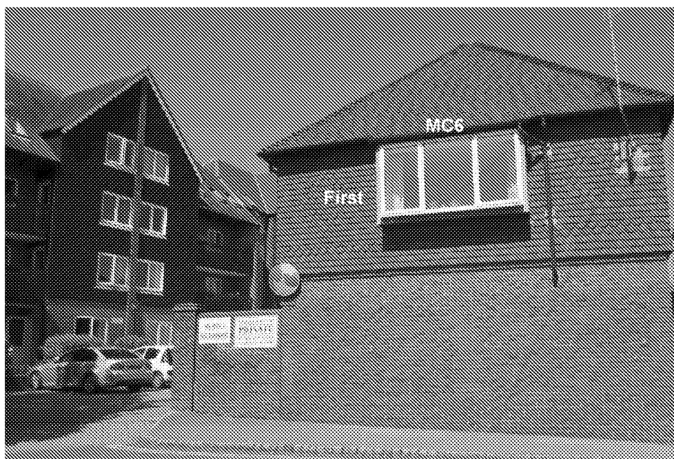
Figure 5: Window analysed to separate building at Martlets Court
