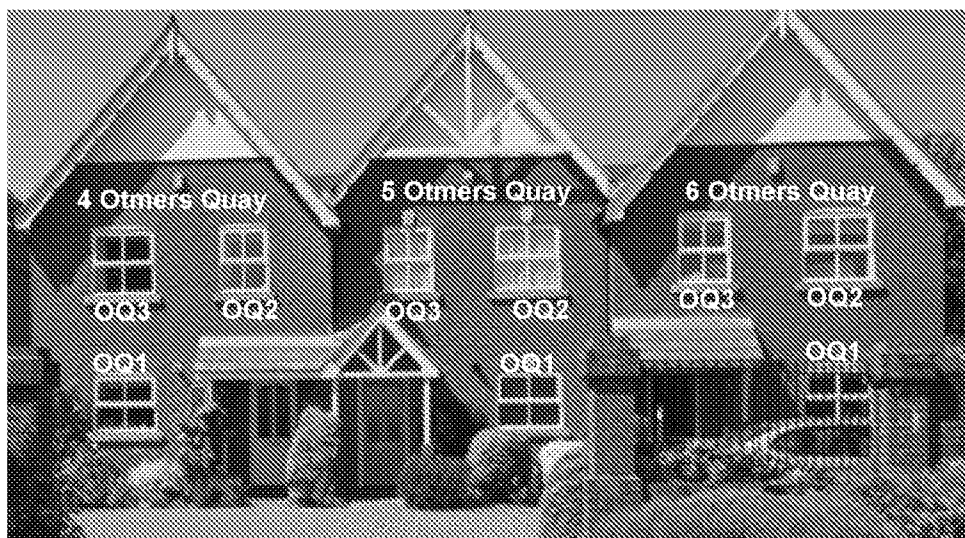
Figure 2: Layout of windows analysed at 4 - 6 Otters Quay, as seen from the development site. The window arrangement is the same at 1 - 3 Otters Quay.
