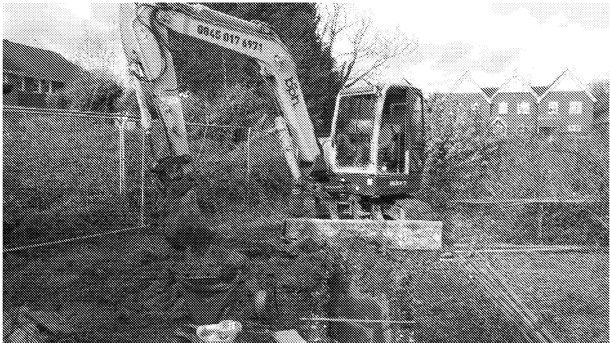
PLATE 1: 8ton Rubber Tracked Machine used for trial pitting.
