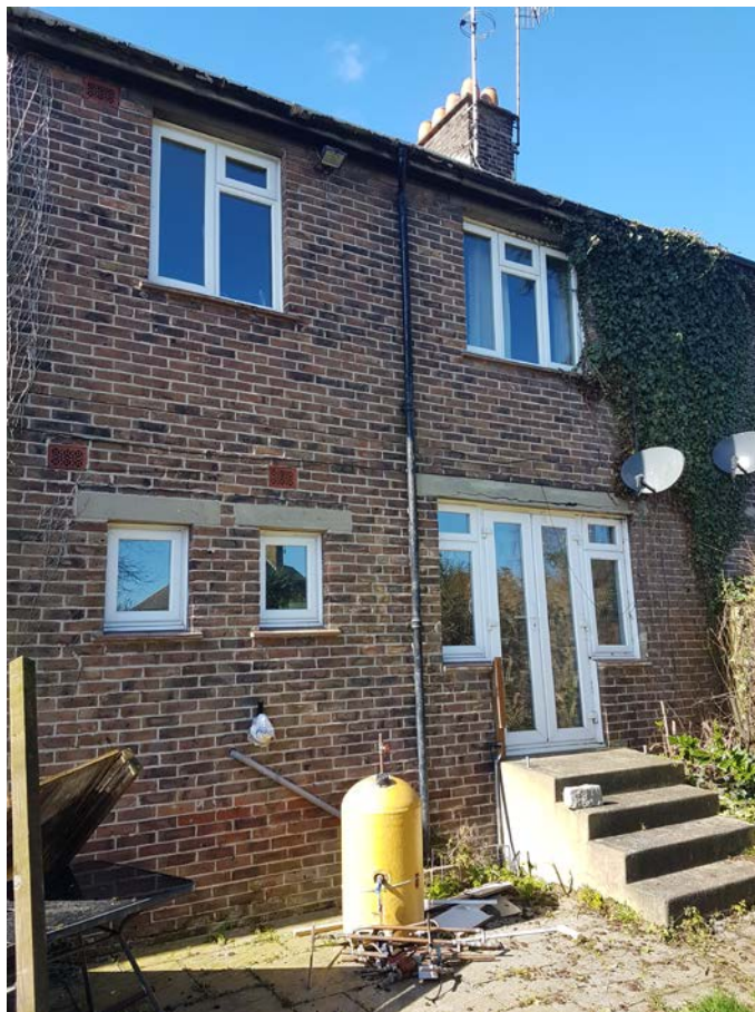
3: View of rear (North East) of property
