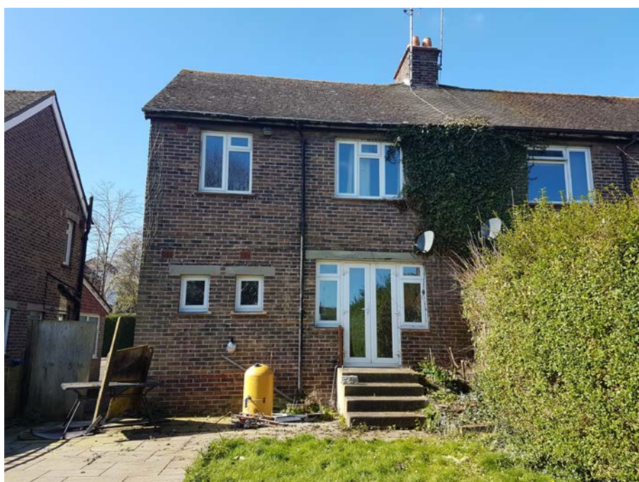
4. View of rear (North East) of property
