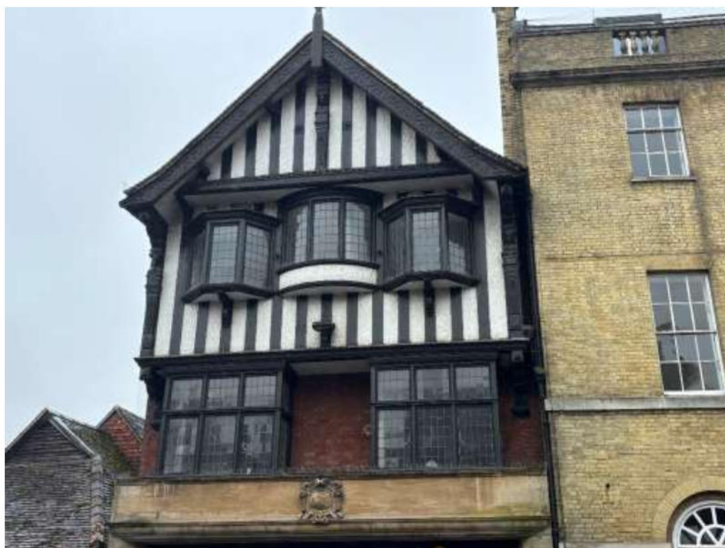
Existing upper floors to 53 High Street Arundel
