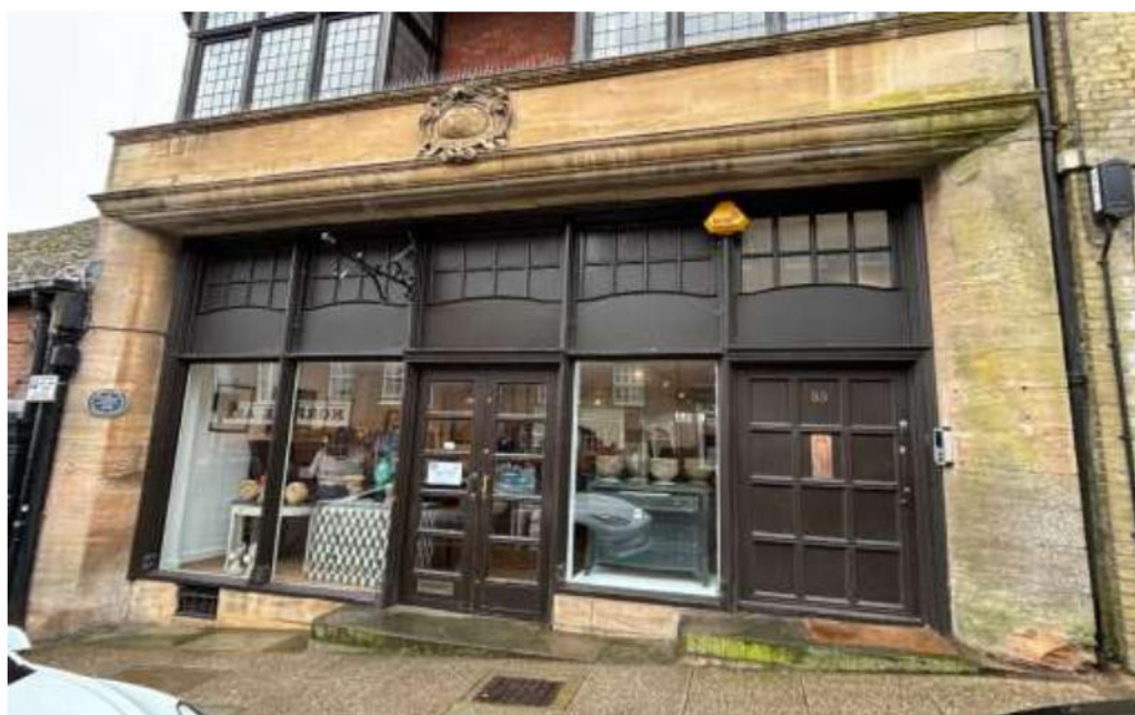
Existing ground floor shopfront 53 High Street Arundel
