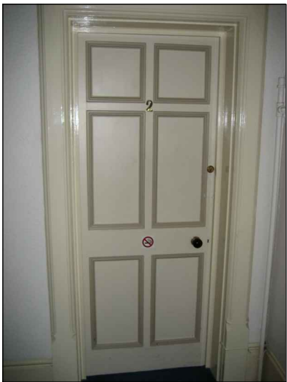
Existing Bedroom 2 6-panel Door.
