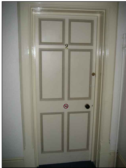
Existing Bedroom 2 6-panel Door.
