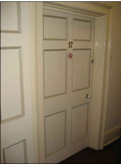
Existing Bedroom 17 6-panel Door.
