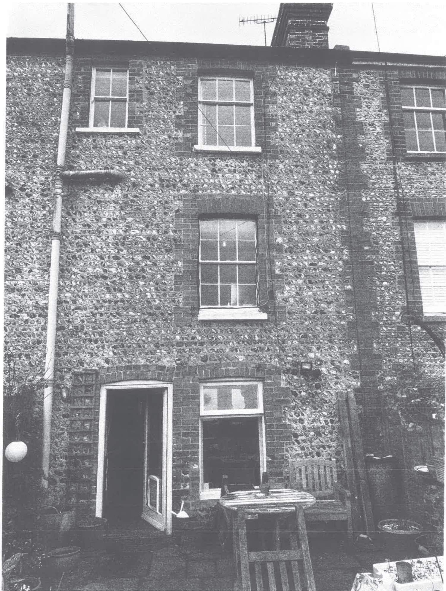
Rear - 1st floor window (replacement)
