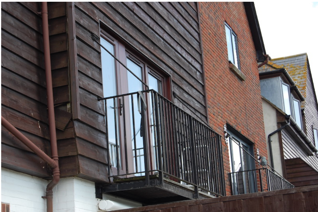
figure 1 Balcony to flat 3
