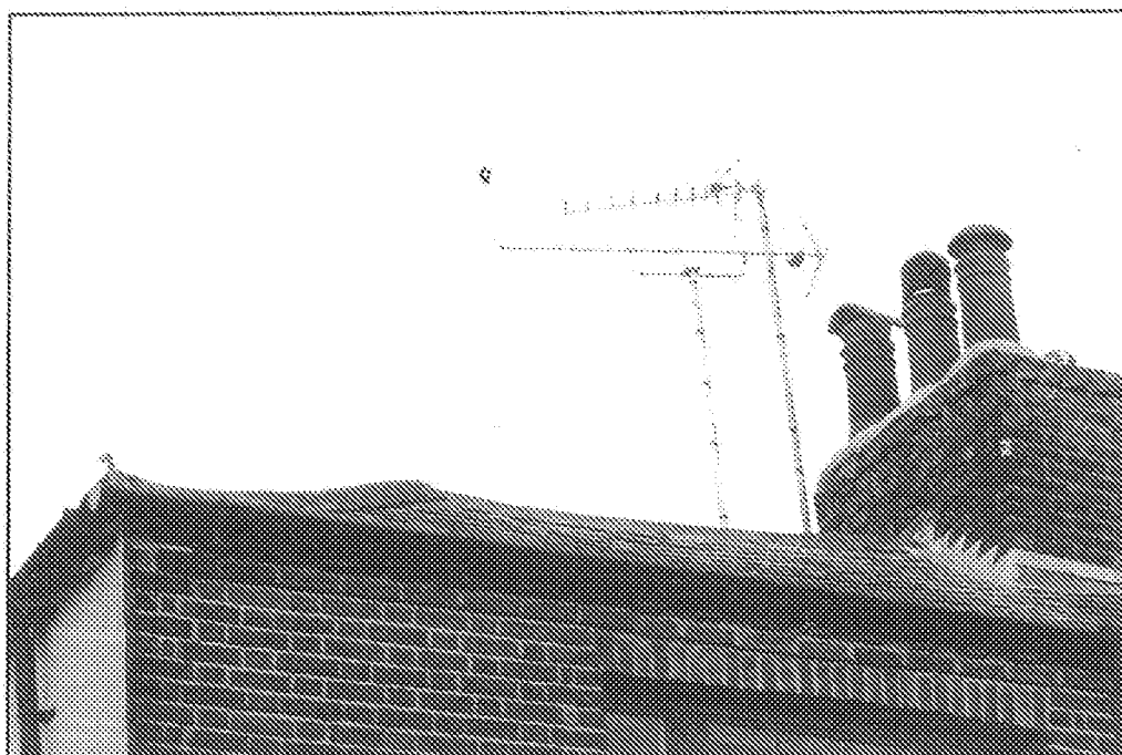
Undulating roof coverings
