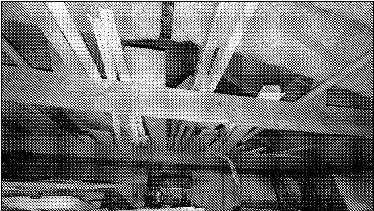
Photo 7 – Photo showing inside of the garage.
