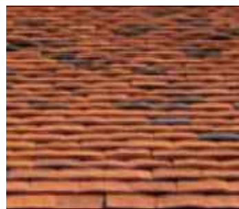
Clay Tile Roof
