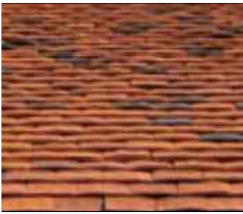
Clay Tile Roof
