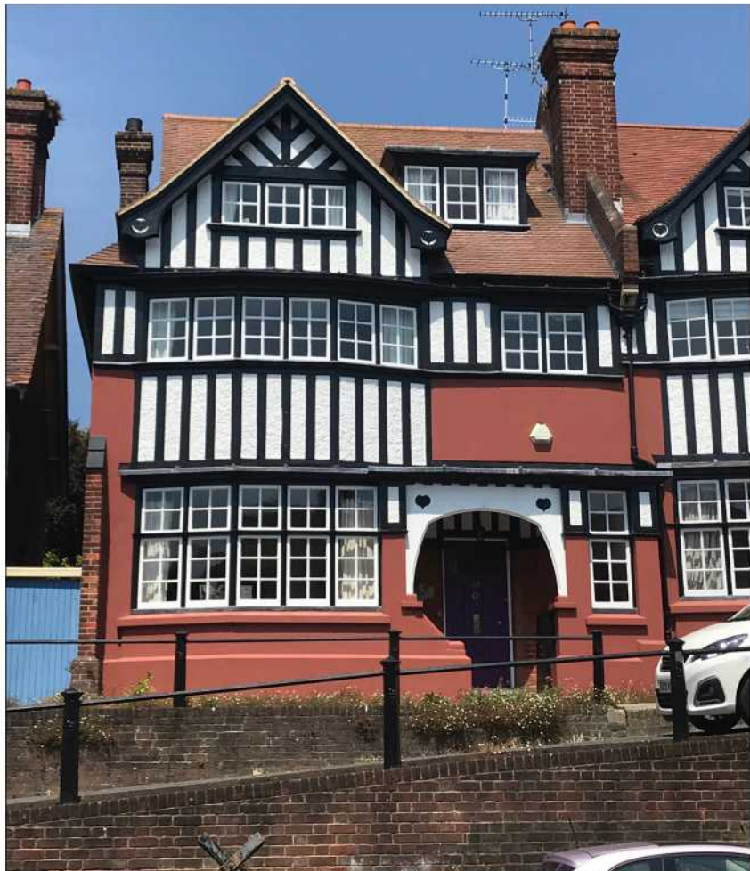
existing photographic view of front elevation of No 32 Maltravers Street
