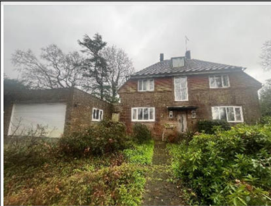
Front elevation of 37 Torton Hill Road. Single storey flat roofed garage with parapet roof. Mature front garden. Front elevation with upper 50% hanging tiles and dormer in the roof.
