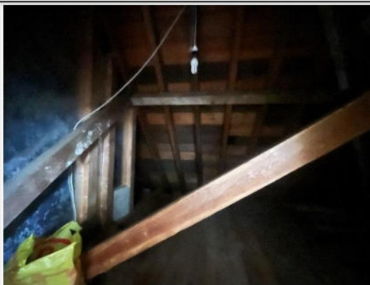
Loft space that wraps around the central bedroom in the main roof. Lined with wooden sarking boards.
