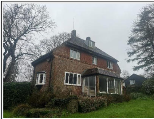
Rear elevation of the house showing the single storey conservatory/sunroom with a mansard roof (part flat/part sloped). Surrounding vegetation is mown lawn and small amounts of low ornamental scrub and creeper.
