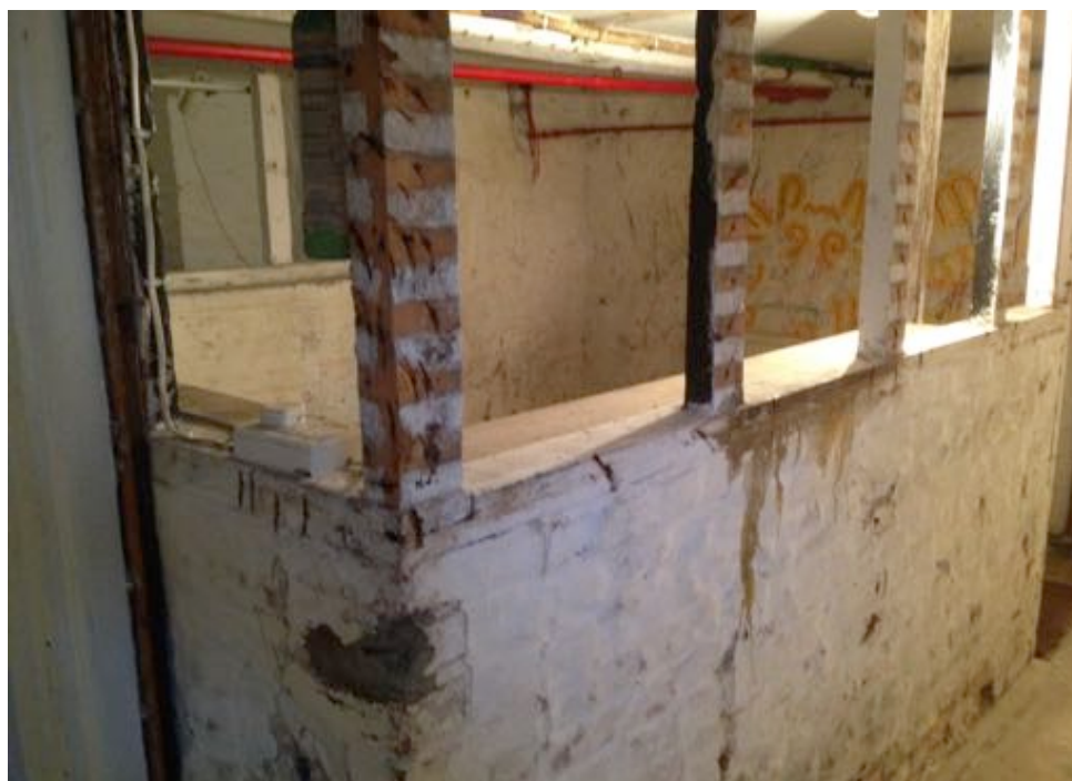
Internal wall to be removed
