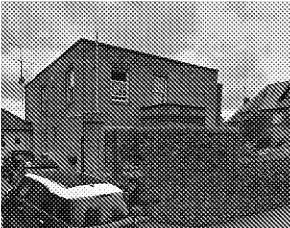
Figure 3: Existing main elevation as seen from London Road
