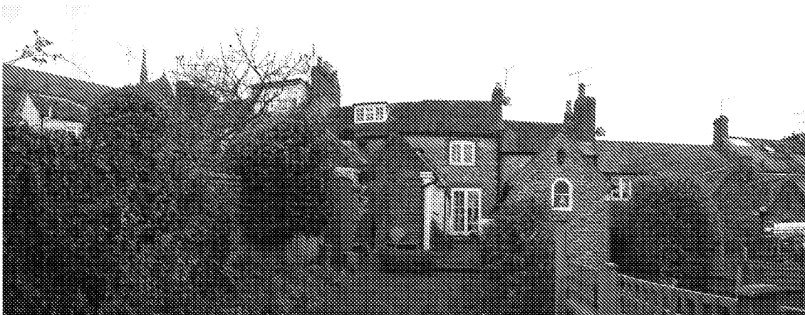
Panoramic rear elevation (no.37 to centre of picture)
