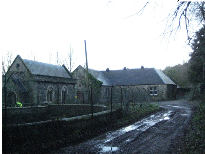
Plate 2 The Farm Buildings and Pump House from the North
