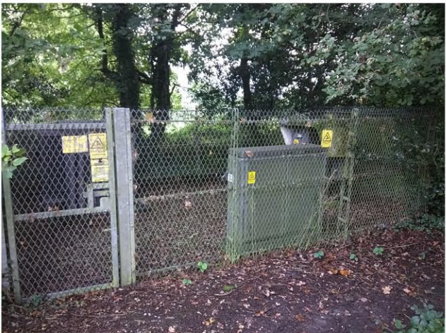
View 2 - Existing sub station located at southeast corner of proposed site
