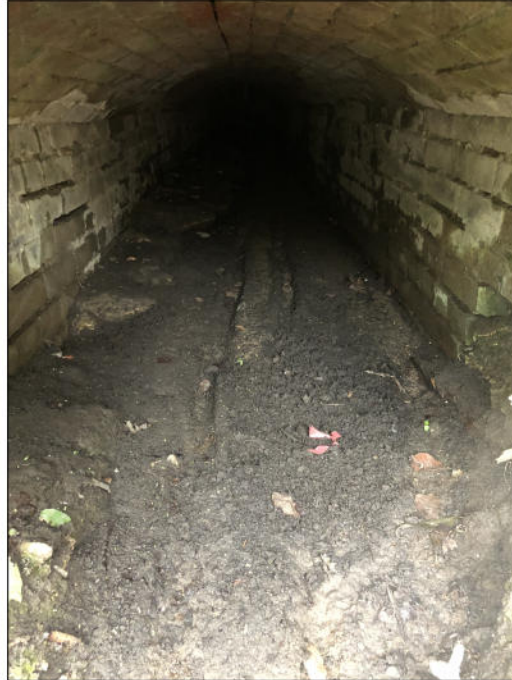
Photo: UPSTREAM FROM OUTFALL.1.JPG 0m, Start node type, outfall, reference number : OUTFALL.1
