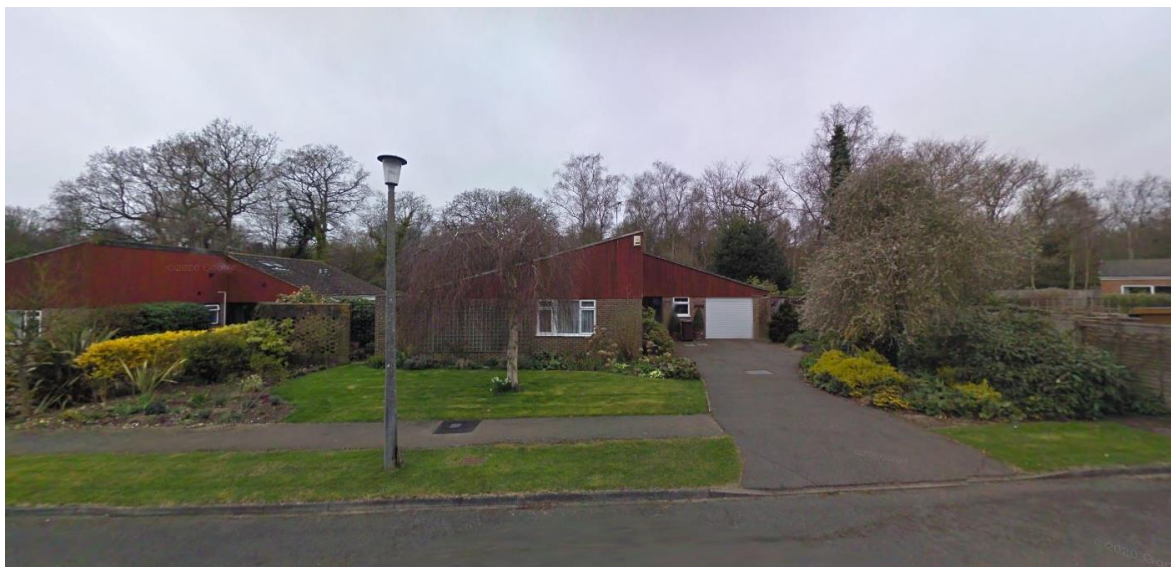
Figure 1: Front Elevation/ Street View of the Site at 7 Birch Close.
