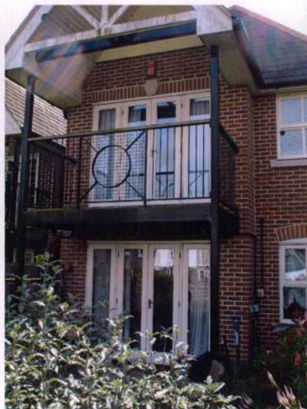
View of balcony area to be infilled
