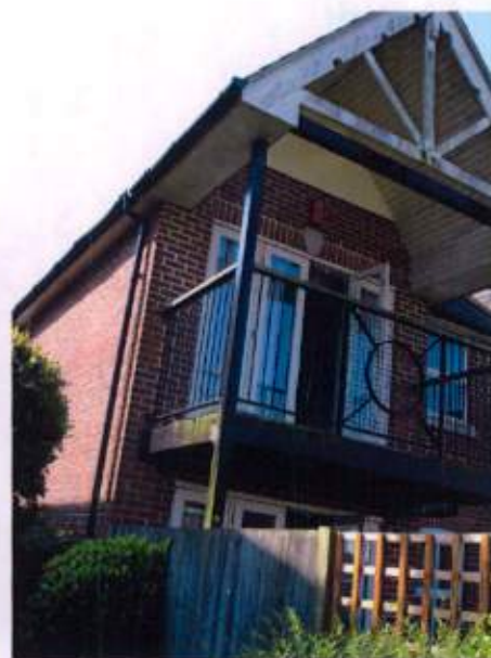
View of balcony structure
